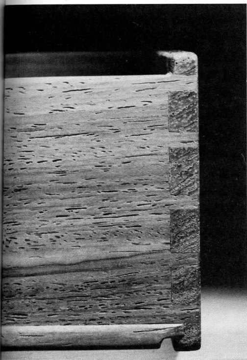
The back of a drawer. The solid wood bottom is shaped and grooved into sides and front piece. Doussie.
