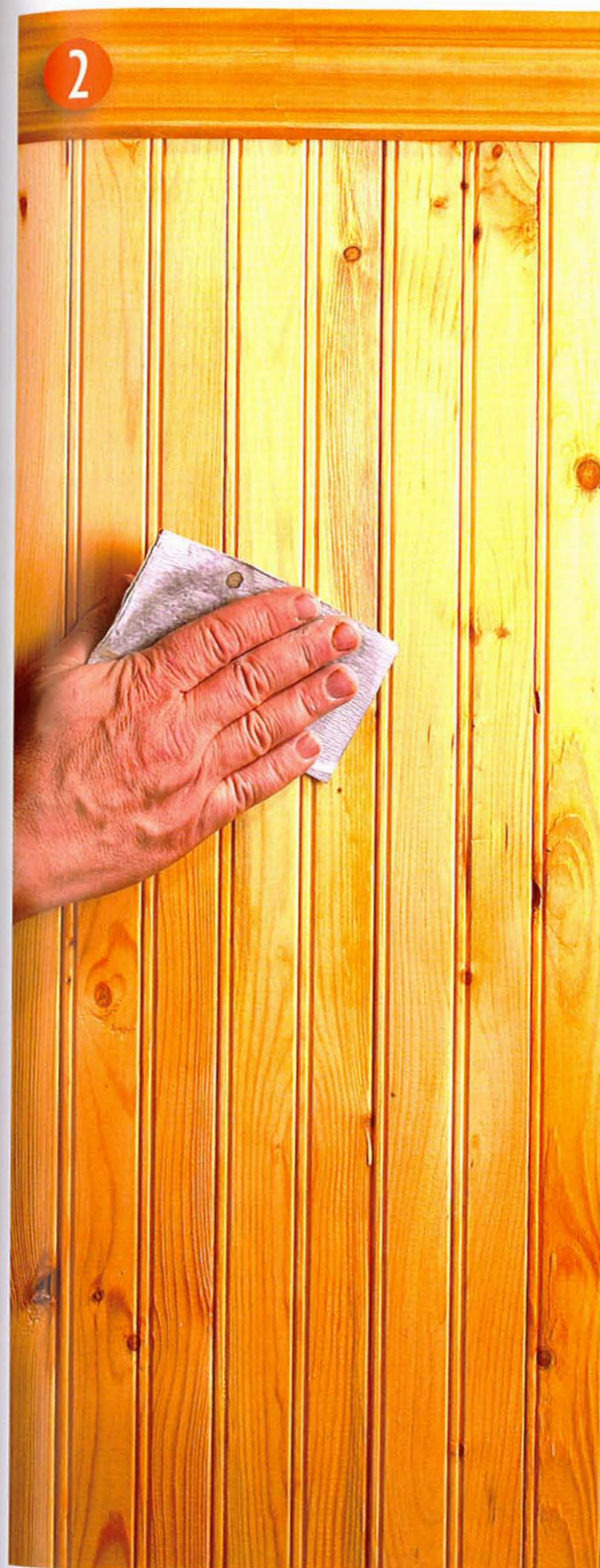
Once the shellac had dried I sanded with 320-grit silicon carbide sandpaper.
