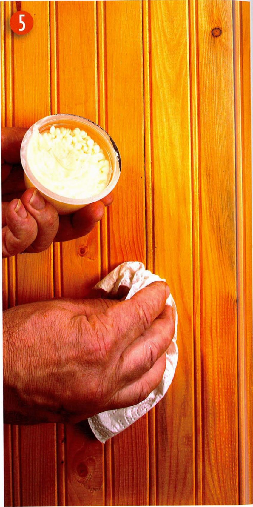
5 I then waxed the wood with a natural (beeswax) homemade wax and buffed it up. No sweat.
