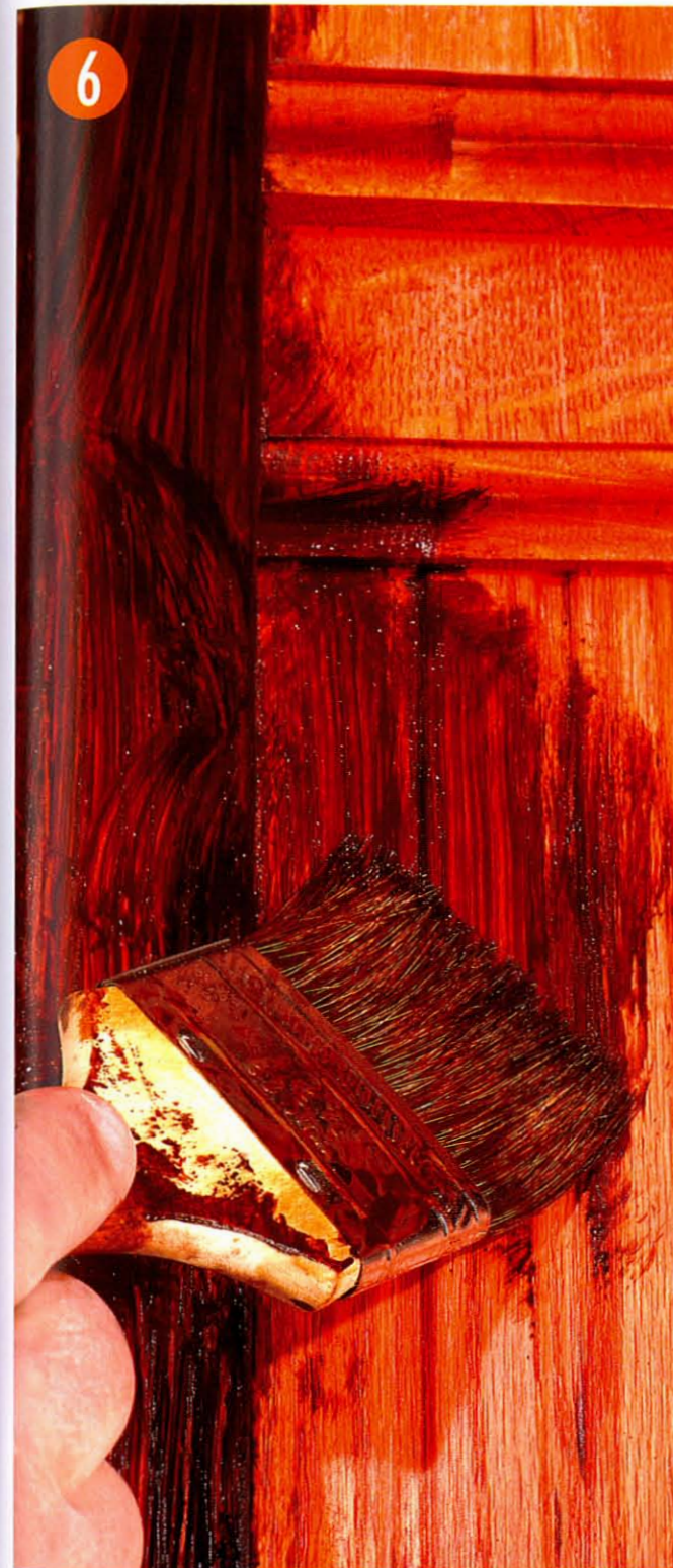
The top color was then applied. I used burnt umber artist's tube colors in place of the burnt umber Japan color. I thinned the tube color with mineral spirits the same way I did the orange color. Remember, because you have sealed the first coat of color with the shellac sealer, you can apply a coat of oil-based color without fear of the second color pulling off the first color.
