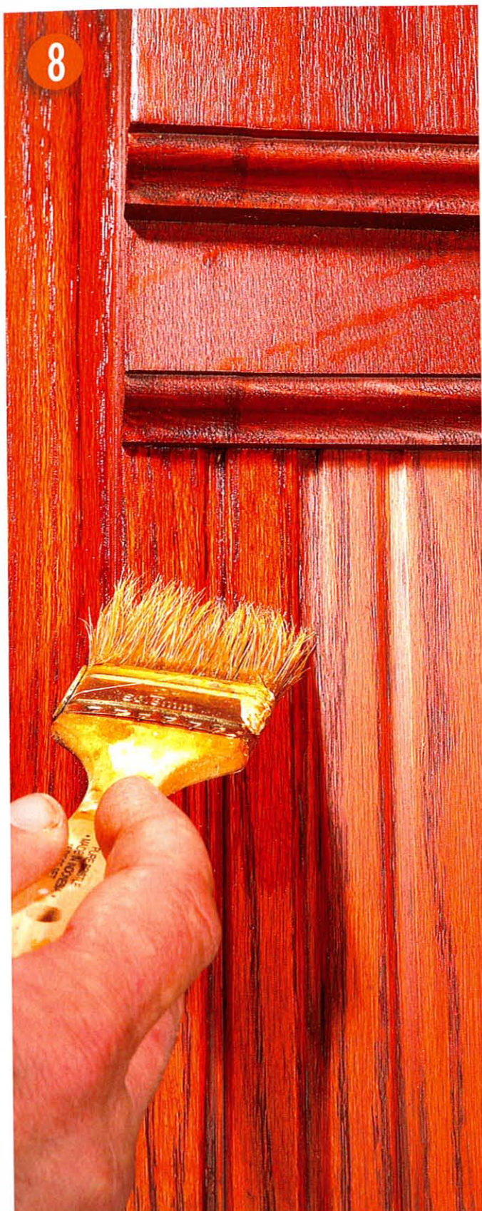
Next, I brushed on yet another sealer coat of orange shellac.
