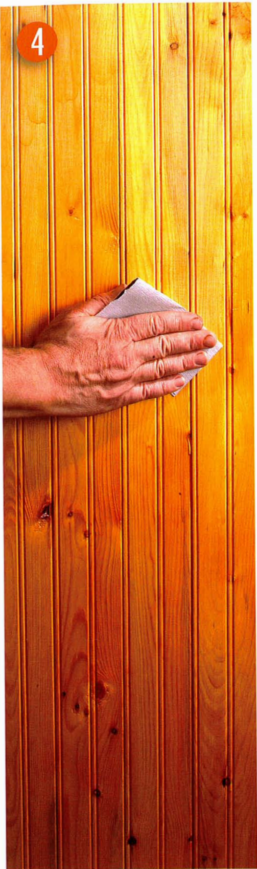
4 I sanded again when the shellac was dry and buffed the finish with No.0000 steel wool.
