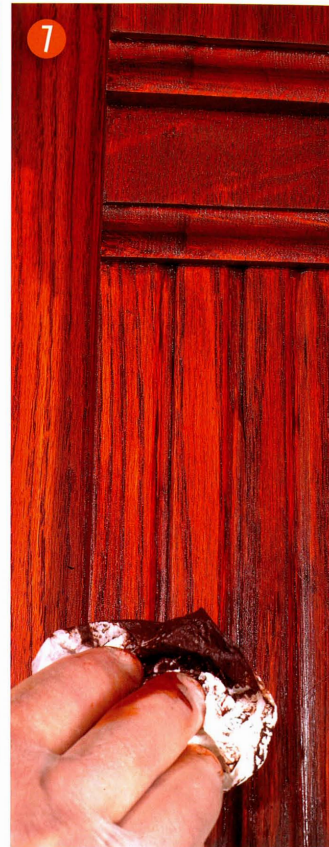
After removing the excess of burnt umber, the stain was allowed to dry.
