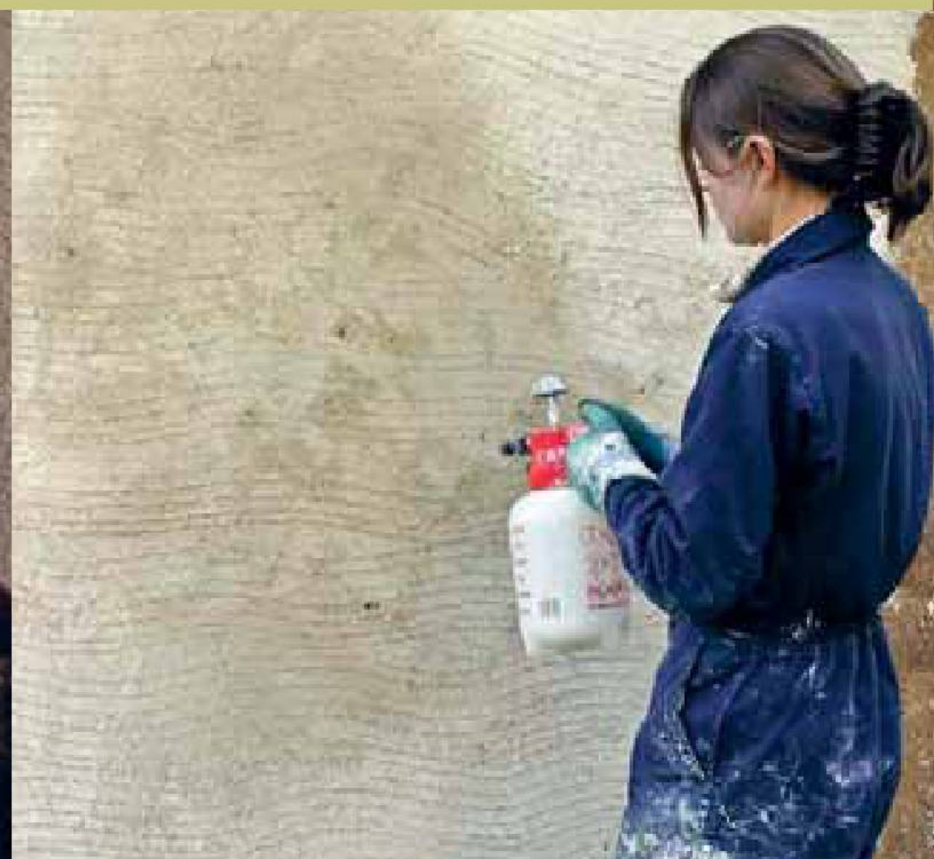
Left: Brushing the wall to remove dust and loose particles. Right: Misting the wall down to create adequate suction.
