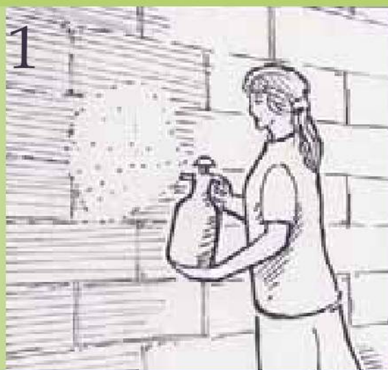
Thoroughly wet substrate to provide adequate suction.
