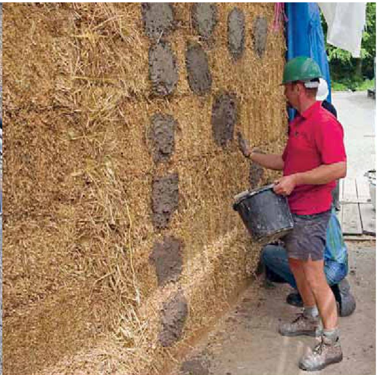
Left: A variety of sample earth plaster mixes with differing proportions of clay and aggregate. Right: The samples are applied to the wall to be plastered, allowed to dry, and then monitored for cracking, durability, adhesion and dusting.
