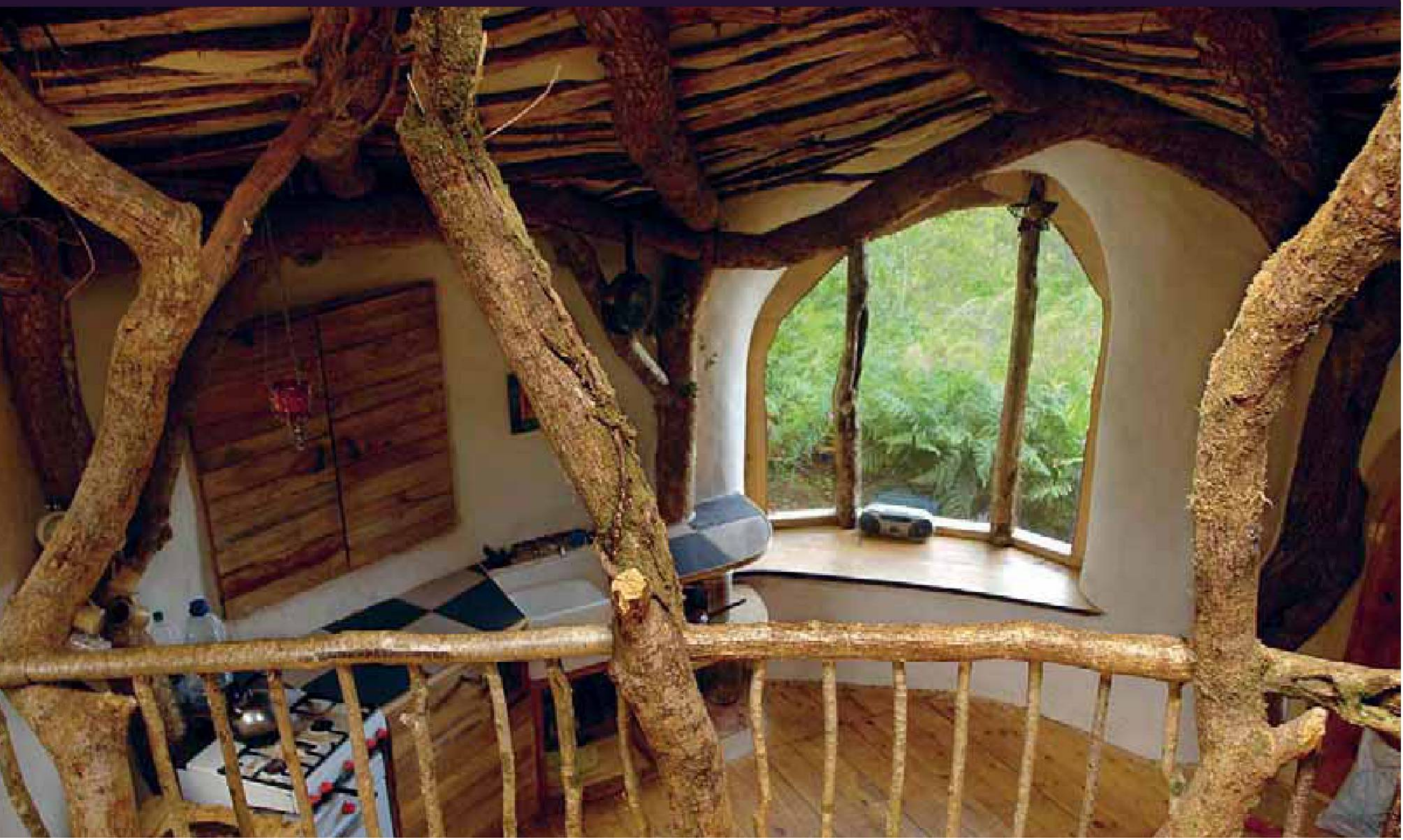
Lime finishes have been used to protect the walls of this straw bale home in Wales. Self-build by Simon Dale and family.
