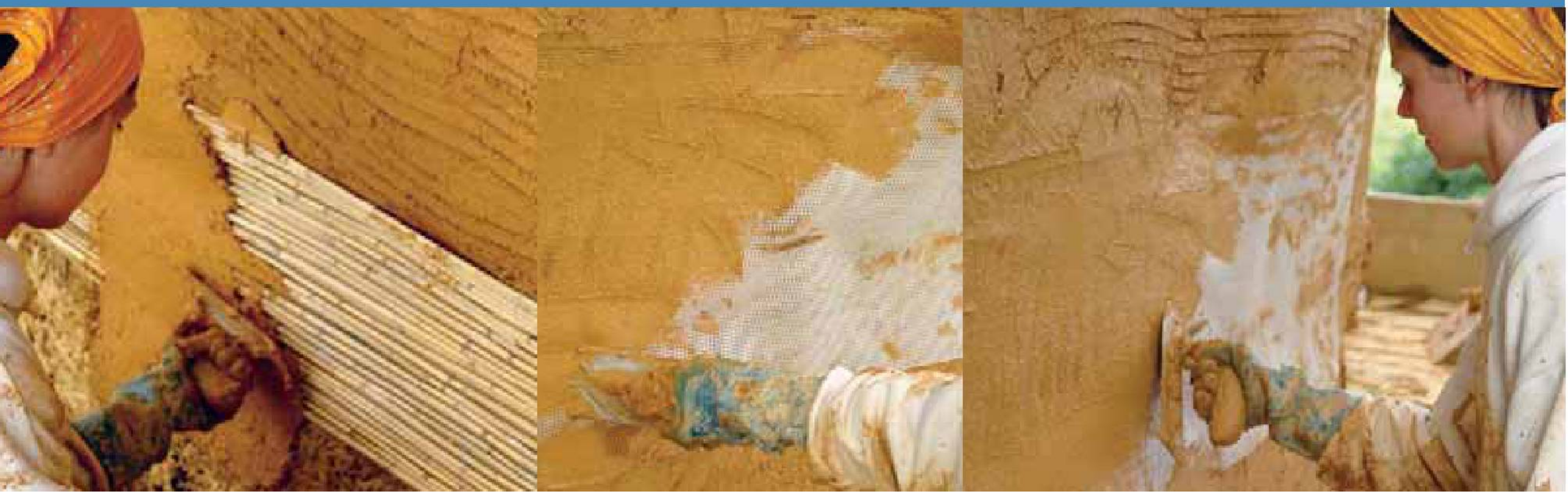
Below: Using reed mat to cover timber in the straw-bale wall. Glass-fibre mesh is embedded into the earth base coat to prevent cracking at the junction of reed mat and wall.
