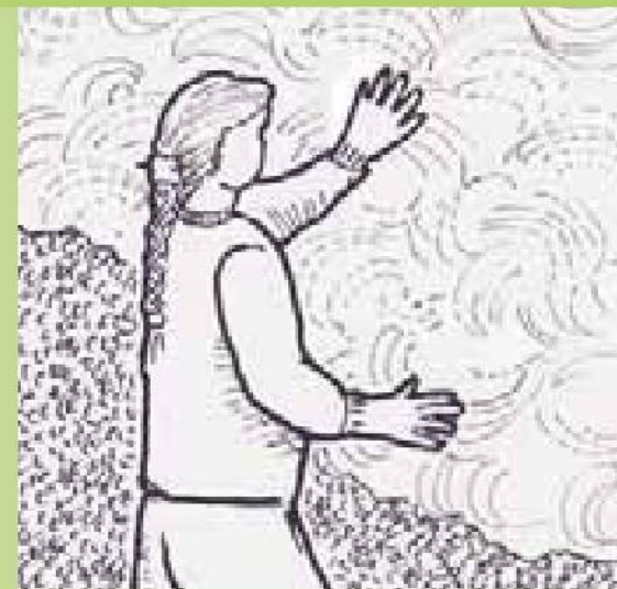
Work the mortar into the bales with the hands to coat the straw and fill holes and crevices.
