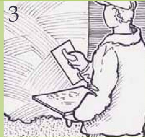
Mortar scooped onto trowel and pressed into wall into an upward arc.
