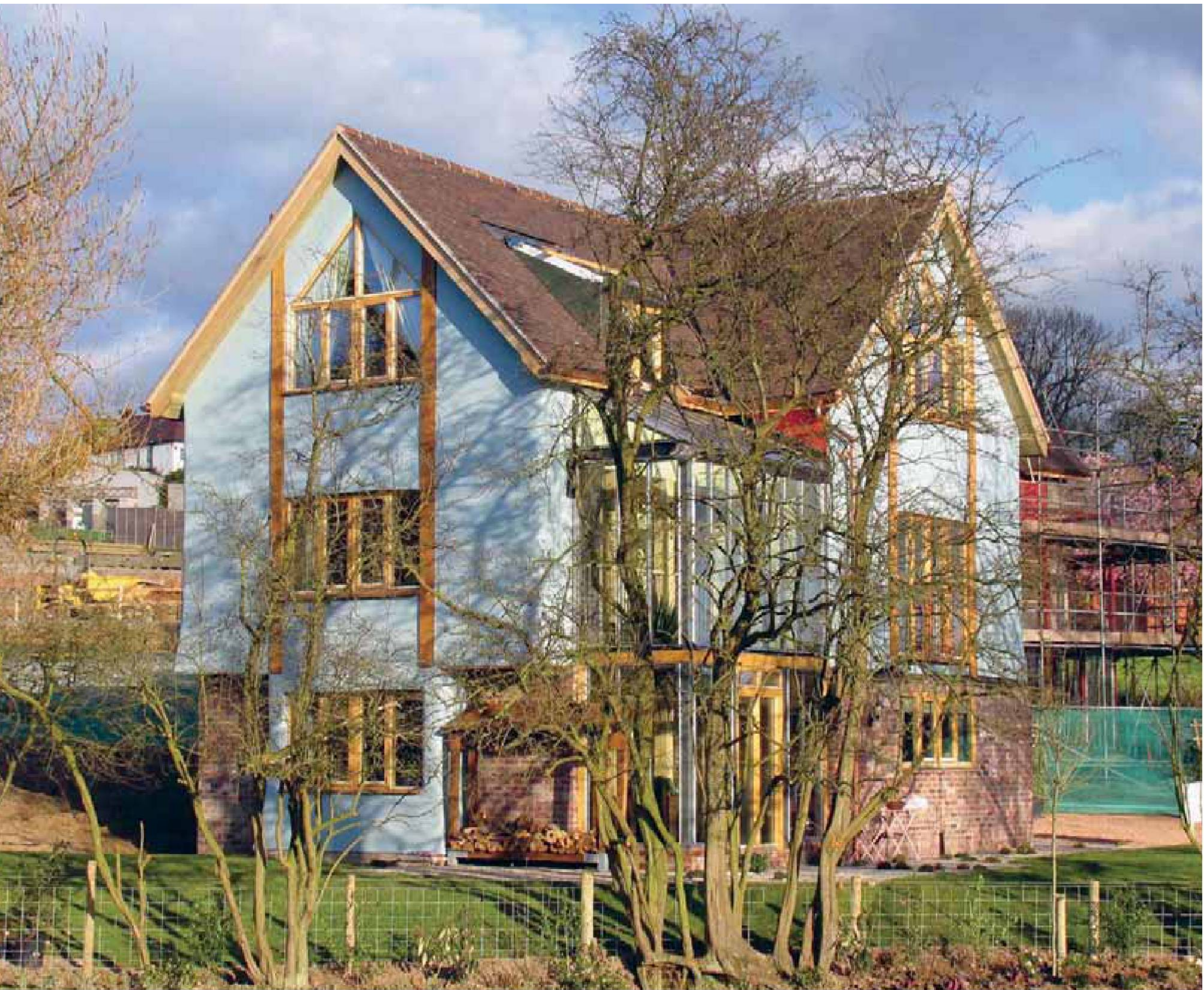
Above and below right: Lime finishes have been used to protect the external and internal walls of this eco-housing development in Shropshire. ( Living Villages, The Wintles ). Below left: A beautiful lime finish used in a kitchen in France. (By D'Ocres )
