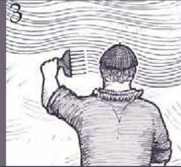
Scratch up damp plaster with a comb scratcher when still damp.
