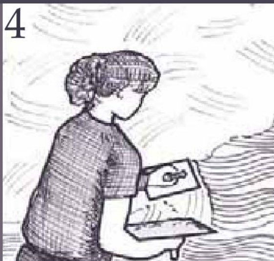
Apply the straightening coat onto the pre-dampened scratch coat.
