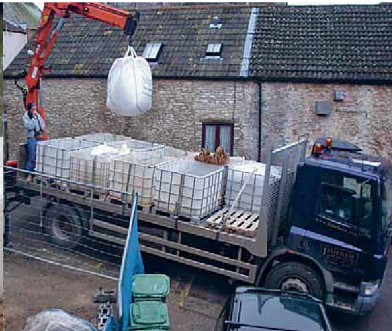
Left: Steaming non-hydraulic lime putty stored in 1-tonne sacks after it has been slaked. Right: 1-tonne ready-mixes being delivered to site.
