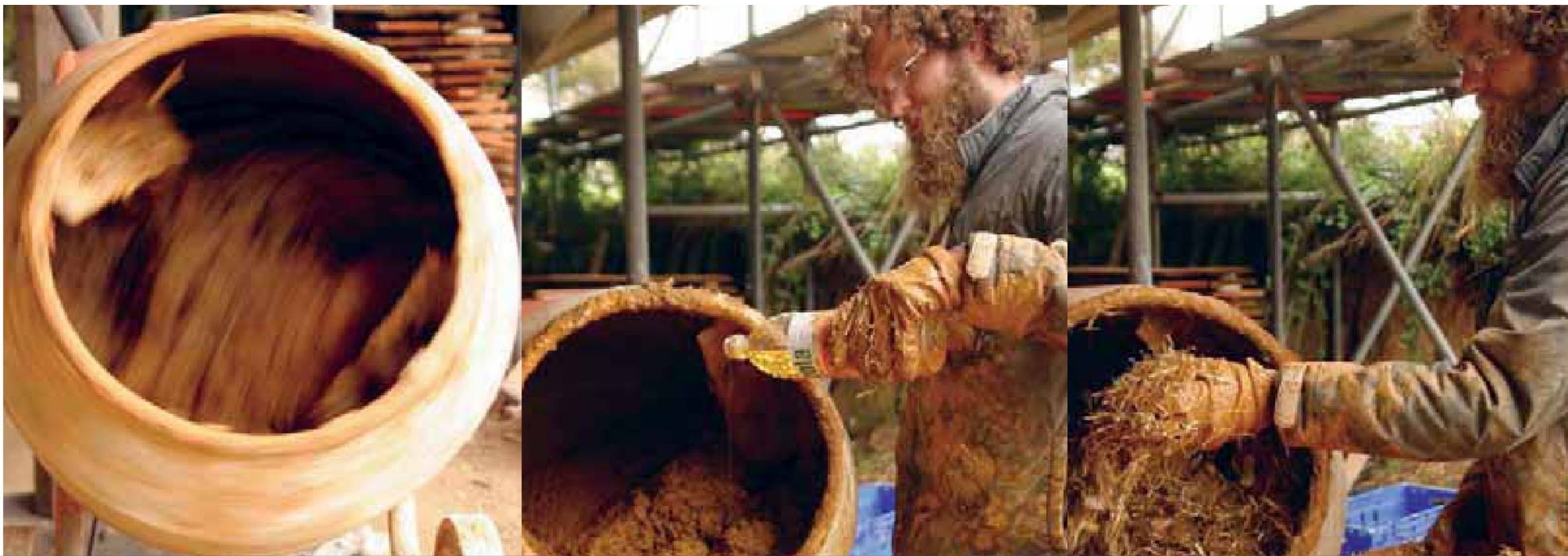
Left to right: Mixing the aggregate and clay slip together. Adding a small amount of vegetable oil to the mix. Adding the straw.
