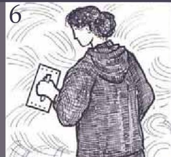
Scratch up the straightening coat with a devil float.
