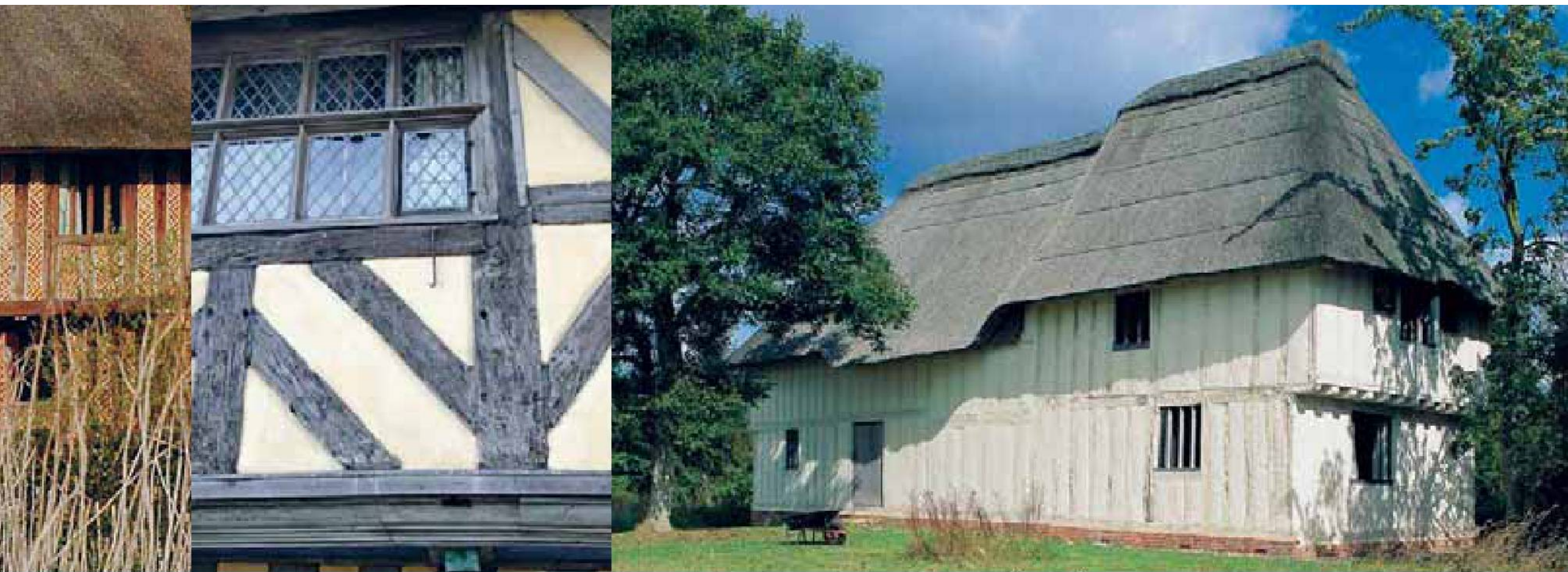
Flat-trowelled lime renders applied onto traditional timber-frame structures.
