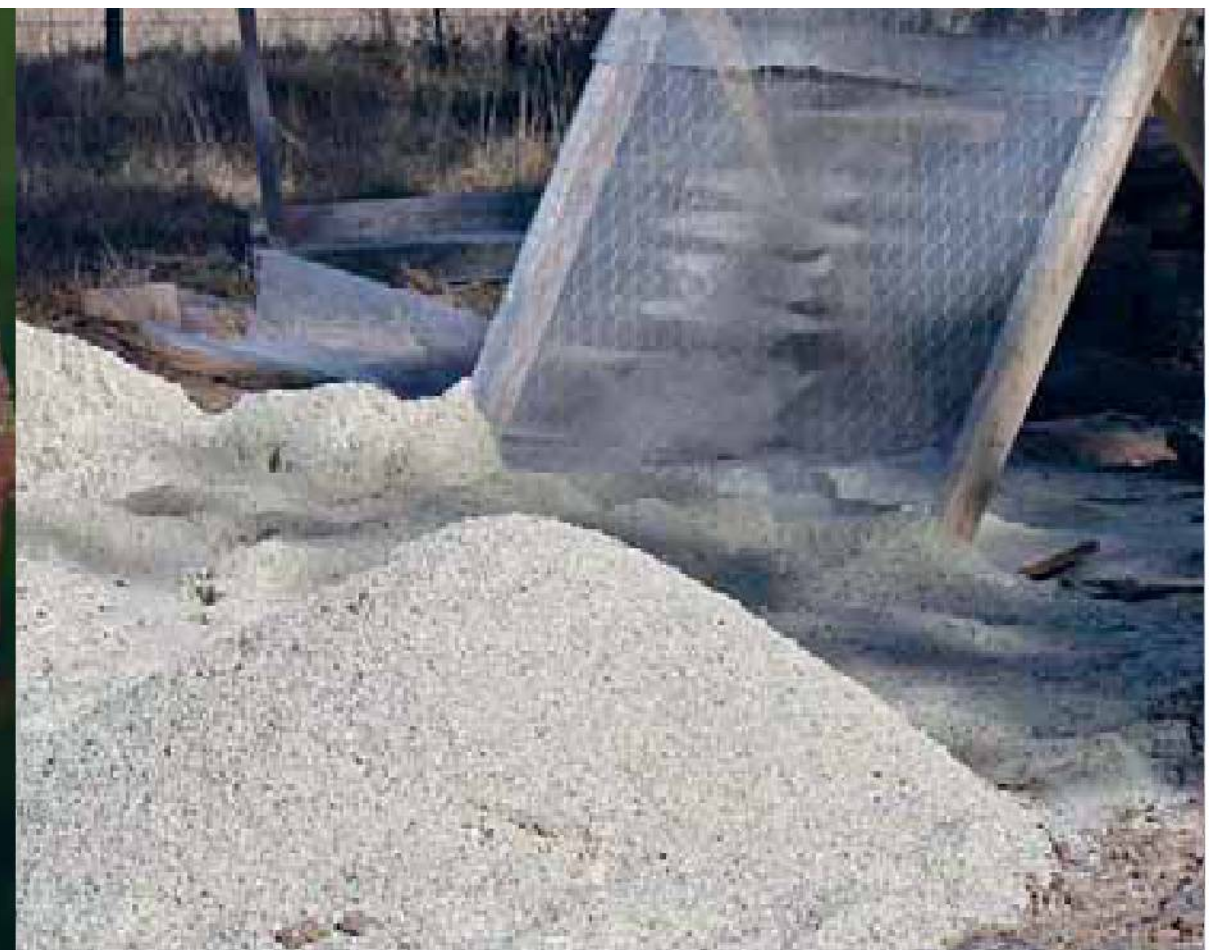
Left: Well-graded fine aggregate for internal finishing coats (left hand), and well-graded coarse aggregate for base coats and external finishing coats (right hand). Right: Home-sieving aggregate to create a well-graded mix.
