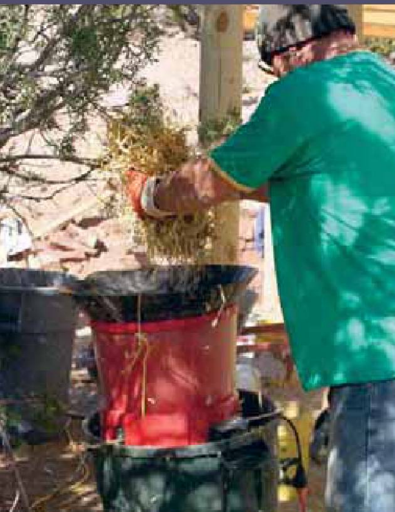
Above left: Sieving straw for the finishing coat. Above right: The fine, sieved straw ready to be mixed into an internal finishing coat earth plaster. Below left: Processing long fibres of straw through a leaf mulcher to chop it to the desired length. Below right: Adding the processed straw to the earth plaster mix.
