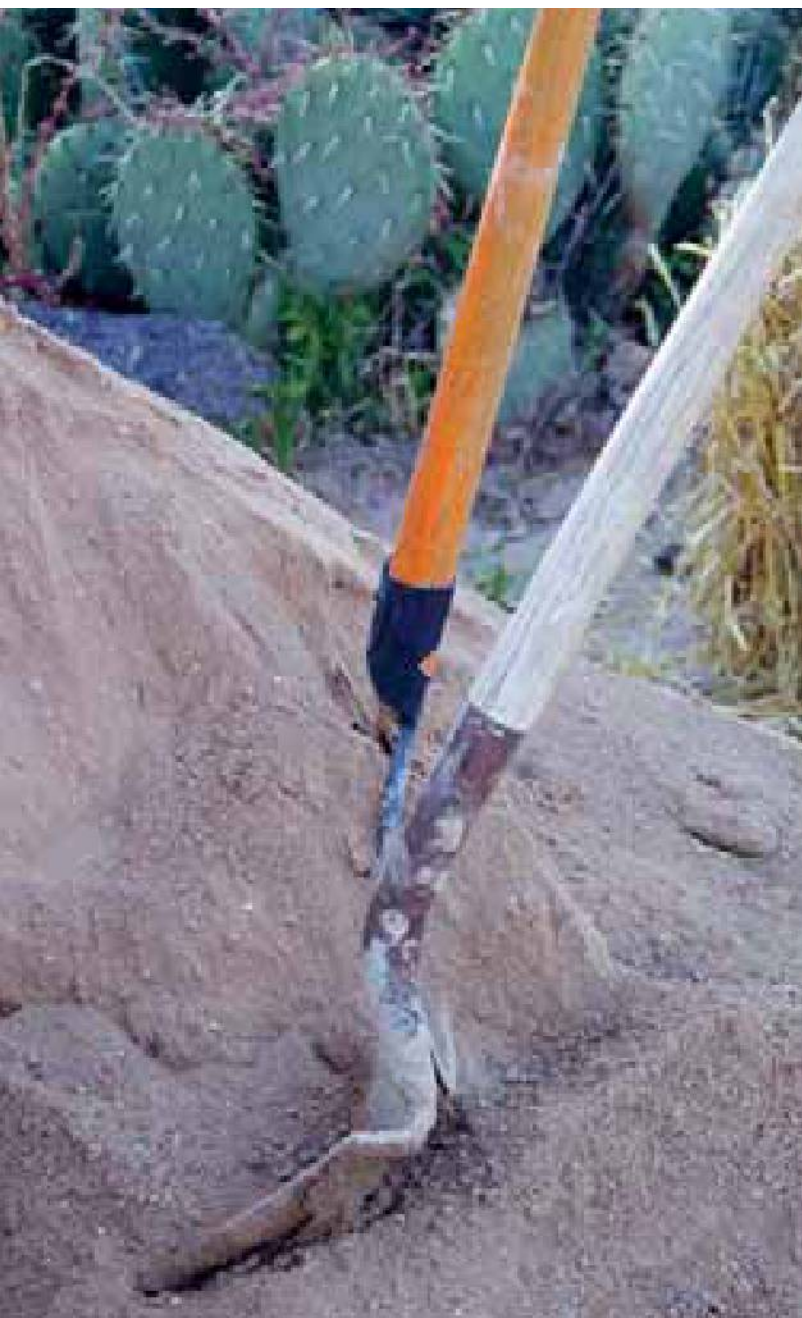
Above left: Dry clay and aggregate mix for an earth plaster. Above right: Sieving dry clay through a sieve set up at a 45 degree angle. Middle left: Straw can be used in earth plasters to provide tensile strength. It must be chopped into short lengths for ease of application. Bottom left: Kaolin clay can be used to make earth plasters. Below: A pre-manufactured earth plaster. It simply needs the addition of water.
