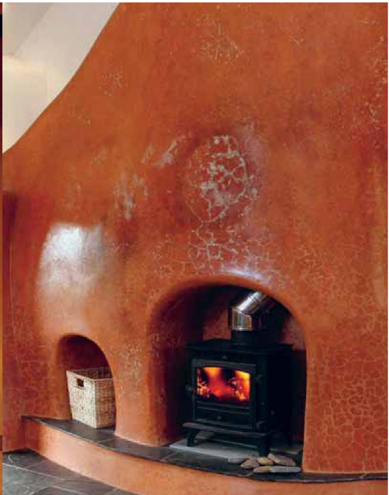
Left: Linseed oil has been used as a stain on an earth plaster to create this beautiful trim detail at the Tower Gallery, New Mexico, USA. Right: A polished beeswax finish on top of an earth plaster to create a rich, sheeny lustre. Designed by Alison Bunning.
