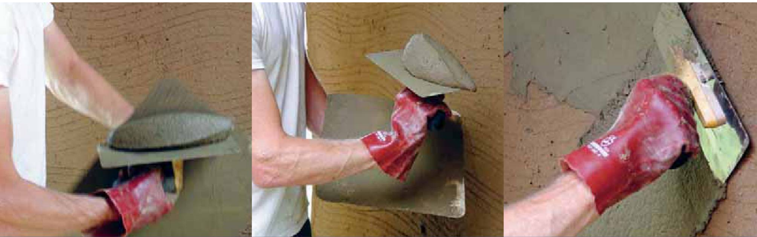
Above left to right: Scooping the worked plaster onto the trowel and spreading it onto the wall with a firm upward stroke.
