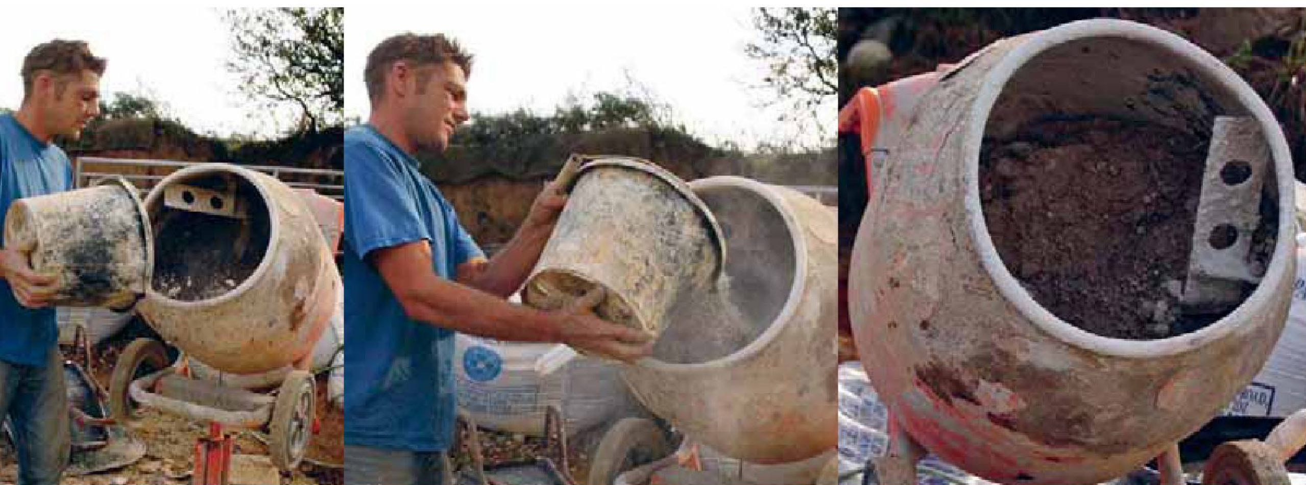
Making up a natural hydraulic lime-aggregate render in a drum mixer. Note: Please wear protective goggles, gloves and dust mask! Left to right: Adding aggregate; Adding hydraulic lime powder; Aggregate and lime mixing together.
