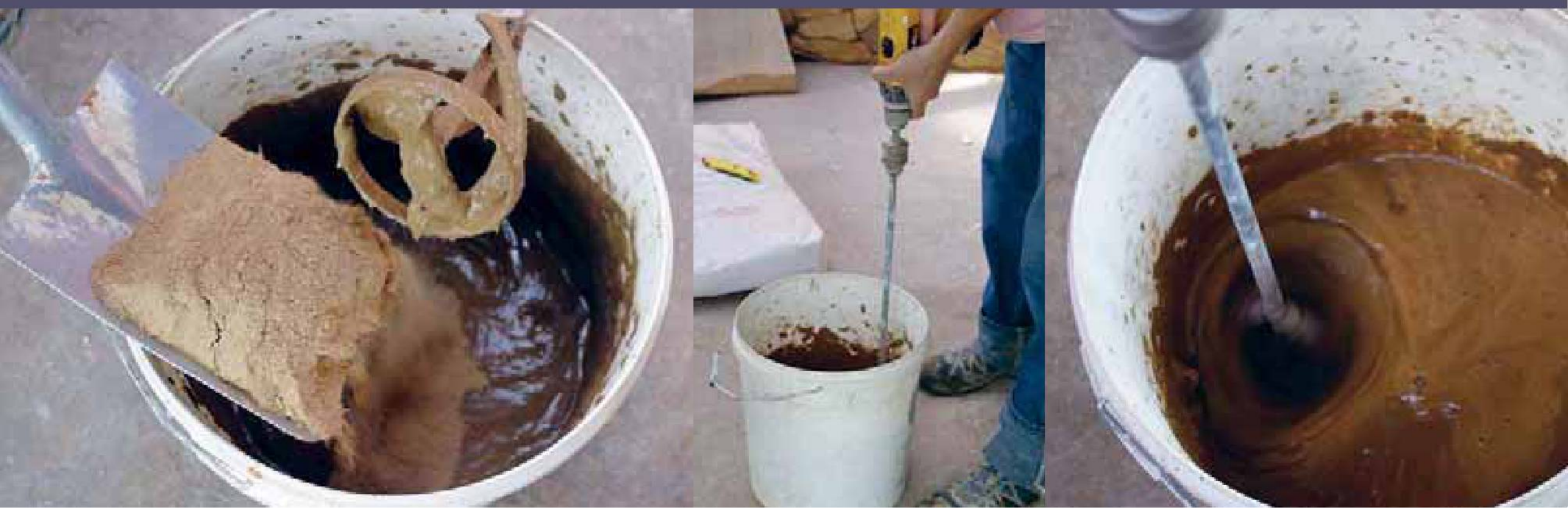
Mixing a pre-manufactured earth plaster in a bucket.
