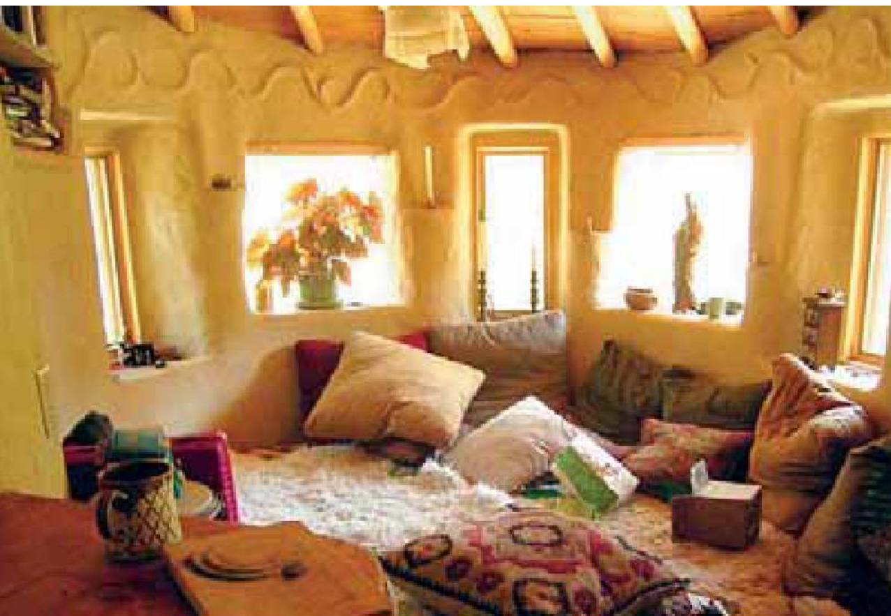
Left: New cob house with internal lime finishes and relief work. Right: Pigmented lime render in Saint-Antonin-Noble-Val, France.
