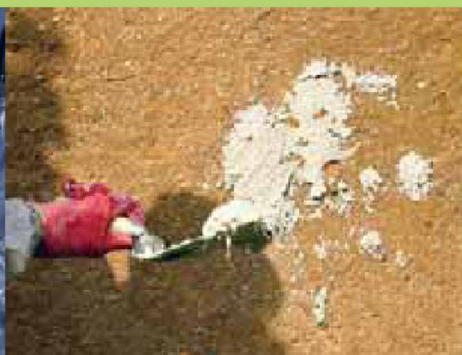
Stand at right angle and forcefully flick the mortar onto the wall evenly.
