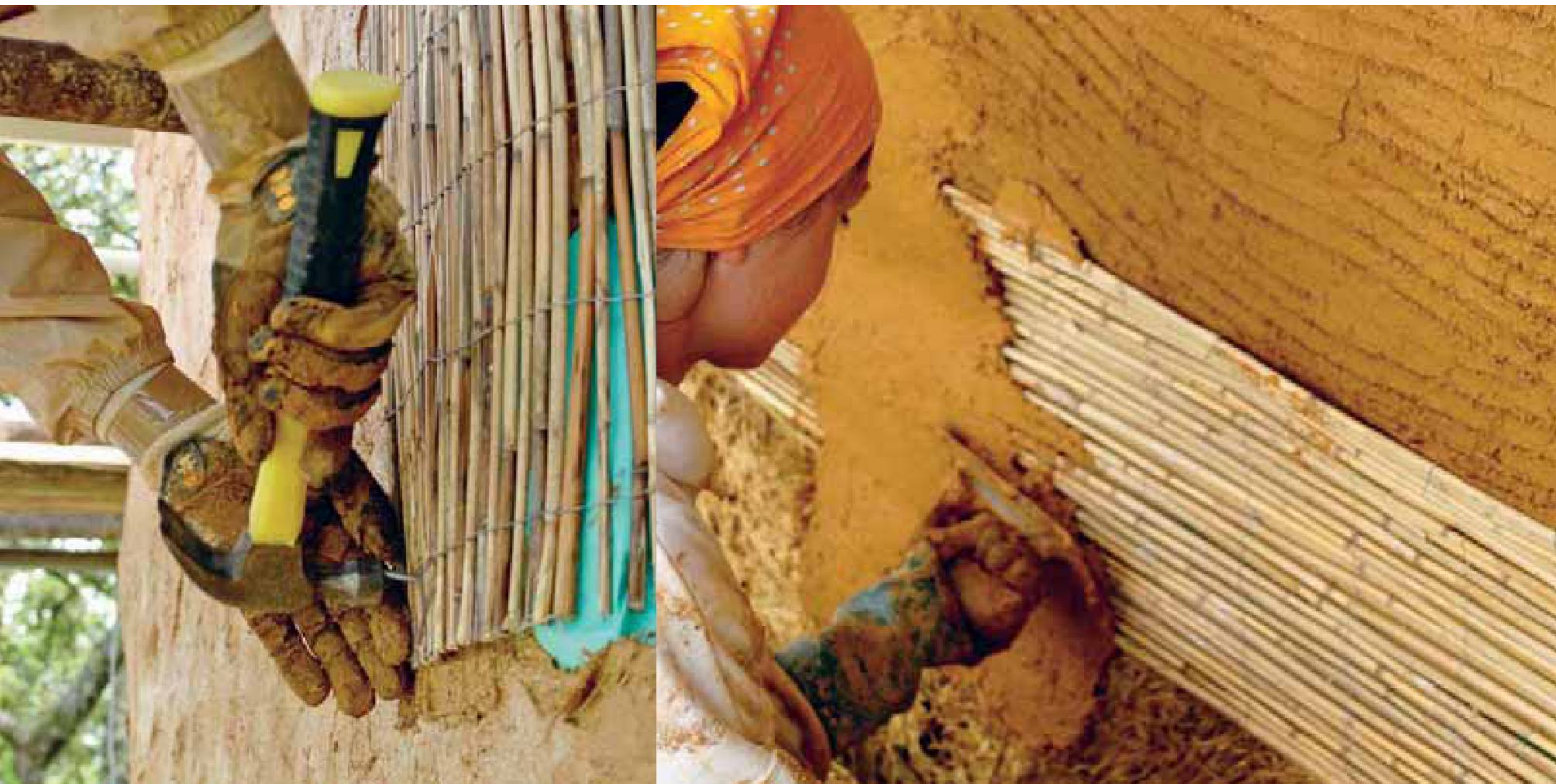
Left: Spiking reed mat into the bales using u-nails. Right: The reed mat has been used to cover timber in a straw-bale wall. An earth plaster is being squeezed through the gaps to key it into the wall beneath.
