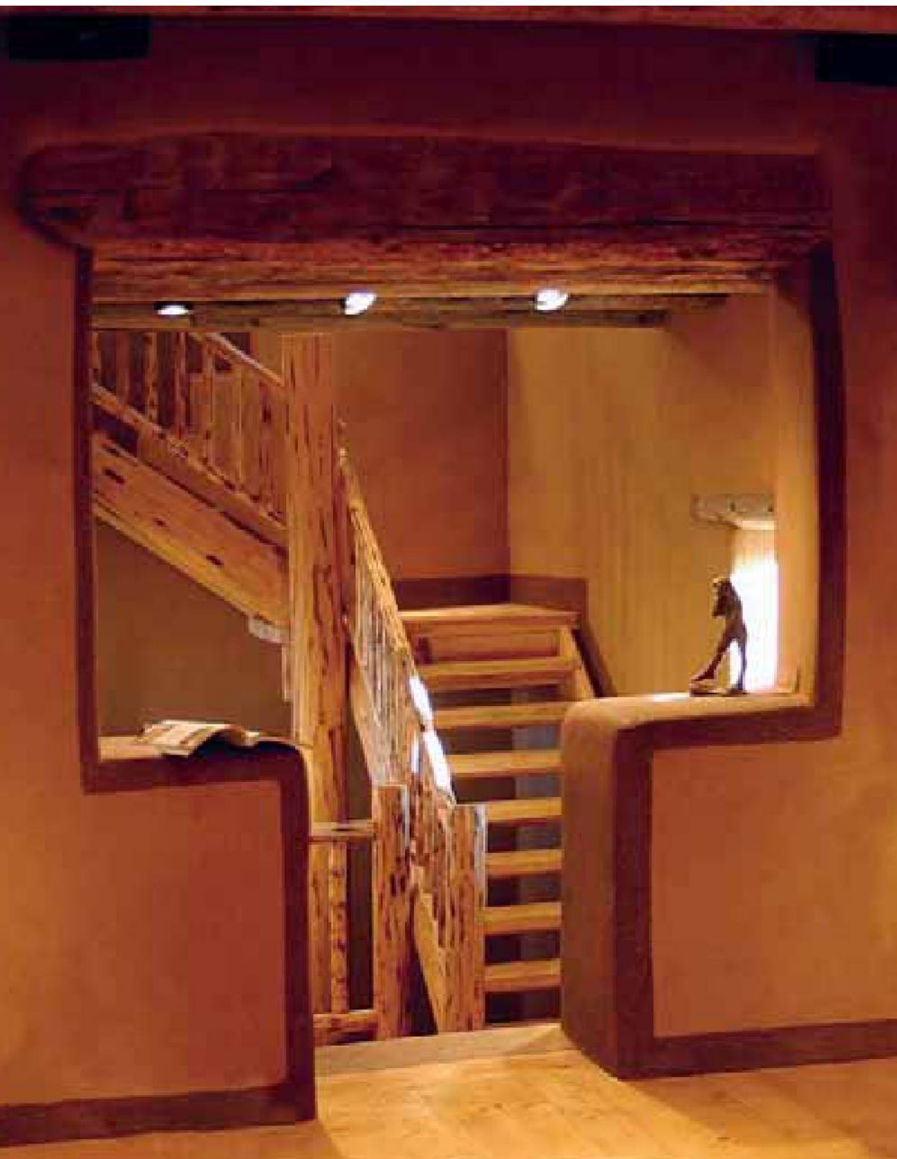
Left: Linseed oil has been used as a stain on an earth plaster to create this beautiful trim detail at the Tower Gallery, New Mexico, USA. Right: A polished beeswax finish on top of an earth plaster to create a rich, sheeny lustre. Designed by Alison Bunning.
