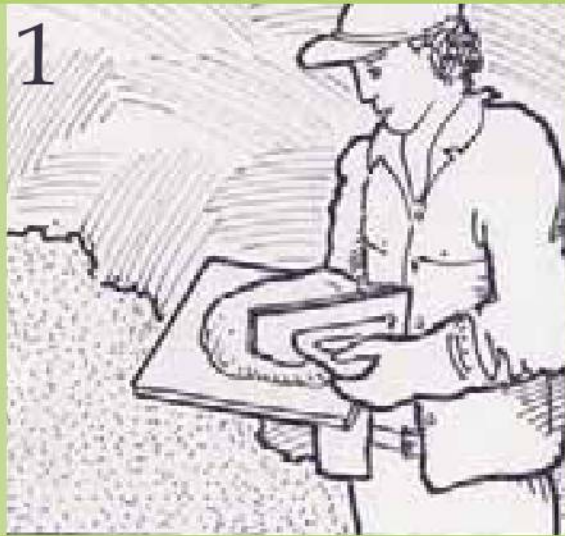
Working mortar on hawk standing square onto the wall.
