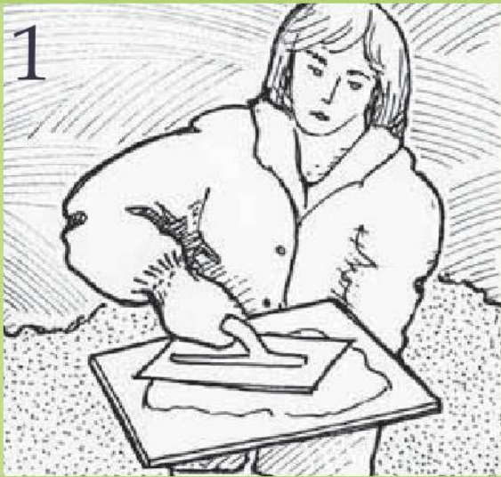
1 Worked mortar on hawk. Scoop up mortar onto trowel.
