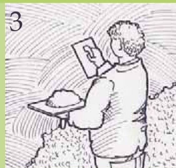
Apply further troweled or harled coat(s) as needed. Harled material can be pressed back or left rough.
