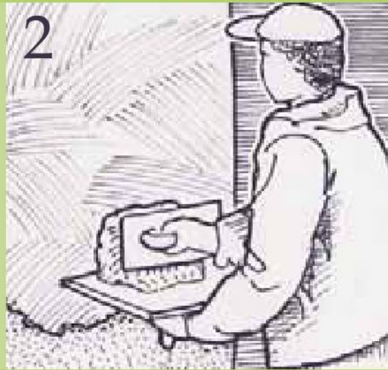
Hold hawk up against the wall and push mortar onto wall.
