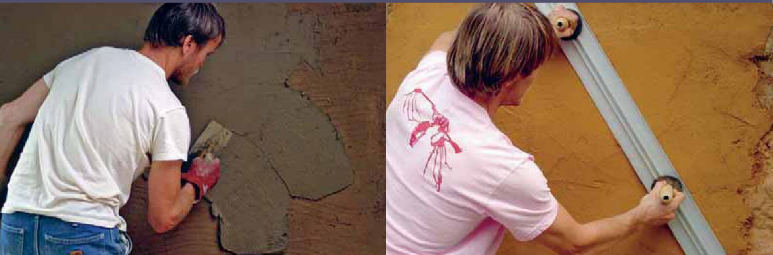
Above left: Applying an earth plaster straightening coat with a laying on trowel. Above right: Using a darby to straighten the earth plaster. Below left: Applying a kaolin clay plaster finishing coat. Below right: Sponging the kaolin plaster finishing coat.
