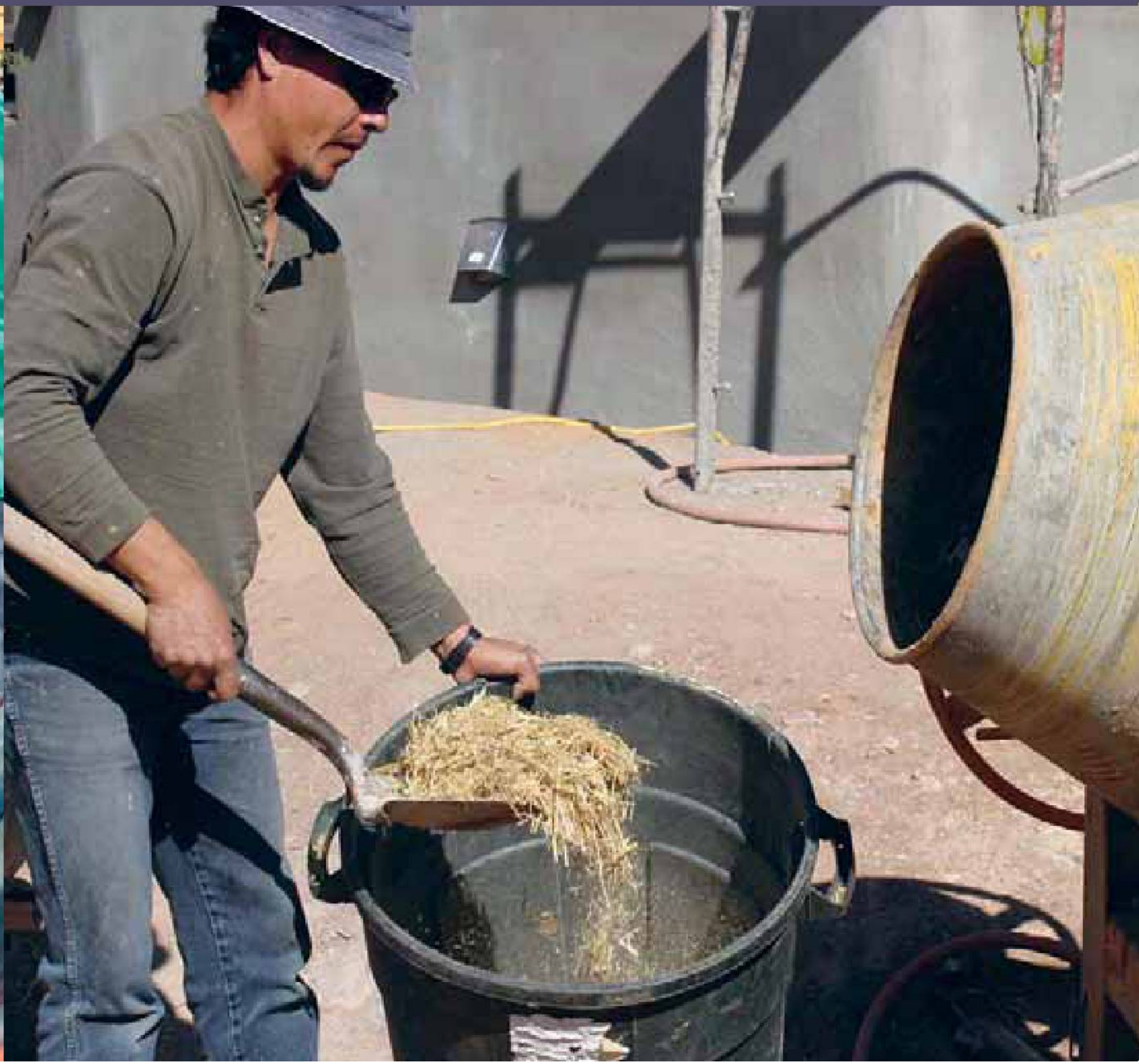
Above left: Sieving straw for the finishing coat. Above right: The fine, sieved straw ready to be mixed into an internal finishing coat earth plaster. Below left: Processing long fibres of straw through a leaf mulcher to chop it to the desired length. Below right: Adding the processed straw to the earth plaster mix.
