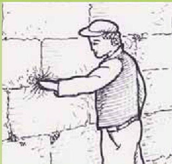
Stuff the crevices between the straw bales with straw coated in clay slip.
