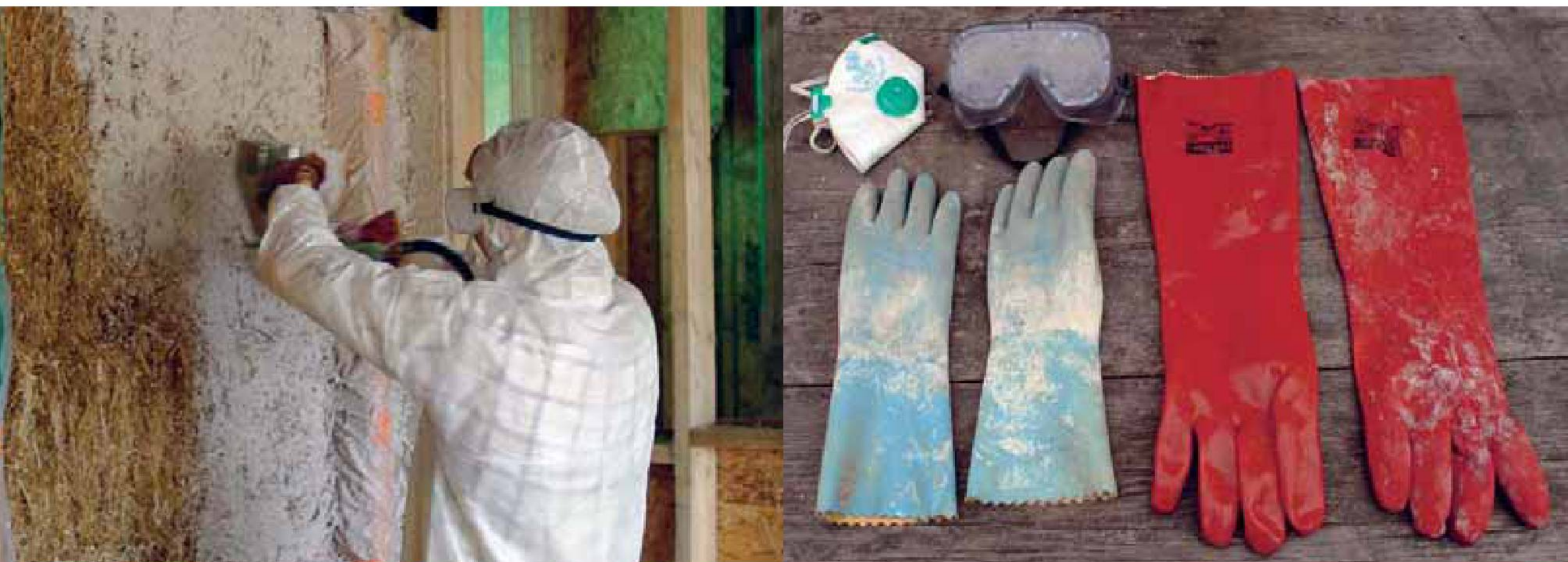
Left: Protective gear worn to protect against the lime. Right: It is essential that suitable gear is worn when working with lime to protect the skin, eyes and lungs (when mixing natural hydraulic lime powder).
