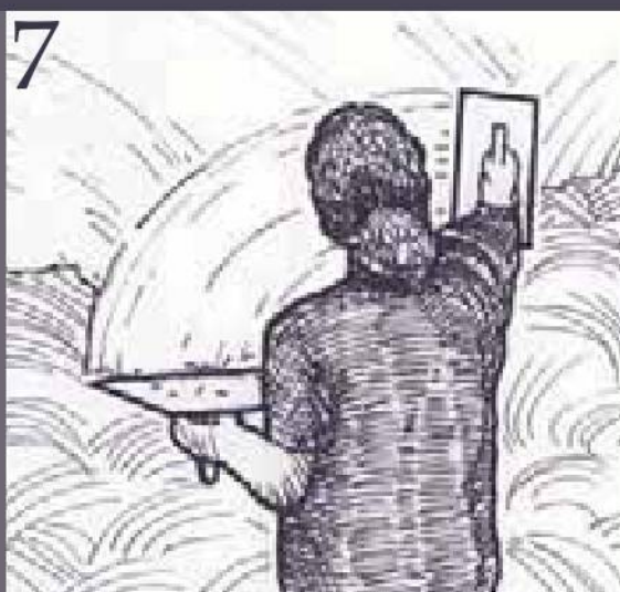
Apply the final coat onto the pre-dampened straightening coat.
