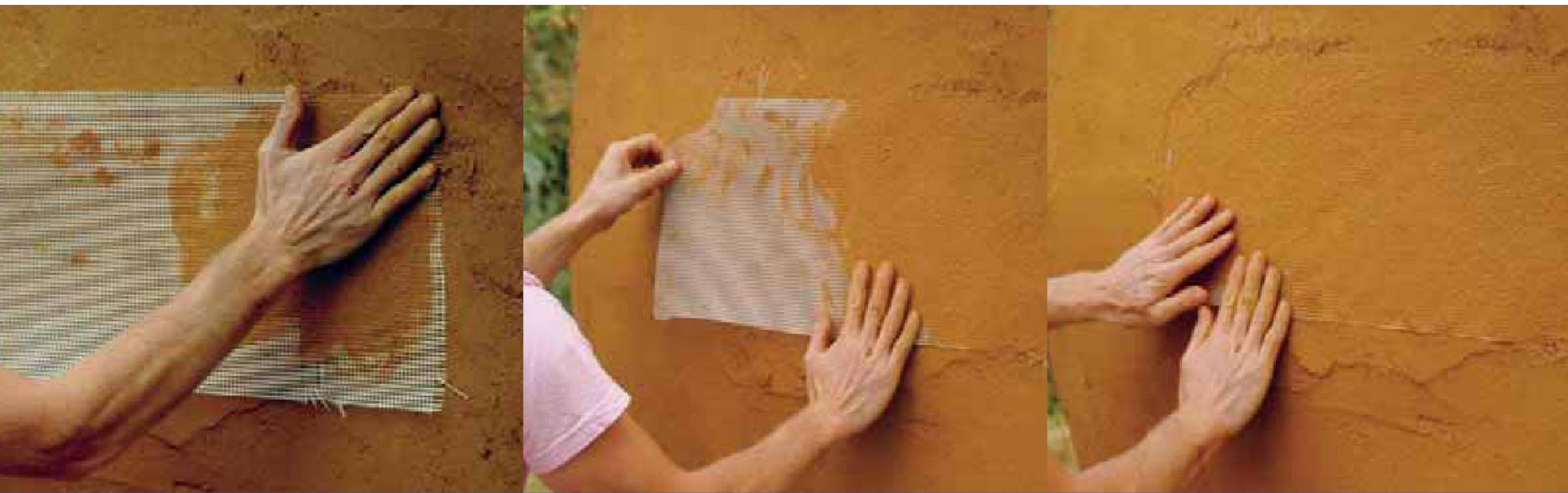
Glass-fibre mesh being incorporated into an earth plaster base coat to cover a localised repair in the wall. Once worked in with the hands, it should be well compressed into the plaster with a trowel.
