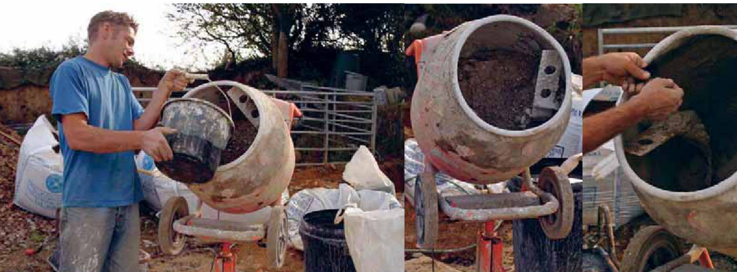
Adding water gradually and in small increments; Lime, aggregate and water mixing together (approximately 20 minutes); Teasing in hair; Mix until the hair is fully incorporated.
