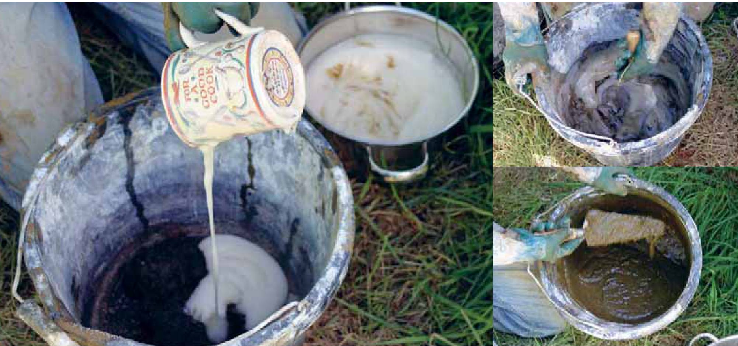
Making a sanded adhesion coat with wheat flour paste, manure and coarse aggregate.
