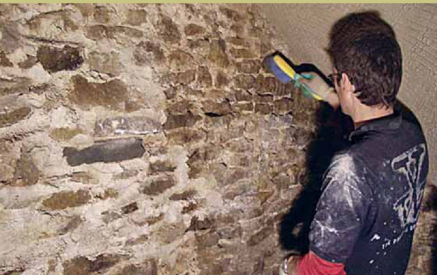
Left: Brushing the wall to remove dust and loose particles. Right: Misting the wall down to create adequate suction.
