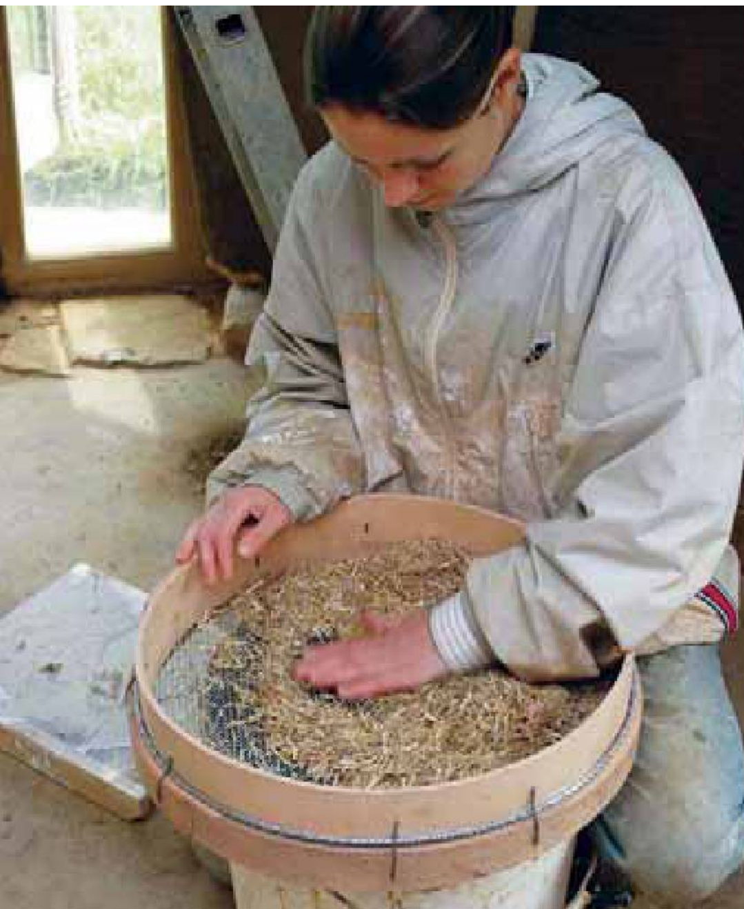
Above left: Sieving straw for the finishing coat. Above right: The fine, sieved straw ready to be mixed into an internal finishing coat earth plaster. Below left: Processing long fibres of straw through a leaf mulcher to chop it to the desired length. Below right: Adding the processed straw to the earth plaster mix.
