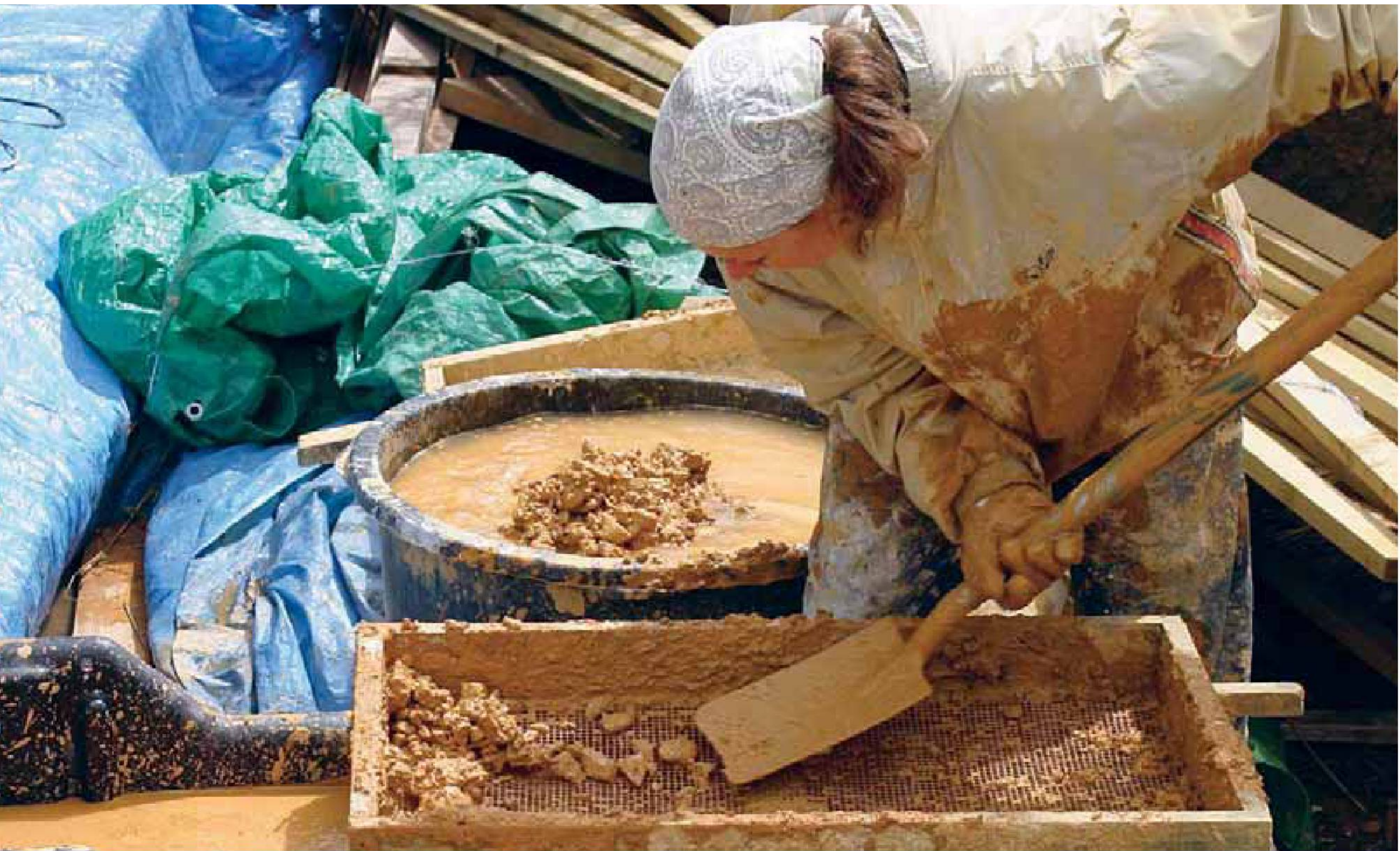
Wet-sieving a pre-soaked clay subsoil.
