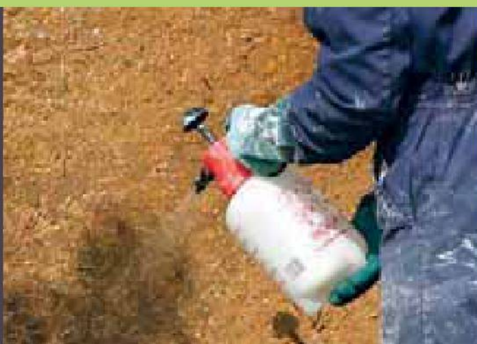
Thoroughly wet substrate to provide adequate suction.
