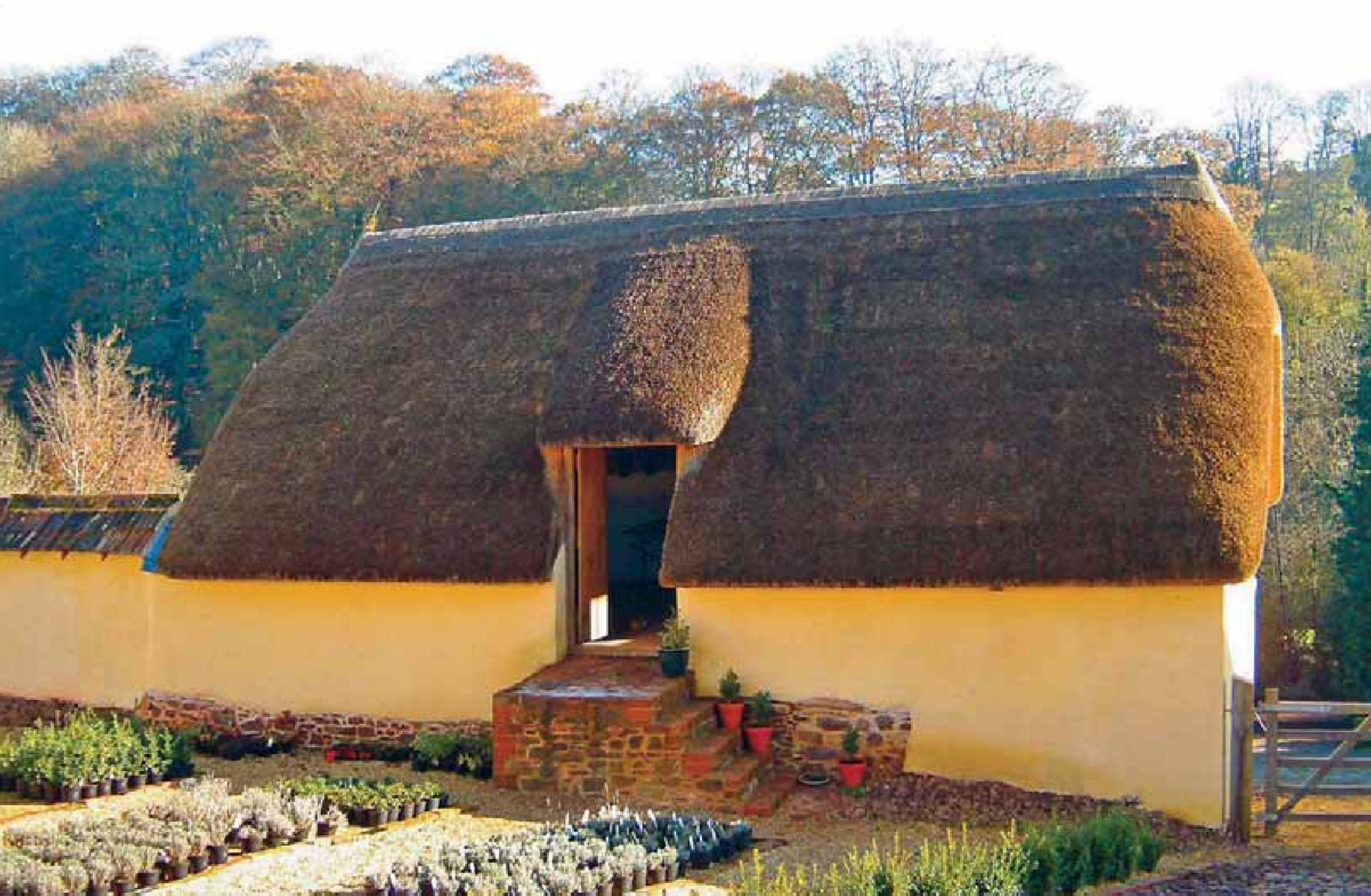
Before and after restoration of old cob barn, with lime render and pigmented limewash. The lime render will allow the cob to breathe, ensuring that the structure will remain healthy well into the future. Finishes by Mike Wye & Co.
