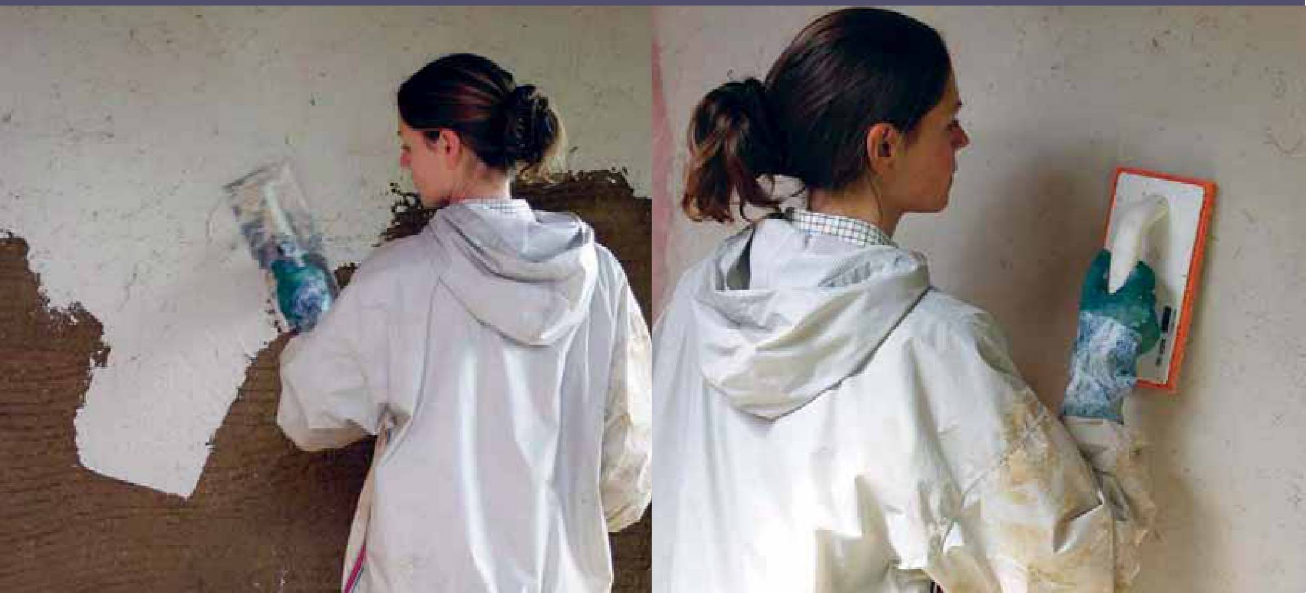
Above left: Applying an earth plaster straightening coat with a laying on trowel. Above right: Using a darby to straighten the earth plaster. Below left: Applying a kaolin clay plaster finishing coat. Below right: Sponging the kaolin plaster finishing coat.
