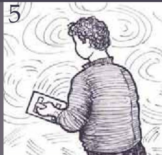
Scour the straightening coat using a wooden float once it has firmed up.
