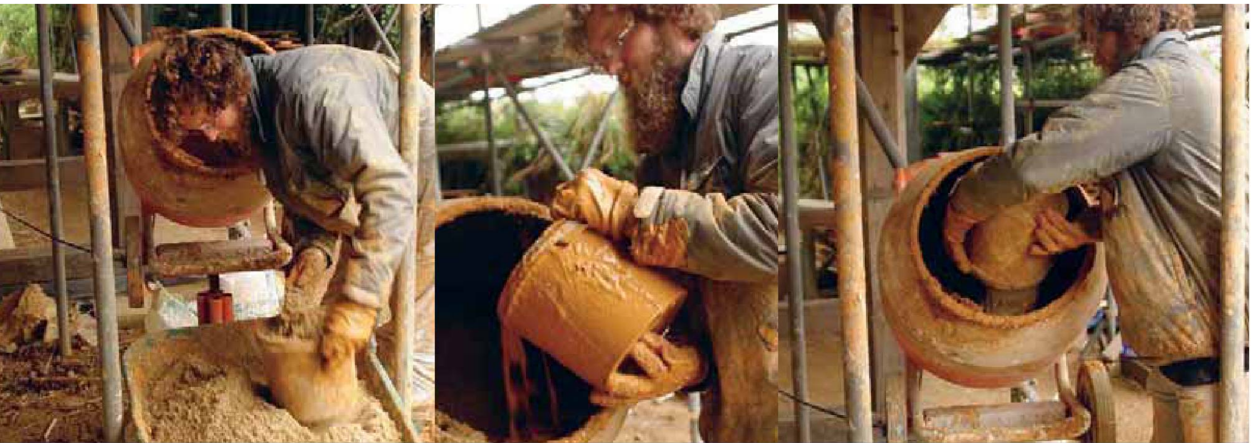
Left to right: Adding half of the aggregate to the mixer. Adding clay slip to the aggregate. Adding the rest of the aggregate.
