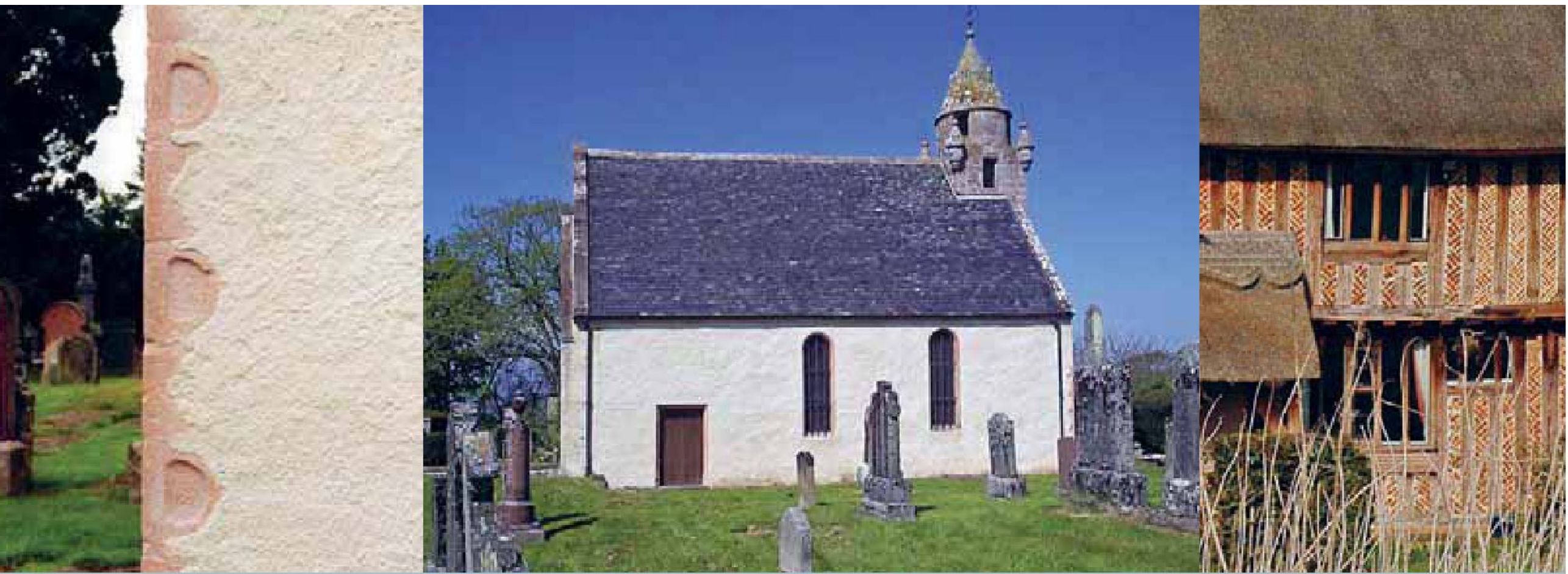
Left and middle: Traditional harled lime finishes in Scotland. Right: Herringbone brick infill laid in a lime mortar.
