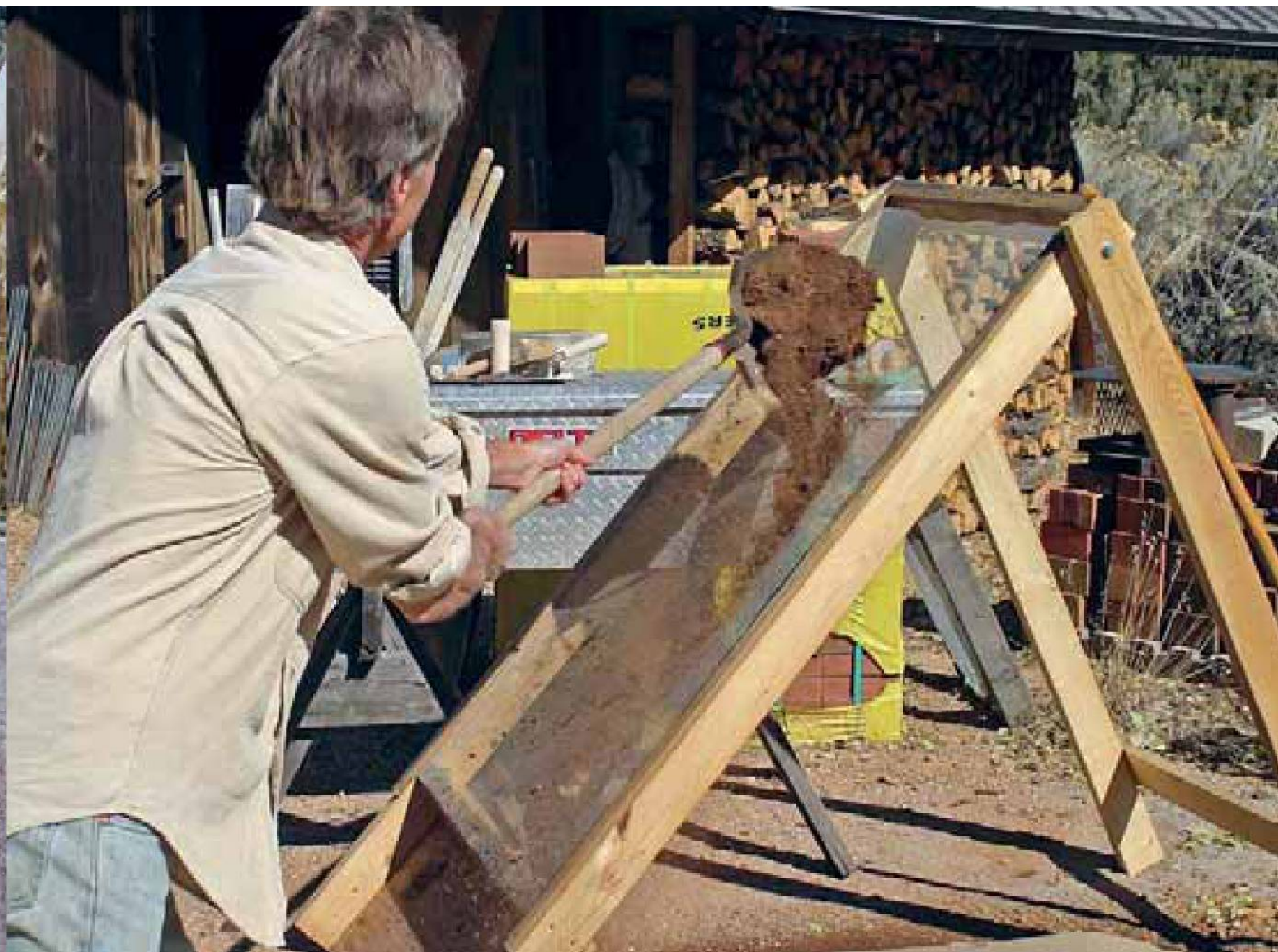
Above left: Dry clay and aggregate mix for an earth plaster. Above right: Sieving dry clay through a sieve set up at a 45 degree angle. Middle left: Straw can be used in earth plasters to provide tensile strength. It must be chopped into short lengths for ease of application. Bottom left: Kaolin clay can be used to make earth plasters. Below: A pre-manufactured earth plaster. It simply needs the addition of water.
