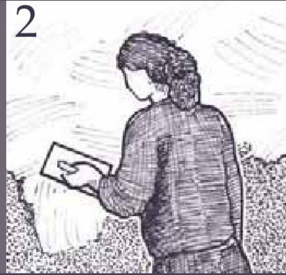
Apply scratch coat using a steel laying on trowel or tool of your choice.
