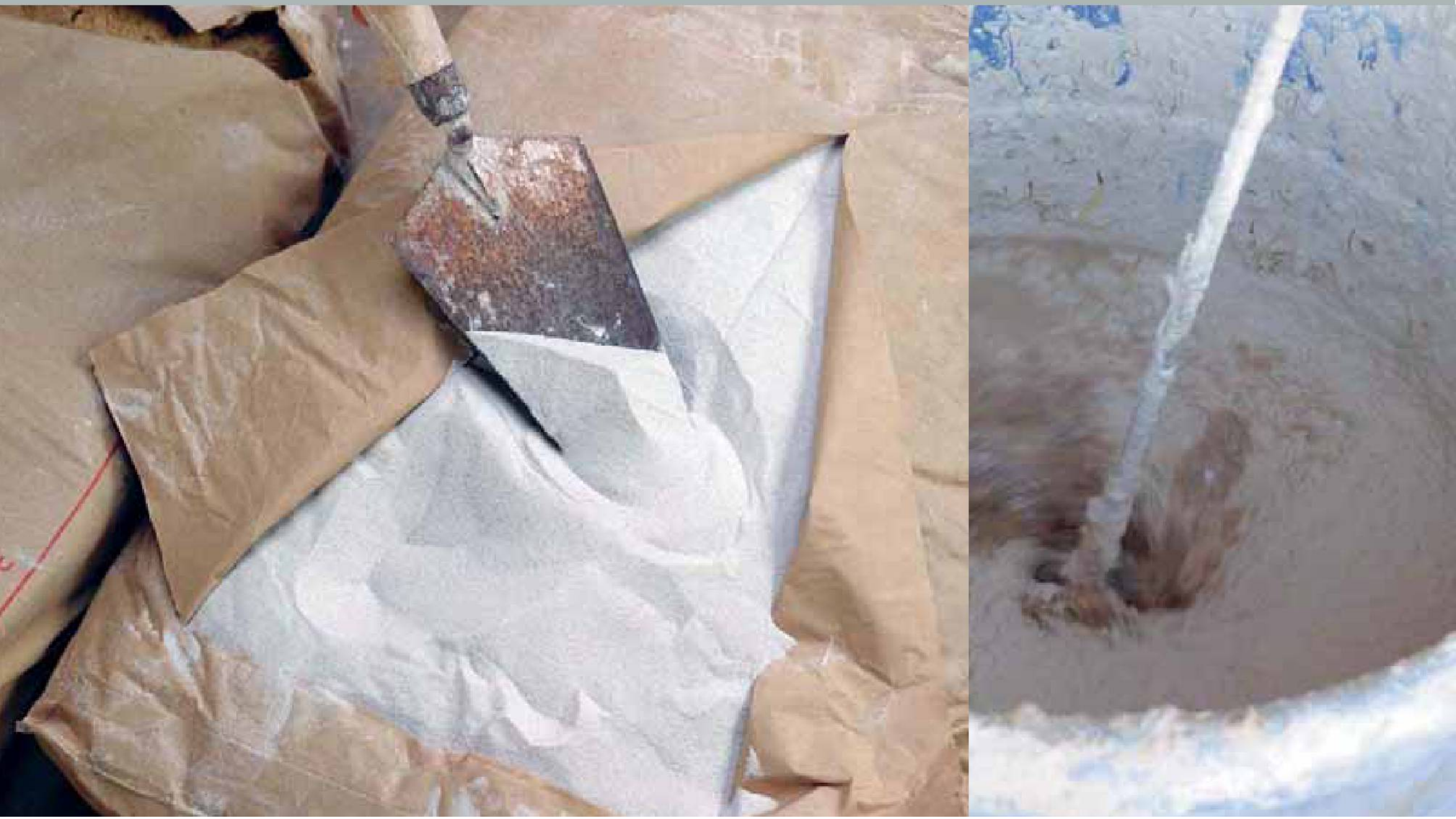
Left: Fine silica sand used for clay alis paint finishes. Right: Adding fine silica sand to a clay alis.
