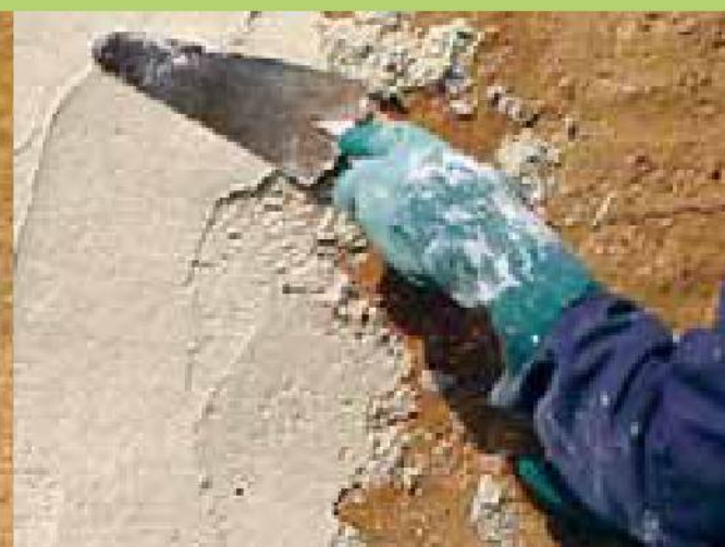
Apply further troweled or harled coat(s) as needed. Harled material can be pressed back or left rough.
