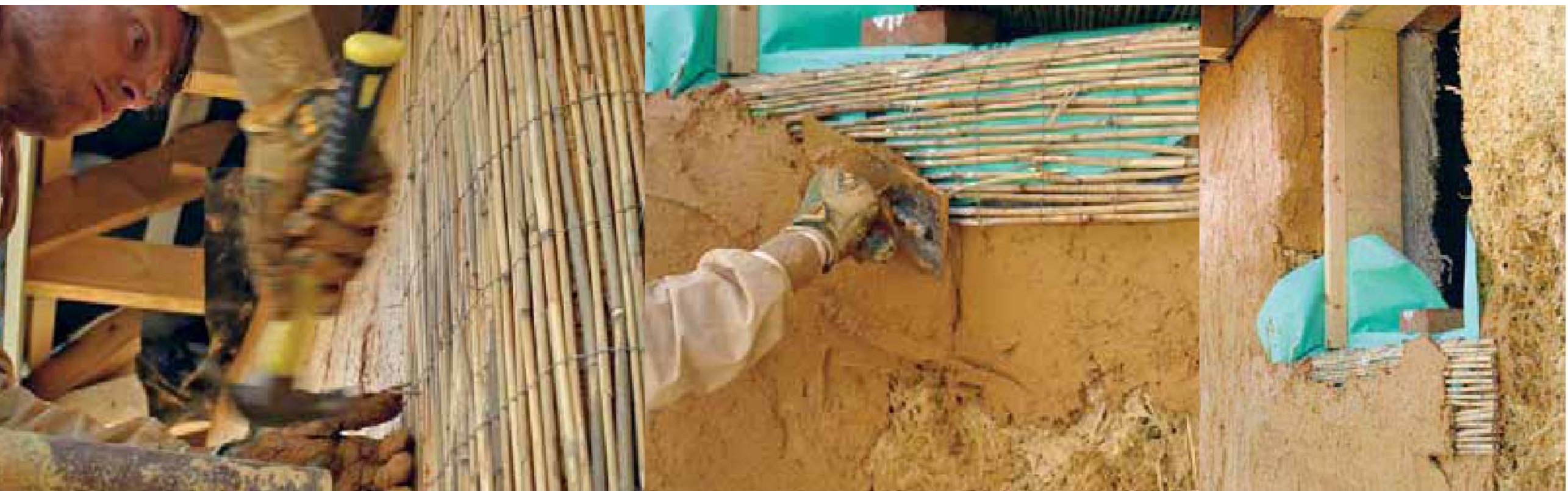
Above: Using reed mat to reinforce around straw-bale window openings. The earth plaster base coat is squeezed between the openings in the reed mat to help create a solid key.
