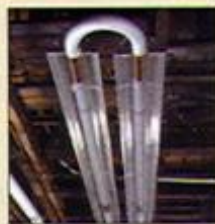
11 Heating and Ventilation
