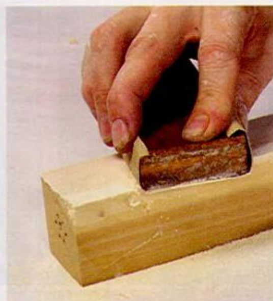
The two-part polyester resin used to repair this leg is tough, hard, and sands easily.
