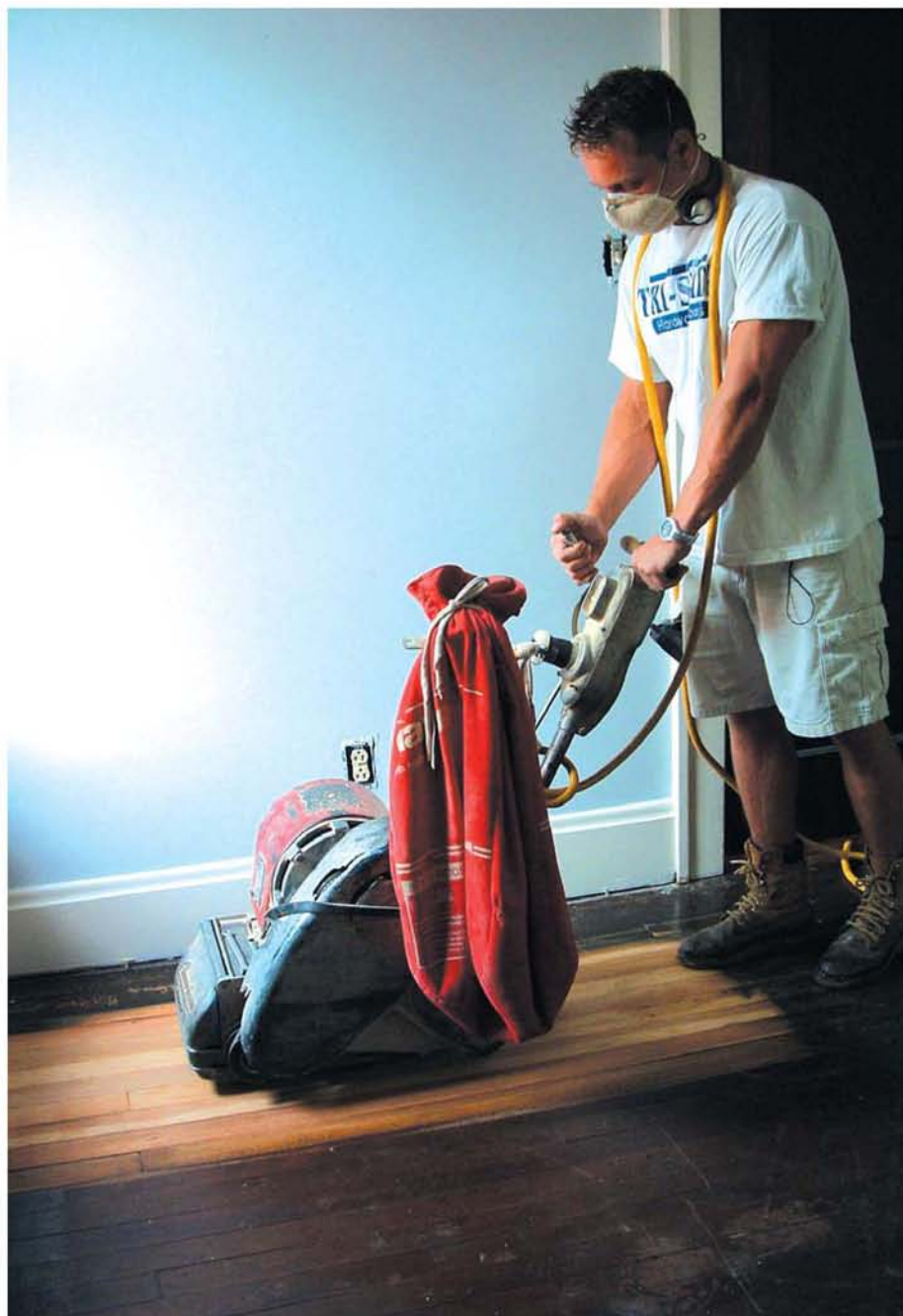
Rob McClanahan from Bethel, Ohio-based Tri-State Hardwood Floors, uses a stand-up sander to start the refinishing process. This type of sander can be rented at rental stores and some flooring-materials suppliers. Look under "rental" in your phone book or on the Internet under "floor sander rental."
