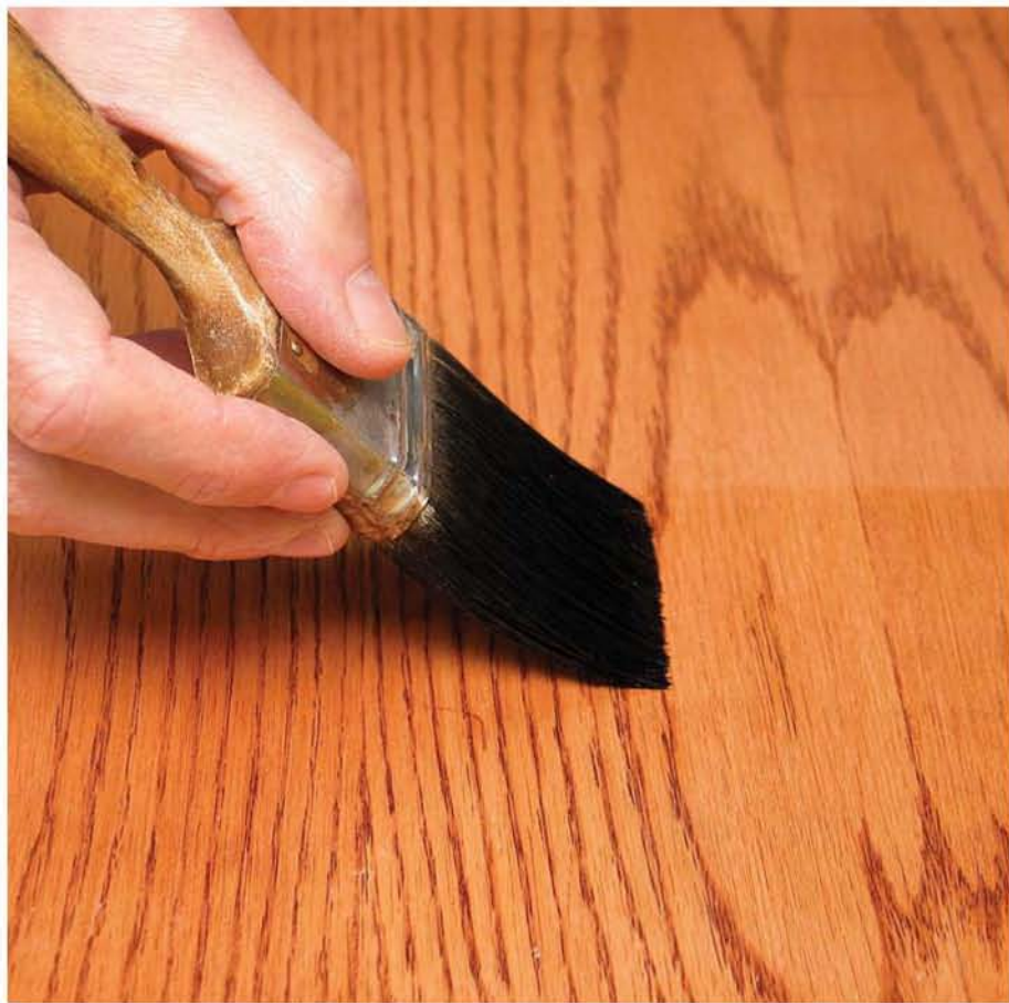
Myth 1: It's not necessary to brush across the grain, as I'm demonstrating here, to work the finish into the wood. The finish penetrates perfectly well by capillary action no matter how it is applied.
