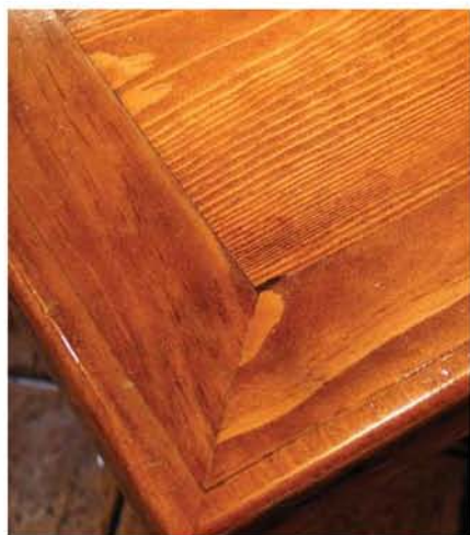
One of the thickest and most protective of all finishes is an epoxy-resin finish which is applied very thick and commonly used on bar tops and restaurant tabletops such as this one.
