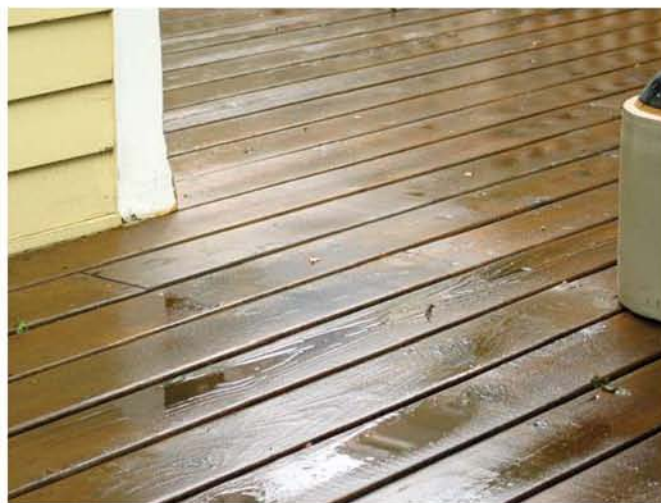
Because of compression shrinkage, all the boards in this deck have warped concave on the top even though they were laid randomly.
