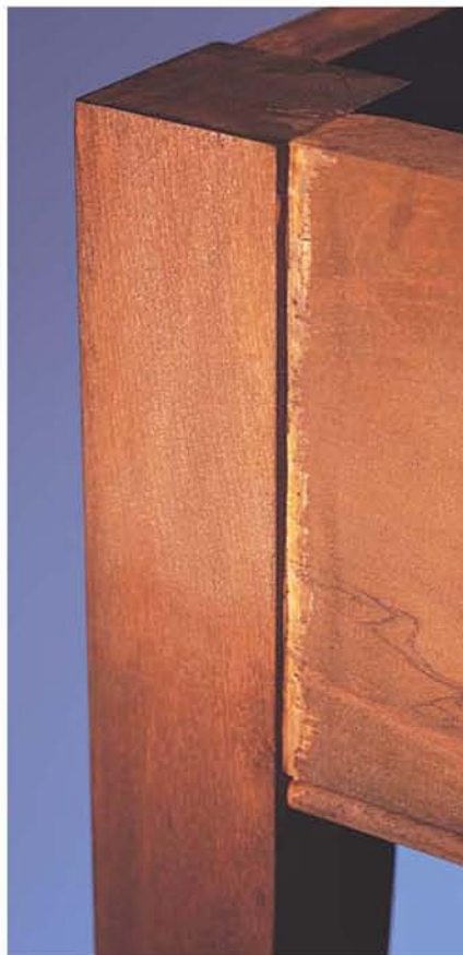
Glue squeeze-out is a particularly thorny problem when a joint meets at a 90° angle, such as a table leg to an apron. And because the apron is set back, it's easy to miss the squeeze-out during sanding.
