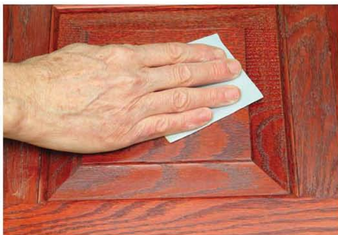
It's always best to sand between coats of a film-building finish to remove dust nibs. Use steatrated sandpaper to reduce clogging.
