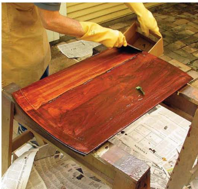
When the finish or paint is dissolved, blistered or loosened from the wood, scrape it into a box or can using a wide putty knife or plastic spreader.
