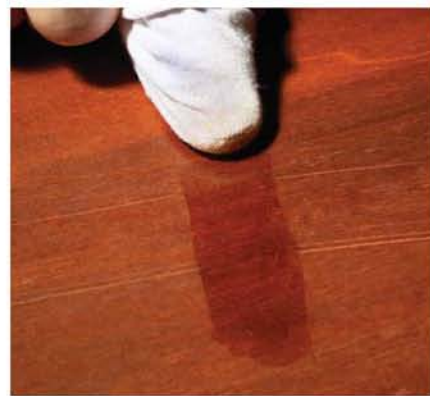
If a liquid is all you need to restore the color in a scratch, wipe the surface with an oil finish.
