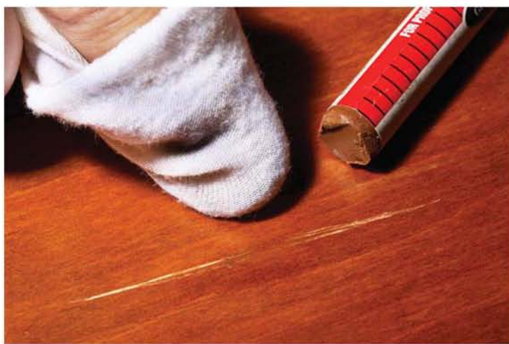
If a liquid darkens the scratch, just not enough, wipe the surface with a stain or colored paste wax.
