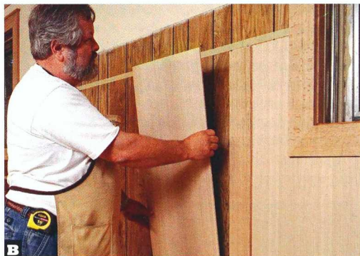
B Apply construction adhesive and slide the panels into place.
