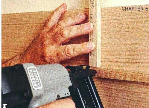
F A homemade gauge is more reliable than measuring for keeping the trim aligned.
