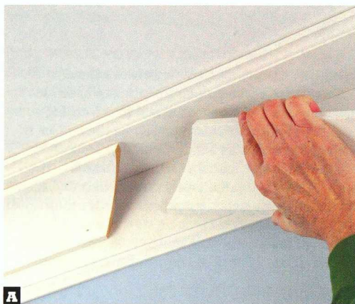
A Dress up the molding that goes against the ceiling by combining it with a molding that goes along the floor.
