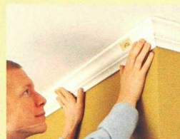
Installing crown molding 138
