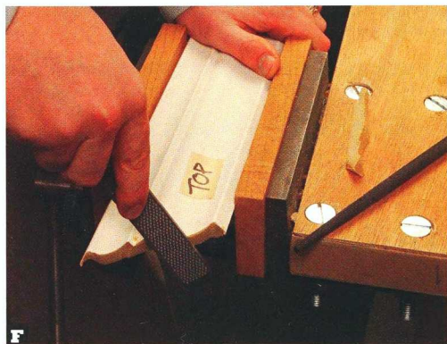
F Finetune the joint. File away high spots that are causing gaps. Measure the length of the molding and cut it to length with a 90-degree cut. Put the molding in place and nail it to the backer.
