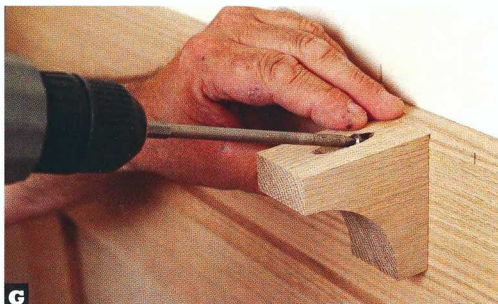
G Pocket-screw holes fasten the brackets in place. The shelf covers the opening.
