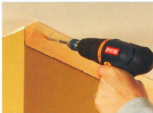
Drill pilot holes and use screws to fasten the backer to the studs in the wall.
