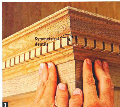
J Hold the mating pieces of dentil crown in place on the project and cut them so their miters are symmetrical.
