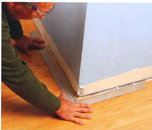
Outside corners are rarely perfectly square. Use a framing square to check a corner.
