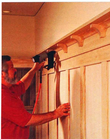
This is one project where a brad nailer really pays off in speed and neat installation.
