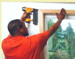
Trimming windows and doors 132
