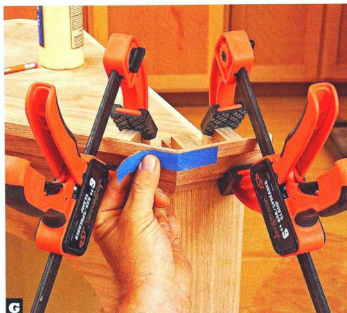
G Use clamps to hold the crown molding to the cabinet and apply painter's tape to help draw the miters tight.
