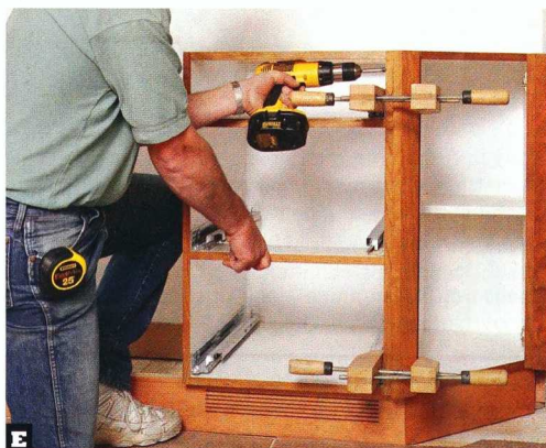
E If you build your base cabinets carefully and set the toe-kicks perfectly level, this step is easy. Clamp adjoining units together and attach them with screws.
