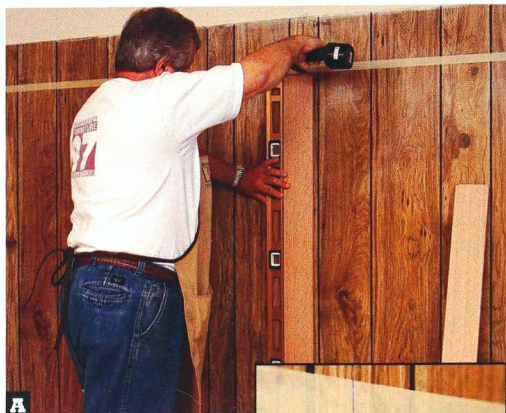
A Align the mullions to check your layout. The inset shows how to hold them before you're ready to nail.
