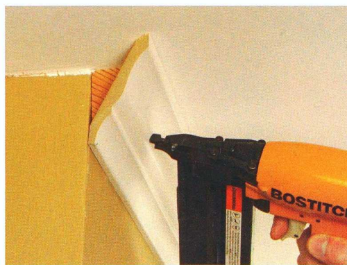
Beveled to the right angle, a backer strip assures that the crown molding will be at a consistent angle, guaranteeing tight joints.
