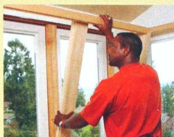
Prefabbing window trim 133
