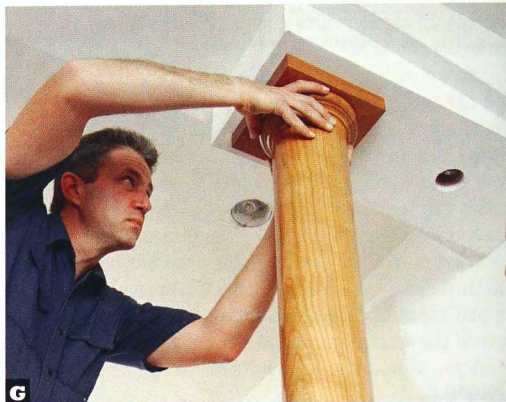
G Apply epoxy at both ends, then slip the column assembly onto the plinth. Turn the capital to lock everything in place.
