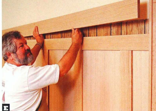
E Set the plate rail ledger atop the upper rail and fasten with finish nails.
