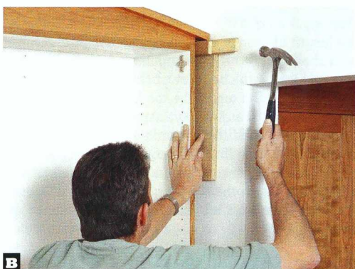
B Protect the wall with a board when you use shims like this. Remove the shims after screwing the cabinet to the wall.
