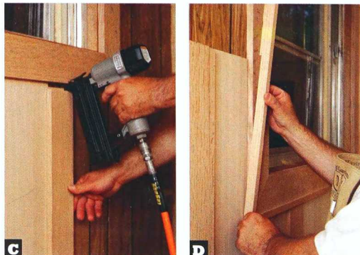
C Leave a gap between the window frame and adjacent mullions and fit the window trim pieces.
