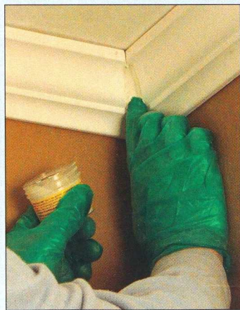
F Finetune the joint. File away high spots that are causing gaps. Measure the length of the molding and cut it to length with a 90-degree cut. Put the molding in place and nail it to the backer.
