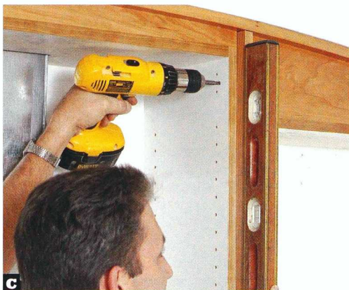
C There's no need to clutter up the inside of a cabinet with lots of screw heads. Fasten adjacent cabinets with screws placed inside hinge or shelf holes.
