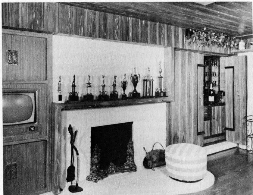
The pecky cypress on these walls and the ceiling has been finished with céruse , a thin white paint. After the wood is sealed, the paint is applied, then wiped off the background with rags. The paint remains in the pores, producing an effect similar to that of white filler.
