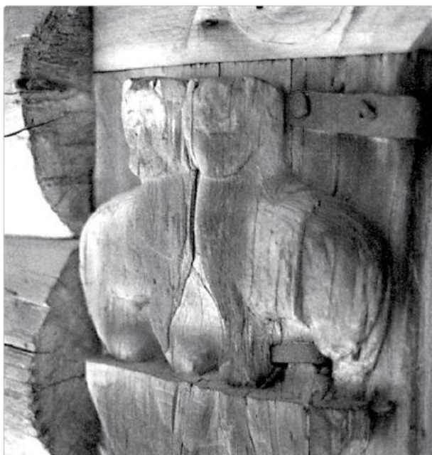
Doorframe detail on storehouse, Telemark, ca. 1300.
