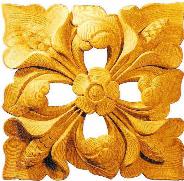
Fig 6.6 A Victorian ceiling boss in pine. Each element is supported by its neighbour to create the web of support that safely allows both the piercing and the thinning of the stems – an essential consideration when using wood which has little inherent strength
