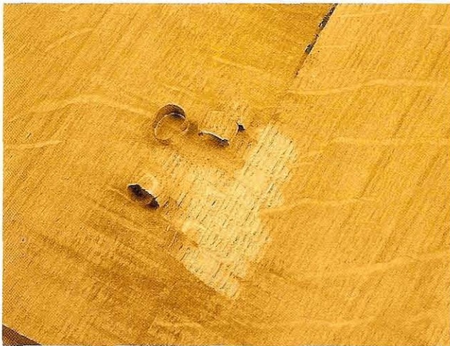
Fig 6.66 Careful grain-matching should make the joints almost invisible once they have been carved over
