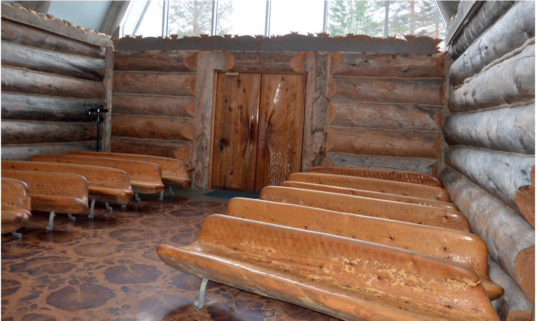
Figure 1.3. Interior detail of Ryynänen's chapel. The altar pews are shaped out of whole logs with outer bark only partly removed, decorated with floral patterns. A flooring of crosscut slices of tree trunks set in mastic allows viewers to see the rings and shape of the original trees. Eva Ryynänen (Finnish, 1915–2001). Täitelijan Temppeli (1991). Wood, glass, steel, mastic, electric lighting. Paateri, Lieksa, Finland.
