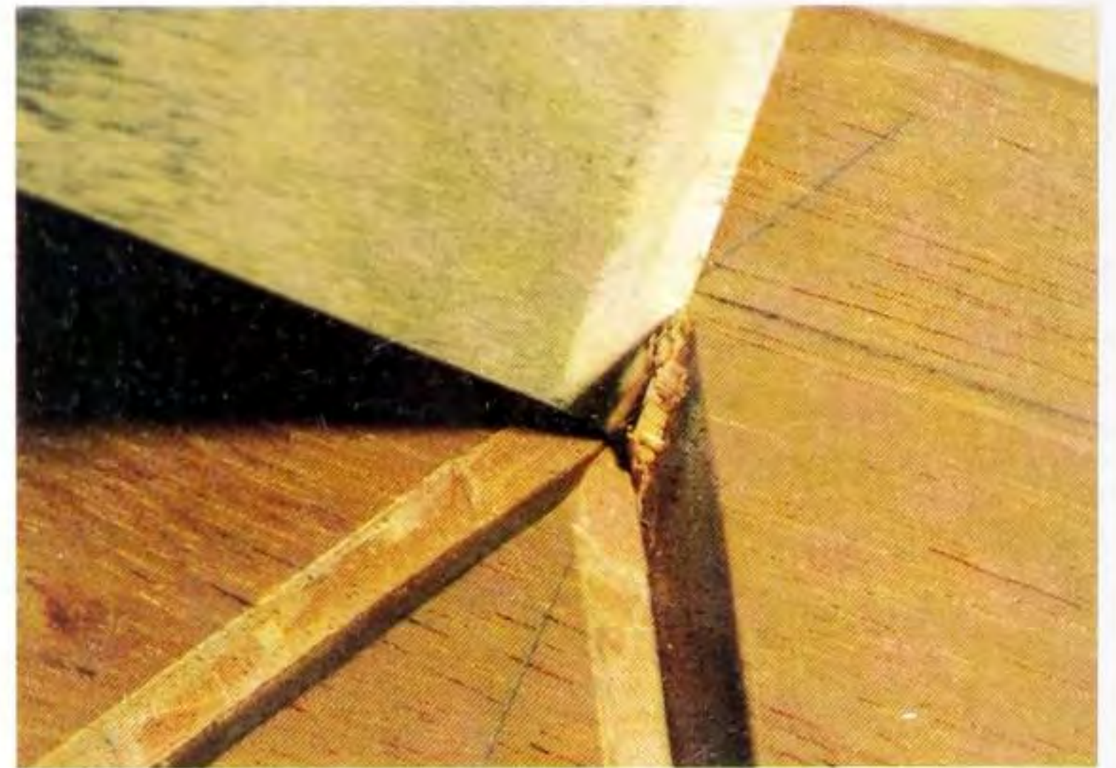
Fig 5.57 Finish off the apex with the corner of the large chisel.
