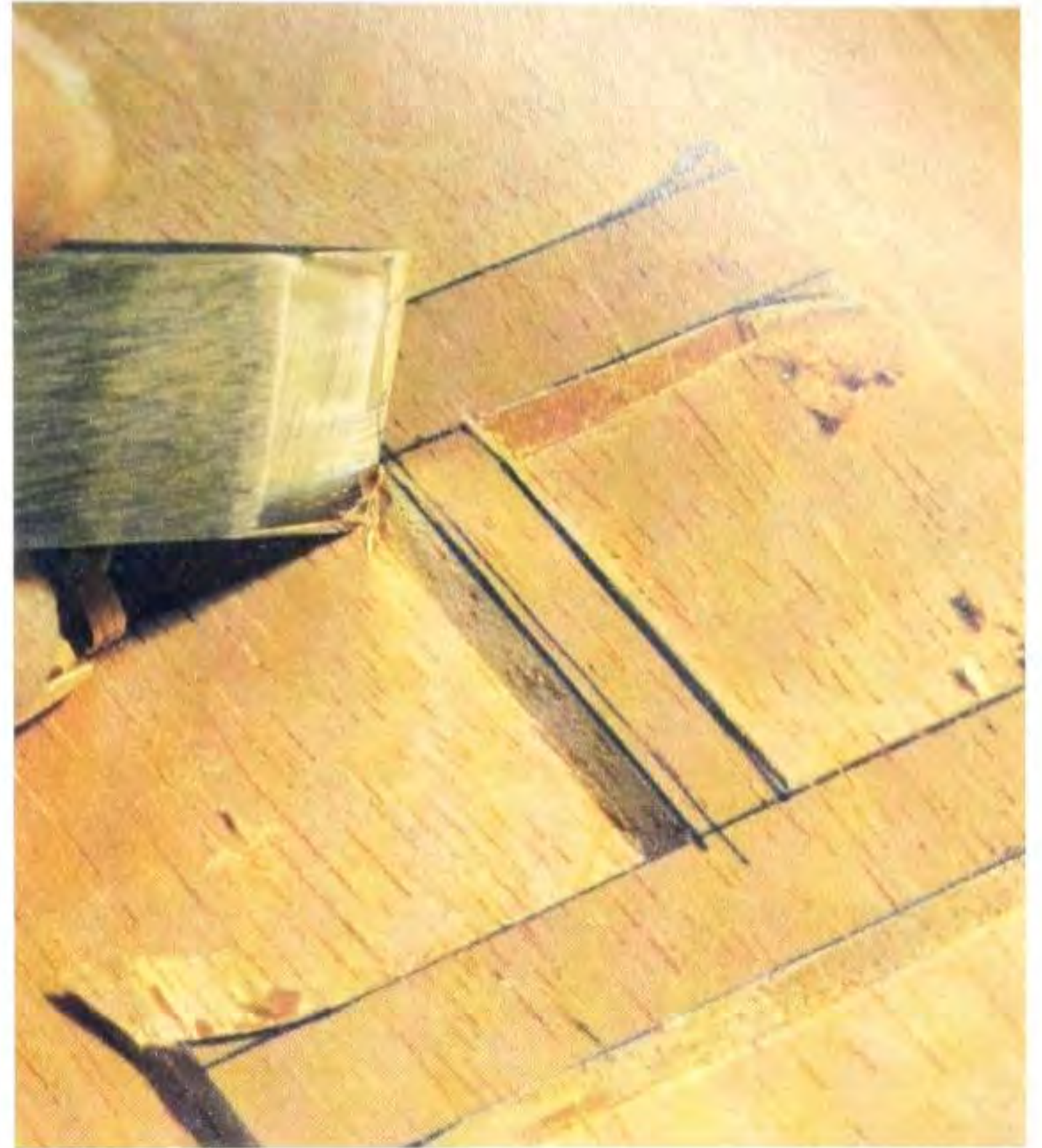
Fig 8.54 Making stop cuts into the corners.
