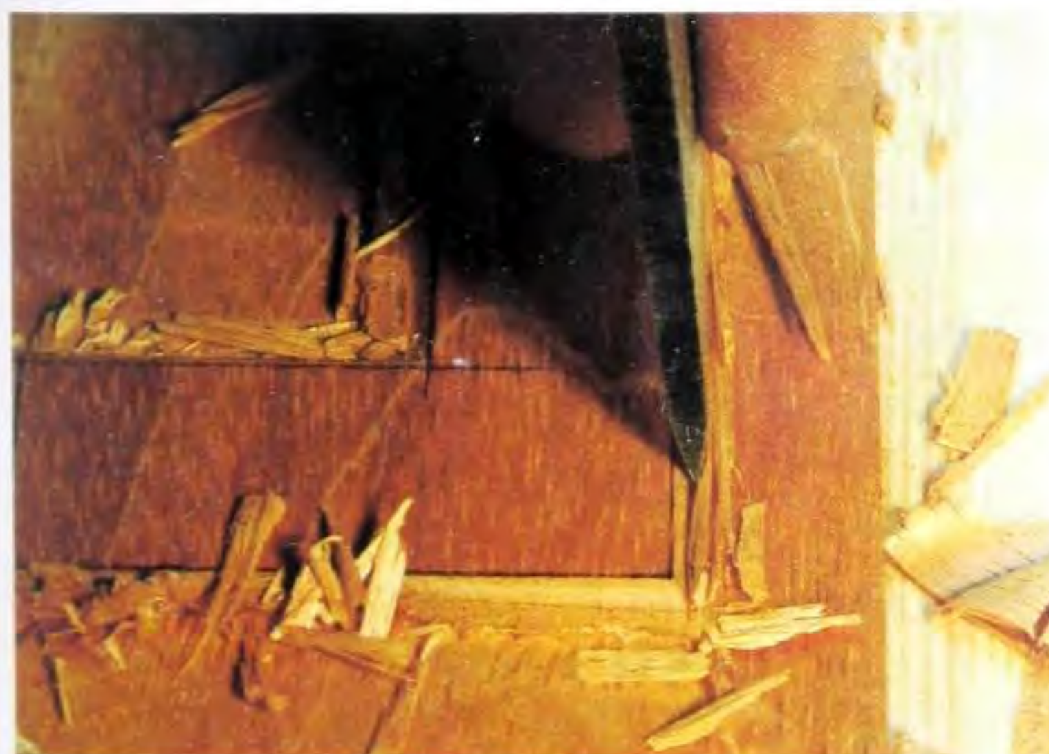
Fig 8.32 After lowering and levelling, trim up to the line with as wide a straight chisel as possible.
