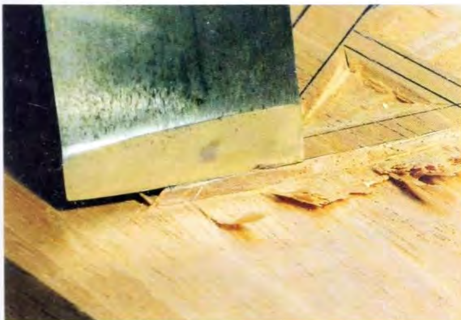
Fig 8.59 Setting in, after levelling, with the wide chisel.
