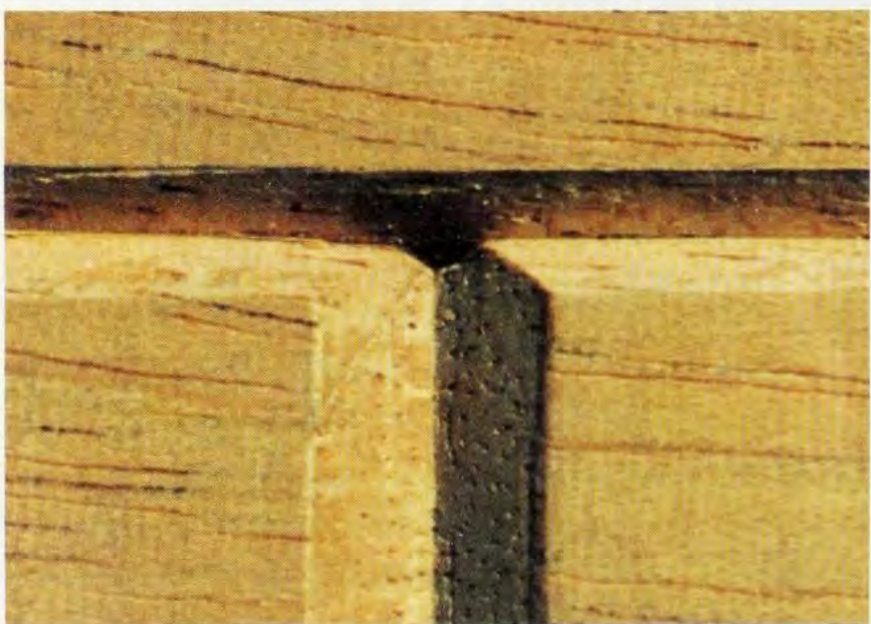
Fig 5.30 Close-up of the junction of a T, showing torn grain not visible at normal viewing distance.
