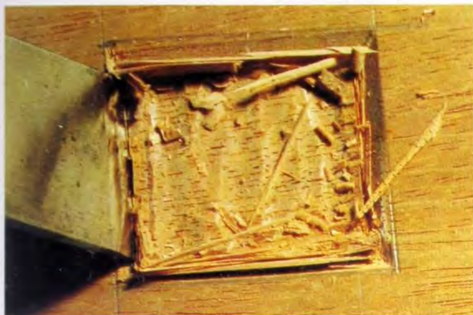
Fig 8.40 Setting in the walls with a chisel, which should be a little narrower than the sides of the square. Stop cuts will be needed in the corners.
