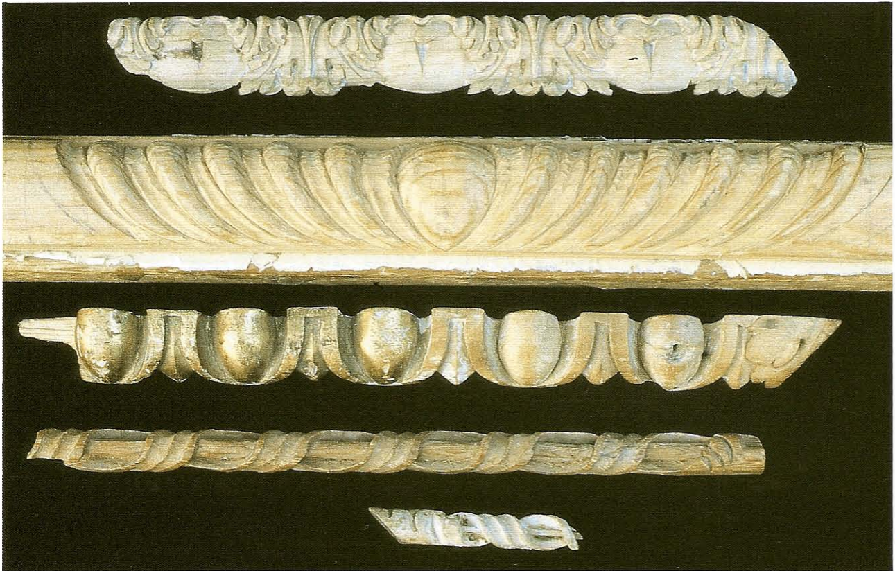
FIG 4.1 Various mouldings (from the top): an elaborate moulding on a cyma section carved in lime, originally gilded; a practice length of gadrooning in deal with U-shaped valleys between the gadroons (note the way the direction changes in the middle of the rail); egg and dart moulding with some of the gilding stripped away – the shadows around the eggs indicate the profile of the moulding (note the leaf at the right end used as half of the mask for a mitre joint); a practice piece of ribbon and stick in pine with an unsuccessful attempt at a leaf at the right end; a fragment of ribbon and stick with a typical leaf for disguising a mitre at the left end.
