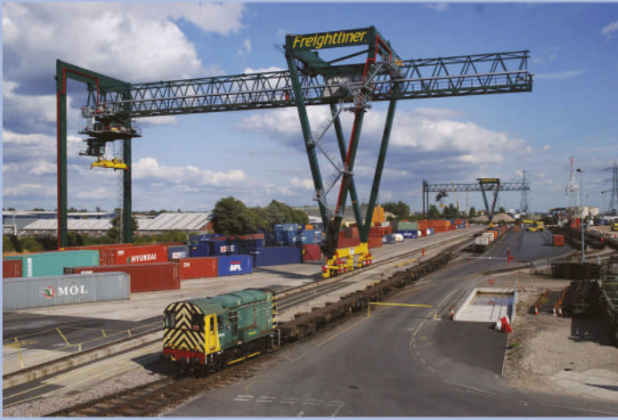
The additional sidings at Maritime have provided useful capacity for sustained growth at the port. Freightliner's pilot loco 08530 shunts empty flats in the sidings on August 22nd, 2014. The two gantry cranes had been installed two years earlier, replacing those that dated back to the 1970s.
