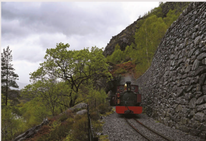
The Glaslyn Pass in North Wales has some particularly massive stone walls around the tunnels at the southern end of the pass, holding back the hillsides. It's quite the engineering achievement for what ended up being a lightly-used railway, but speaks volumes of the effort needed to build it.
