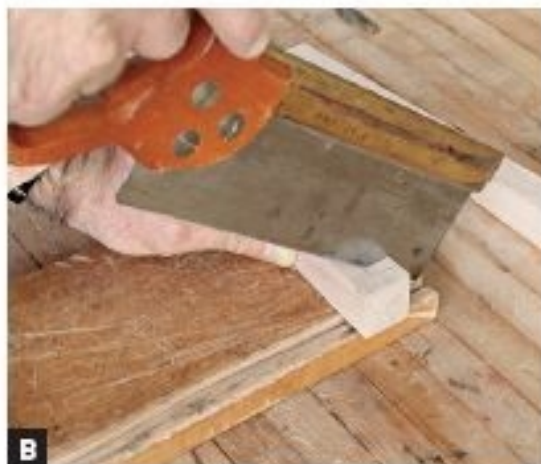
SAW THE EDGES of the mortises in the front posts at a 45-degree angle.
