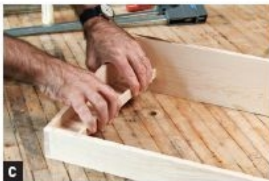
C PRESS THE TRAY IN PLACE by hand and check that it's level and straight. A little glue in the groove will secure it in place.
