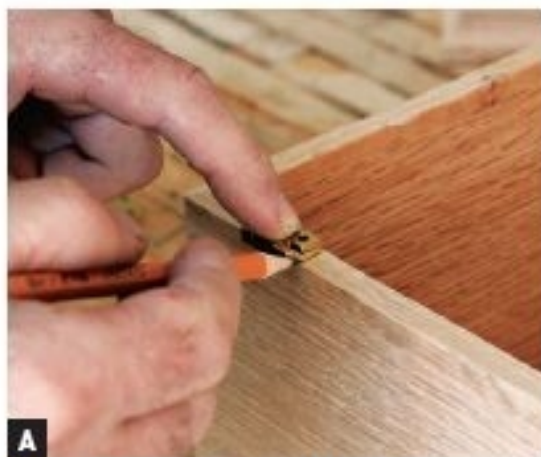
MARK THE LOCATION OF THE HINGES about 1 1/4 in. from the ends of the box.
