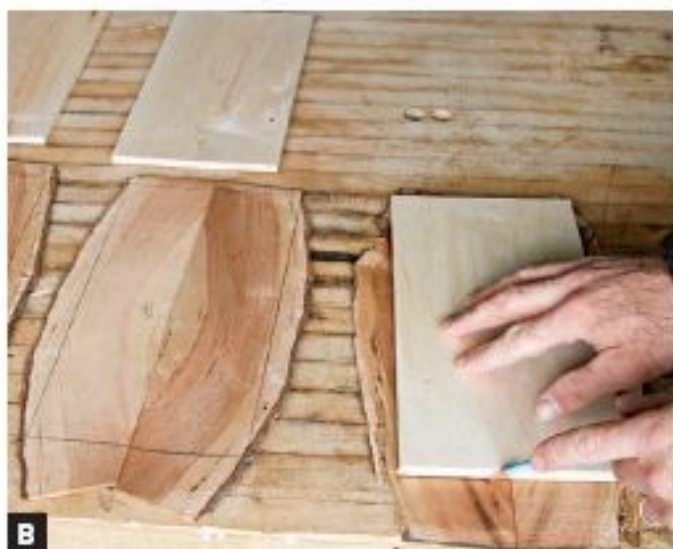
DRAW THE OUTLINE of the doors and interior sides on the veneer to size it correctly. B
