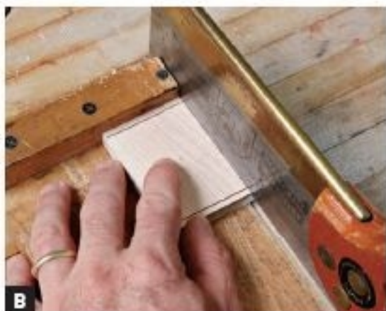
B SAW THE RABBETS on the back of the drawer front on a bench hook.
