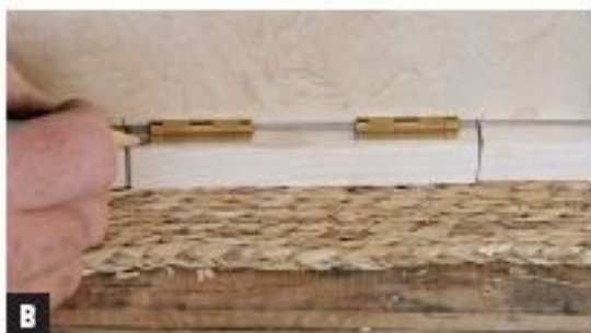
OUTLINE THE HINGES with the center of the top in place. Make sure the gaps between the top center and side pieces are even.
