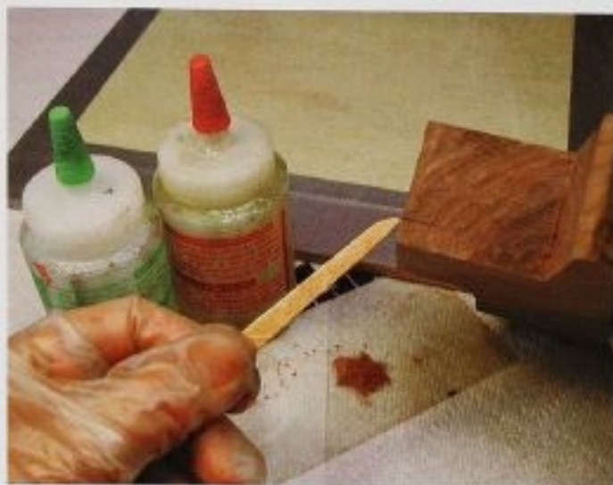
FIG. 45 When using epoxy to make a repair, mix the wood dust with one of the components first; then add the second component and mix thoroughly.
