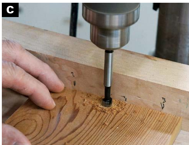
DRILL THE HOLE in the lid for the pin to form the swivel hinge. The \frac{3}{8} -in. drill fits the head of the pin; a \frac{7}{32} -in. drill is required for the body of the pin.
