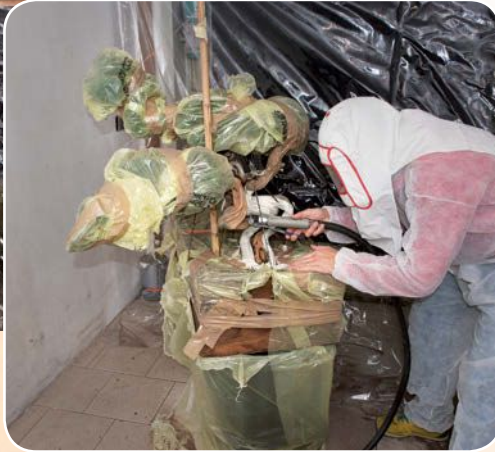
Then Massimo switches on the nozzle; slowly the deadwood is transformed by the sandblasting
