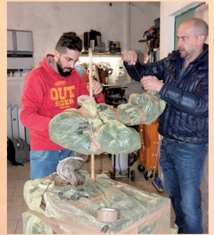
The branches are attached to a bamboo stick to keep them fixed in place during the whole blasting process
