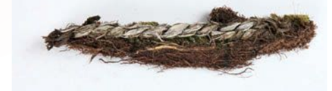
The hemp rope of the dam has already started to decay.
