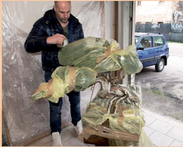
Mauro puts extra tape around the plastic bags to protect the foliage and so the bags won't be blown off when sandblasting
