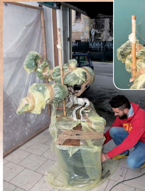
Almost ready to blast . . .
