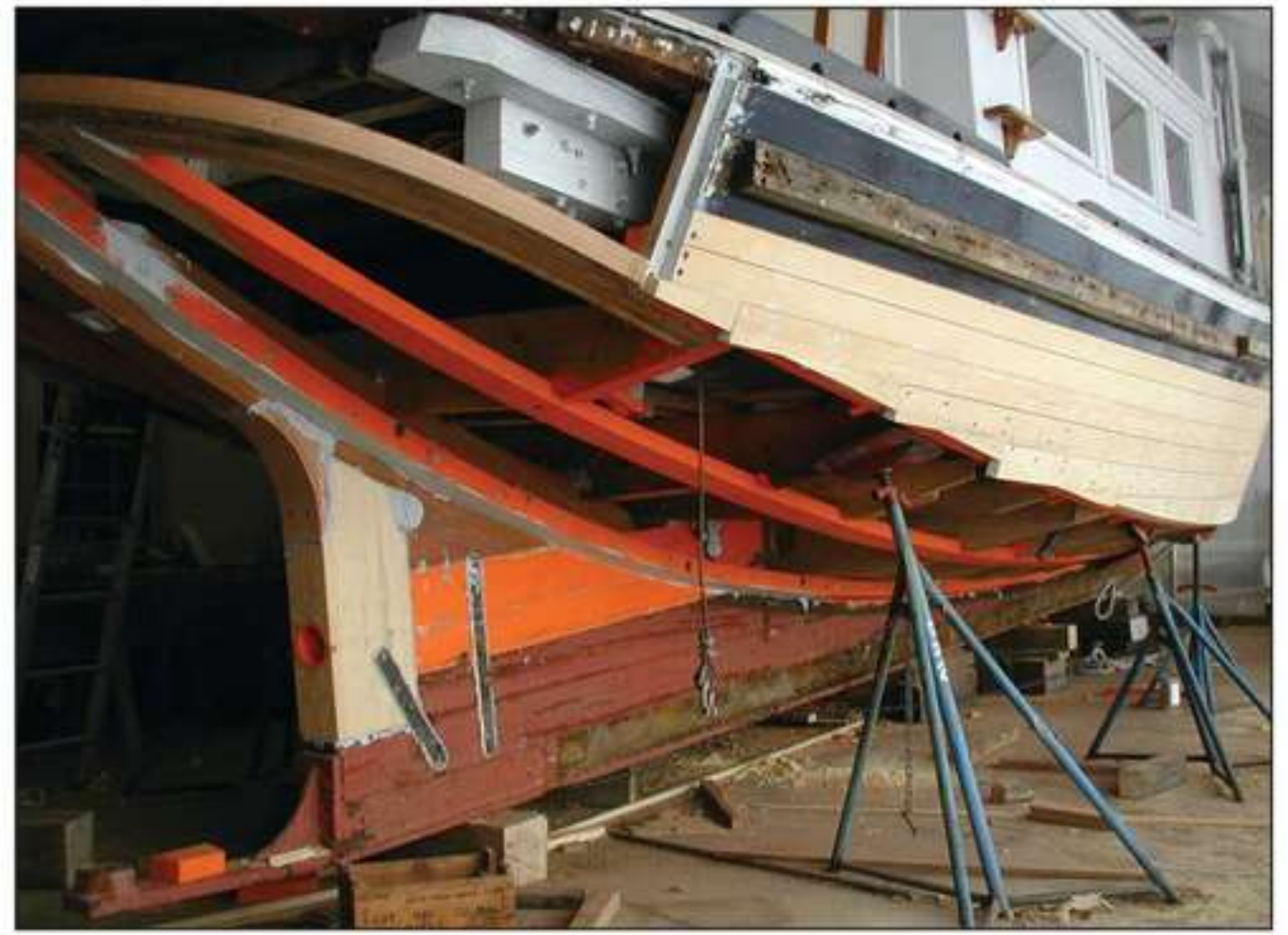
The early restoration phase also saw replacement of the boat's white-oak sternpost, as well as some topside planking in Alaska yellow cedar.
