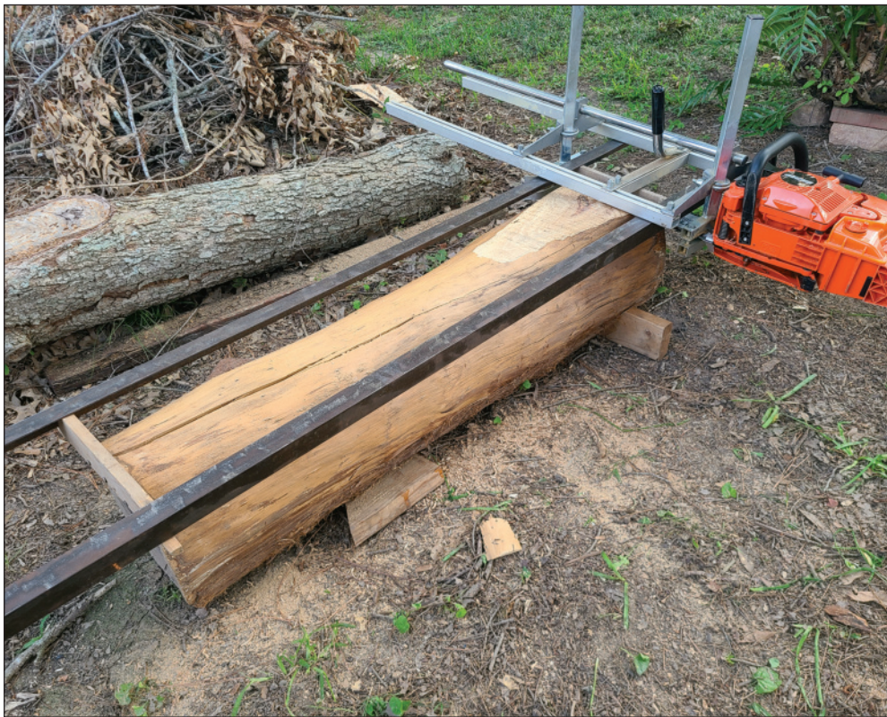
A rail guide system made of angle irons helps to establish a straight and flat first cut of the curved log. The rails are held in position by faceplates screwed into the ends of the log.
