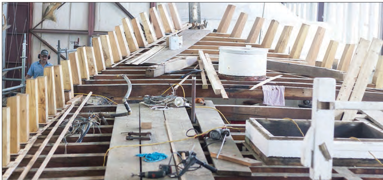
BOWDOIN's white-oak top timbers were mostly rotten, so Kyragoras and crew replaced all of them with tough, decay-resistant black locust. Aaron Freeman is on the staging, to port.
