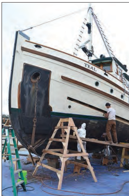
Above left —Since buying the boat in 2008, Kit Pingree has continued TEAL's maintenance and restoration. In 2016, the boat was hauled again at Port Townsend for additional work, mainly painting. Here, her 500-lb anchor is visible. Above right —In the latest haulout, a handful of planks needed replacement, exposing TEAL's heavy double-sawn frames.
