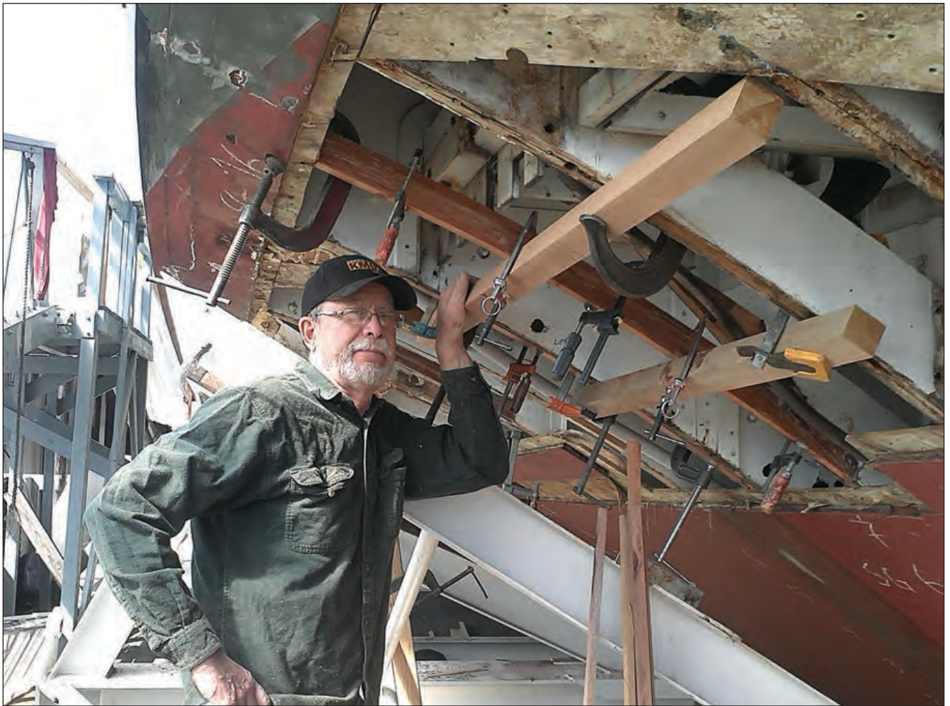
Ron Taylor laminates a section of framing in place during major structural work over the winter of 2012-'13. During this phase of the restoration, 18 bottom frames, 200 linear feet of planking, the lower portion of a watertight bulkhead, and most of the starboard shaft log were replaced.
