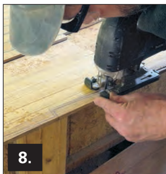
Photo 8 —After tracing the profile of the panel, Mike marked another line on the margin board exactly \frac{1}{4} " outboard of the traced line to allow for the caulking seam. Then he used a sabersaw to cut to the outer line and cleaned up the edges.
