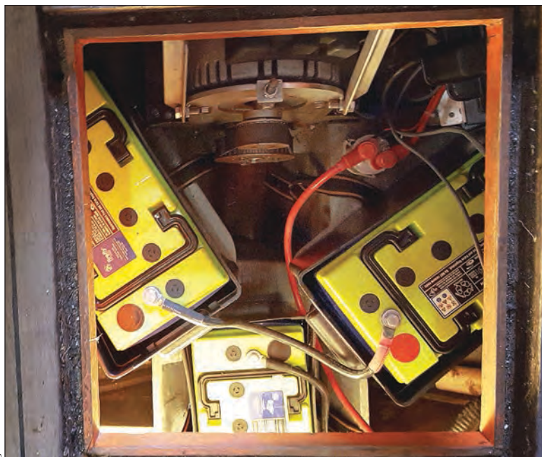
The electric motor and reduction gear, visible at the top of the photo, are smaller and lighter than the Atomic Four gasoline engine that they replaced. Two of the three 12-volt batteries visible here are part of the four-battery bank that supplies the motor; the third is a house battery. Red cables lead to the gray contactor, or solenoid, and at the extreme upper right is the motor controller.
