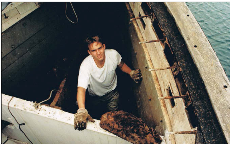
With the foredeck removed, Jeffrey took advantage of the opportunity to clean out the anchor chain locker.
