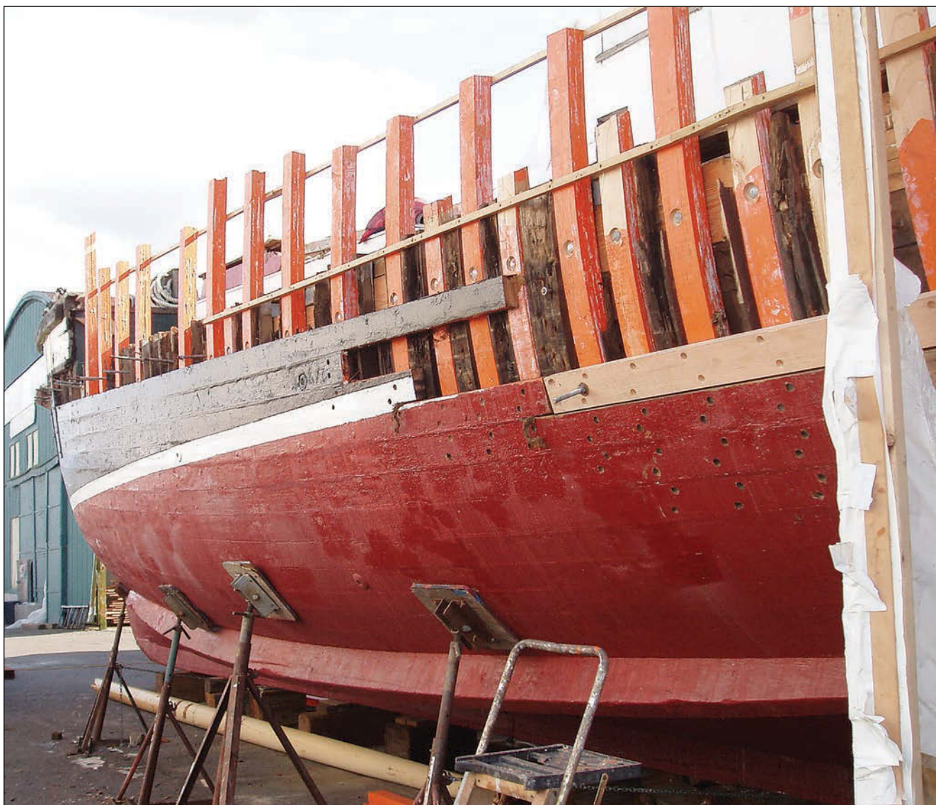
During a six-month haulout in 2004–05 laminated sister frames were installed, along with about 1,000 bd ft of new planking. This was the most extensive project since DAVID B's purchase in 1998, and by the following summer she was ready for her first charter customers.
