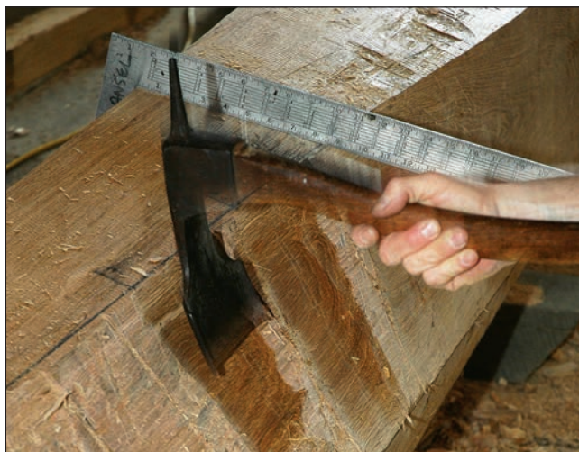
Adze work typically involves working across the grain. Here, Walter Ansel uses an adze to shape a large and complex timber during the restoration of the 1841 whaleship CHARLES W. MORGAN at Mystic Seaport in Connecticut.
