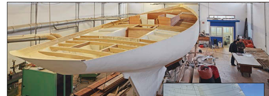
Beside the River Linge in Heukelum, Holland, Pieter van der Aa is building—by himself—a 55' Sparkman & Stephens yawl. This is his second S&S yacht, following his construction of the 48' MASQUERADE (inset), which was accepted into the New York 32 class with sail number 21.
