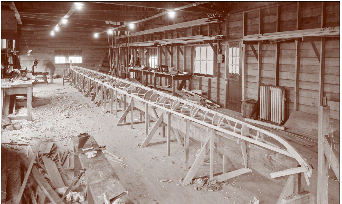
Above—Pocock's well-lighted shop in the Washington shell house featured a long, well-supported beam on which he built his 62' eight-oar cedar shells.
