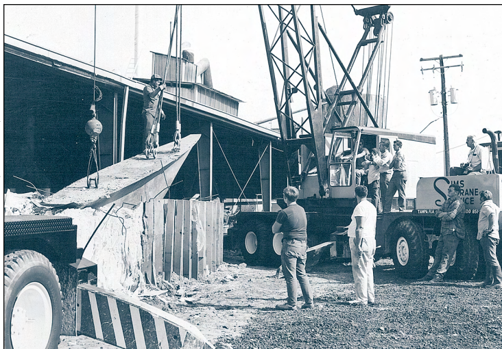
Morgan Yachts made the mold for the keel. The keel itself was poured by Gulf Coast Lead in Tampa; here, a crane lifts it from the mold.
