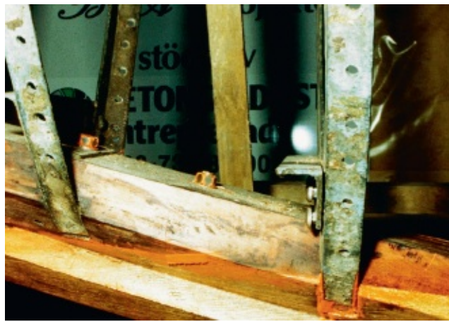
FIGURE 132 } The stem joint of Beatrice Aurore . A well-bolted hook joint between old and new. The joint is drawn together by the wedge, which is visible in the middle of the joint. It may be a double wedge that is tapped in from both sides or, in this case, a wedge-shaped recess that the wedge is tapped into.
