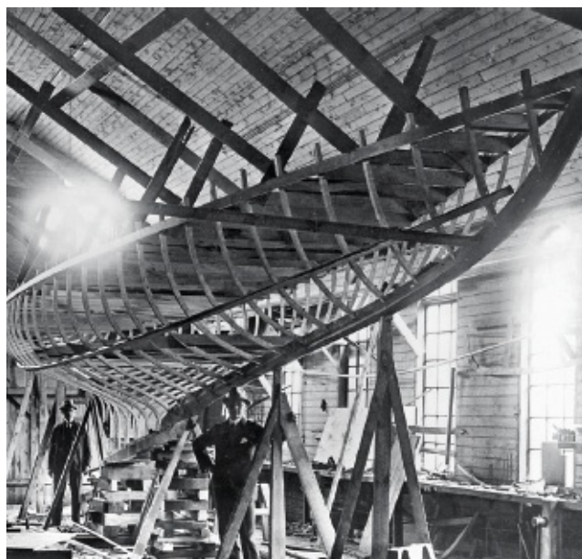
FIGURE 99 } The 2 SK 95-sq.-m. Marga III (18.30 × 2.80 m) under construction at the Stockholm Motorboat yard in 1918. The backbone is now finished, and the steel frame has been set into it. The frames are secured both lengthwise and
