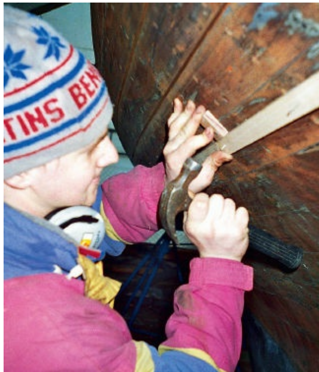
FIGURE 82 } Nailing the guide bar using the distance gauge.
