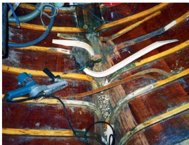
FIGURE 96 } Replacement of parts of the ribs. The picture also shows the old frame pieces, MDF templates, the belt sander and a spoke shave.
