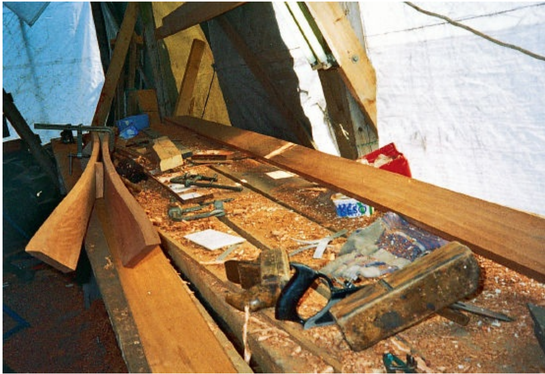
FIGURE 130 } Two planks (in Swedish called crying planks) aft by the top of the rudder post. The planks are \frac{3}{4} " (20 mm) thick in finished condition and cut out of 3\frac{1}{6} -inch- (80-mm-) thick timber. At the front of the photograph are a caliper, a bull-nosed rabbet plane, and curved wooden planes.
