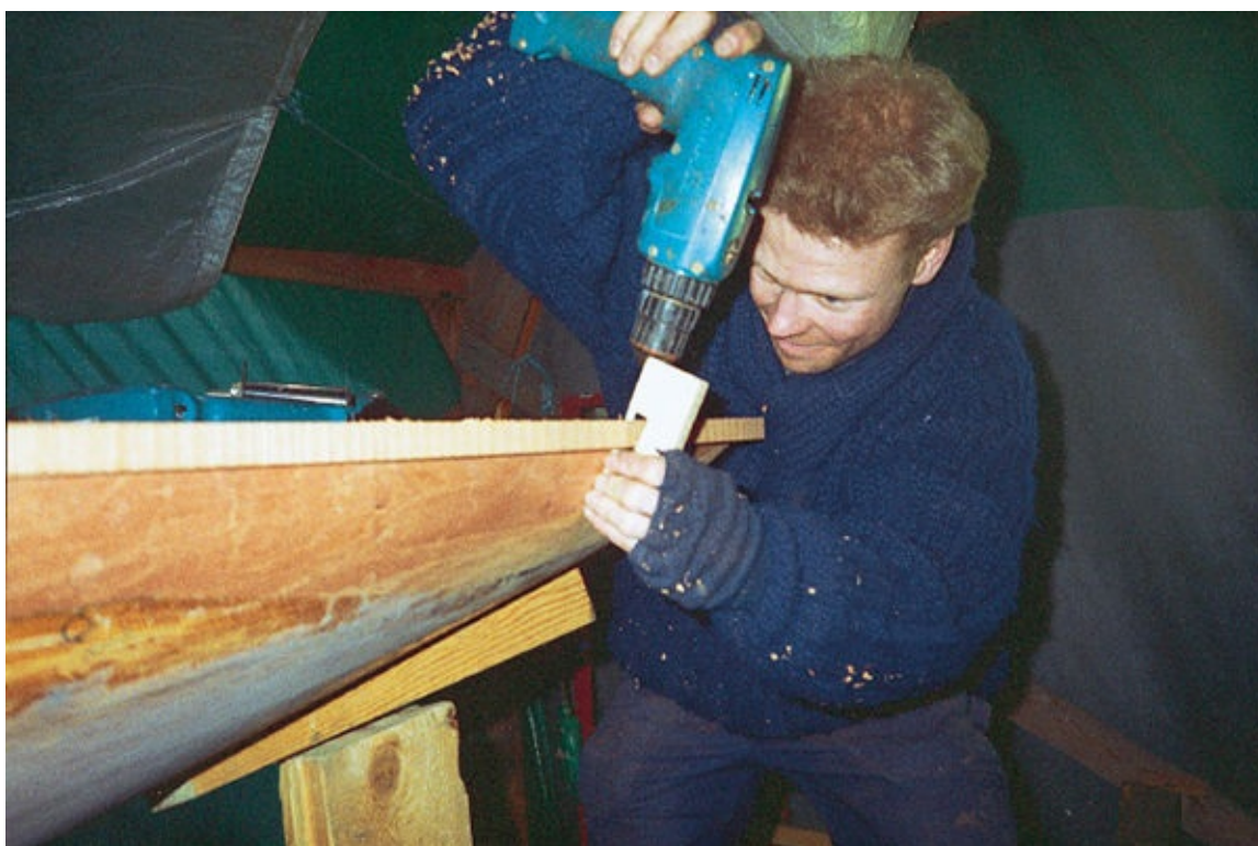
FIGURE 173 } Drilling a side deck screw with a guide.
