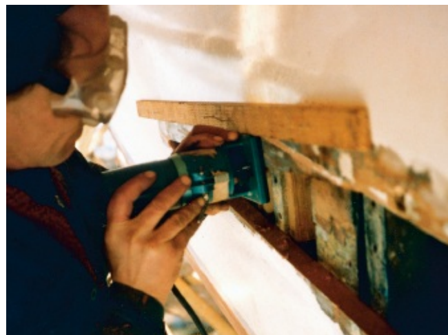
FIGURE 73 } Routing of the plank edge with a router; in this case, the hole has first been roughly cut with a circular saw. The edges can then be cut with a router blade with a large radius that provides smoother cutting surfaces. If you cut the hole directly with the router, use a blade with a smaller radius, which does not require the same amount of force for cutting, but the surfaces will be more uneven.
