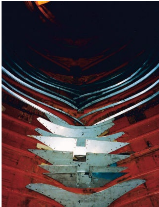
FIGURE 104 } New frames and floors ready for installation.
