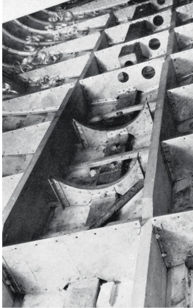
FIGURE 203 } External engine bed and steel floors forming the truss that holds the shape of the bottom. The inner engine bed is not mounted yet. The hole for the propeller shaft is visible, as well as holes for the exhaust pipe in the aft floors. The image is from Segel och Motor (Sail and Motor), 1936.
