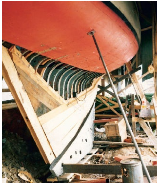
FIGURE 138 } Changing the keel on the 95-sq-m Skerry cruiser, Kerma . The large knee (deadwood) aft has been added, as the bilge was so deep and narrow that it was impossible to keep it clean. The knee wasn't covered by the planking but got a rabbet in its leading edge so that moisture would not get trapped between the planking and the large knee.
