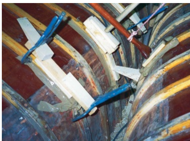
FIGURE 97 } Repairing frames in the turn of the bilge. The pieces are easy to make, but necessity is the mother of invention in terms of fixation while gluing.
