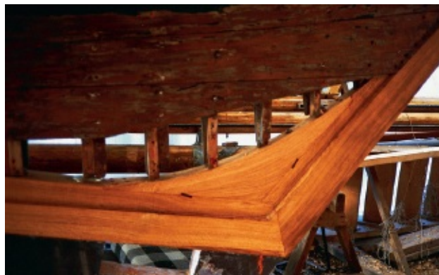
FIGURE 149 } Knee with wooden wedges. The sternpost is tucked in between the old plank ends.
