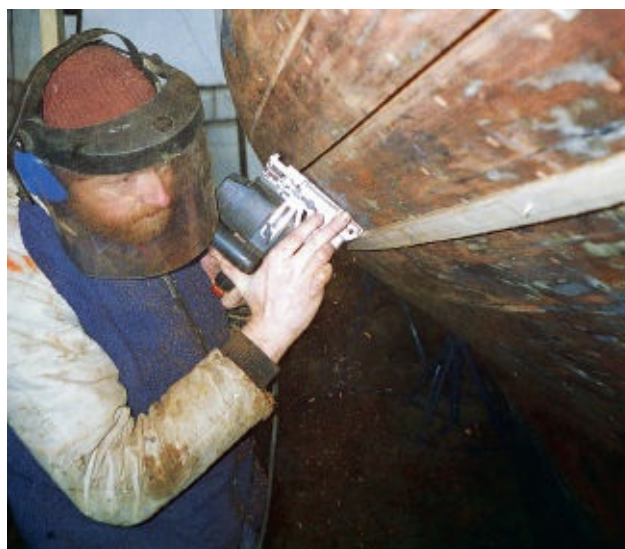
FIGURE 76 } Cutting grooves with a circular saw equipped with a conic scored blade. Sawing is controlled by using a guide attached with nails. The seam above is already sawn up. Once you have strips that fit, you can cut several tracks at once, but if the strips are too hard, the planks will be displaced when the strips are driven in and the last traces will become too thin.
