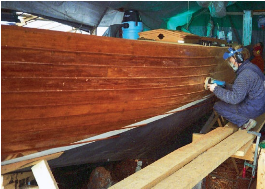
FIGURE 86 } Trimming of surplus strips.
