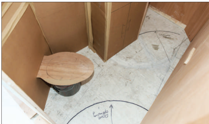
Above —This mock-up of the complex shape of a tiny head compartment includes a bucket for the toilet and marked clearance of a door that will swing open into the limited space. Right —Roscioli, carpentry foreman Hernan Jimenez, and Koch discuss the consistent shape and height of the interior doors for the finished boat.
