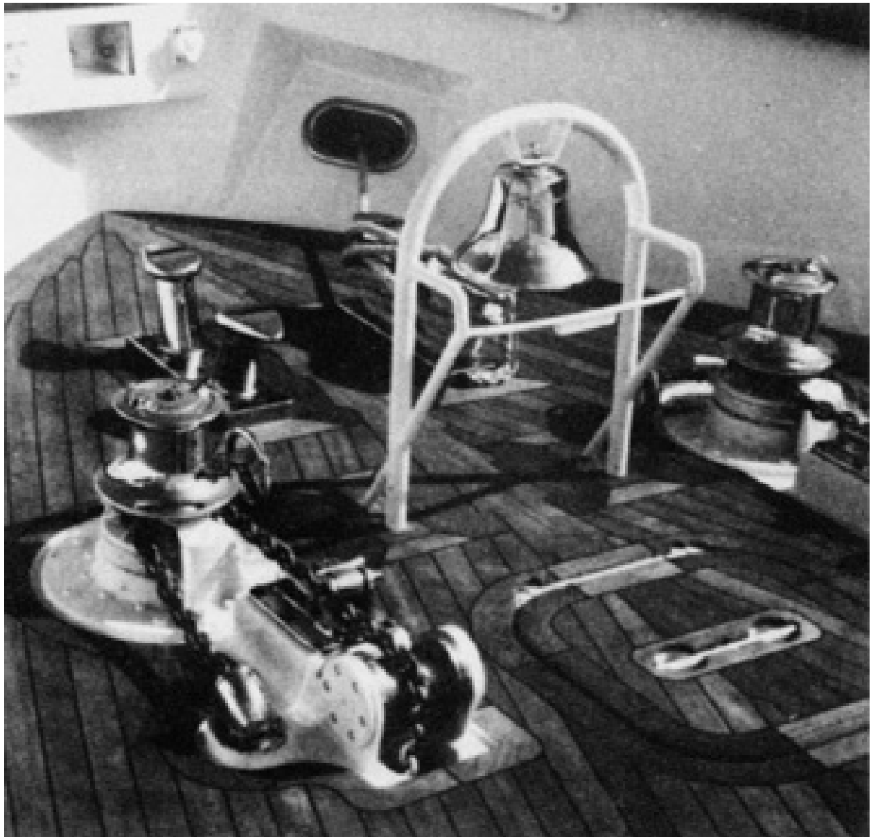
FIGURE 13-5. Installation of prefabricated teak decking on a large yacht. ( Teakdecking Systems )
