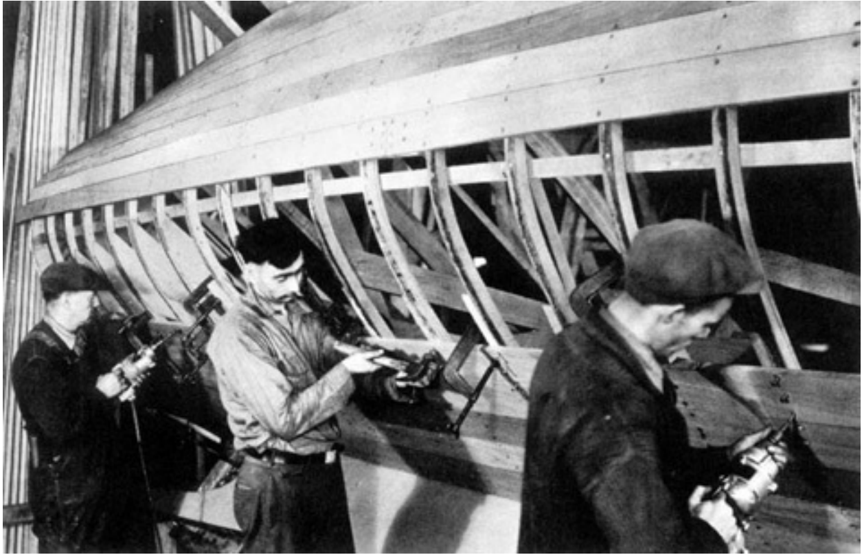
FIGURE 3-10. Boatbuilding, despite all the changes in tools, still involves the forming and fastening of materials into the shape of a boat. In addition to the electric drills and screwdrivers visible here, there are nine C-clamps keeping the plank in place for fastening to the frames. Note that the hull has been tilted to make the bottom more accessible.
