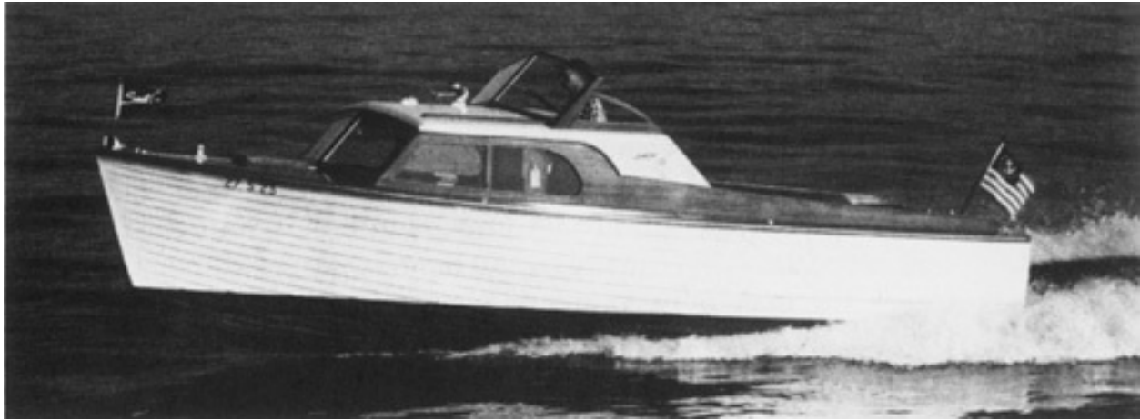
FIGURE 11-14. A 23-foot boat designed by the author and built under his supervision, with plywood lapstrake planking, all strakes scarphed with a dogleg similar to that shown in Figure 11-32 .
