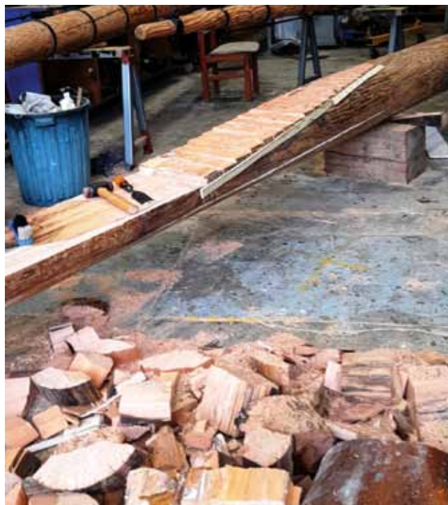
FIGURE 3 – Firewood pile demonstrating extent of rot.
