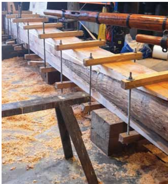
FIGURE 8 – New Oregon slabs glued and clamped.
