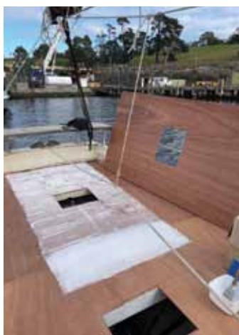
SECOND LAYER of ply going on. Image Peter Manthorpe
