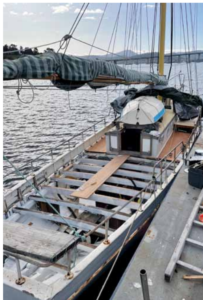
NEW BEAMS in place, first layer of ply going on. Image Peter Manthorpe
