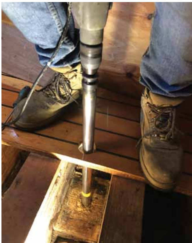
DRILLING OUT THE keel bolts with a specially made long hole saw.
