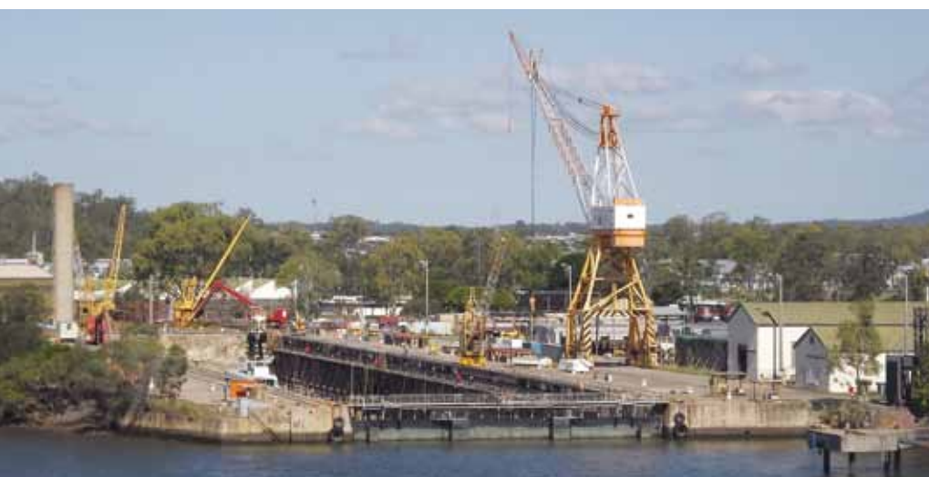
TOP: Cairncross Dock under construction in May 1943. Image QMM collection
