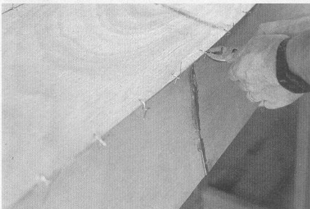
Wire the bottom panels to the sides.
