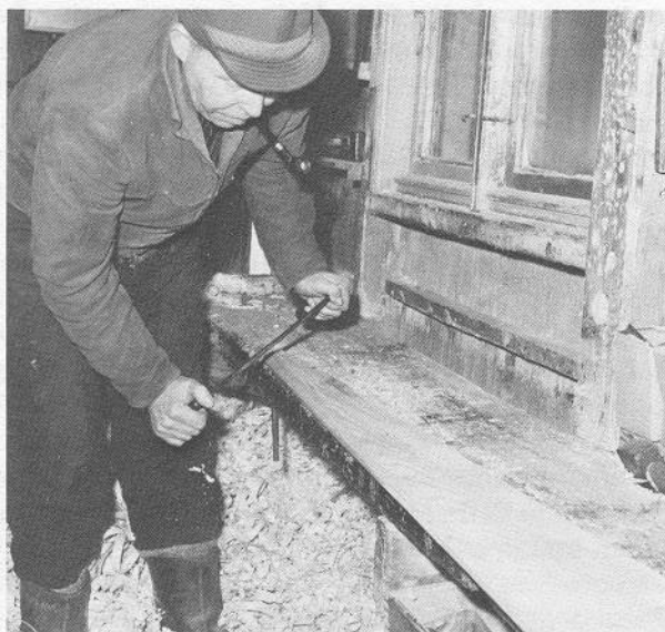
The bevel on the bottom plank is shaped with a drawknife.
