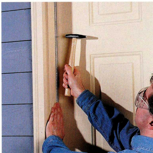
A reinforced felt strip can add rigidity in high-impact areas, such as doorstops, that tend to develop air gaps.
