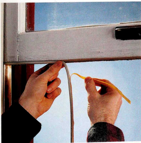
Self-adhesive foam strips are an easy way to seal air gaps around window sashes and door frames.
