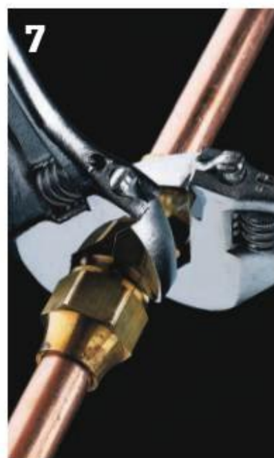
7 Hold center of flare union with adjustable wrench and use another wrench to tighten flare nuts one complete turn. Turn on water. If fitting leaks, tighten nuts.
