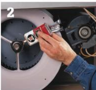
Remove the covers to the oil ports and add a few drops to each port.
