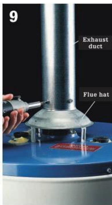
Attach the flue hat to the exhaust duct with #4 gauge \frac{3}{8} " sheetmetal screws driven every 4".
