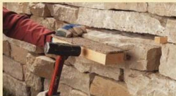
Use a 2 × 4 covered with carpet to avoid damaging the stone when hammering it into place. After hammering, make sure a replacement stone hasn't damaged or dislodged the adjoining stones.
