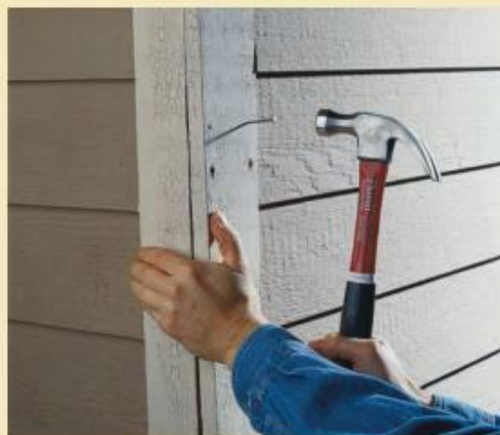
Evaluate broad trim pieces , such as the end cap trim shown above, and make repairs, using the same techniques as for siding.
