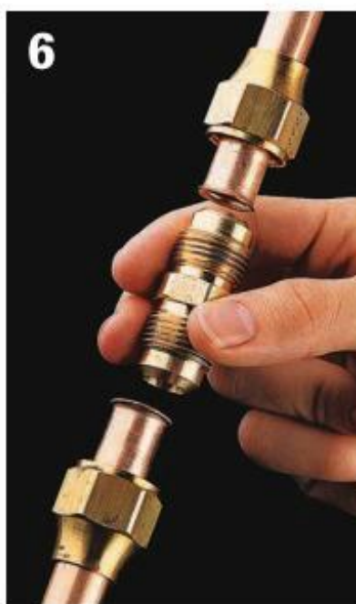
6 Place flare union between flared ends of pipe and screw flare nuts onto union.
