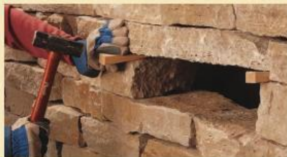
Return a popped stone to its original position. If other stones have settled in its place, drive shims between neighboring stones to make room for the popped stone. Be careful not to wedge too far.
