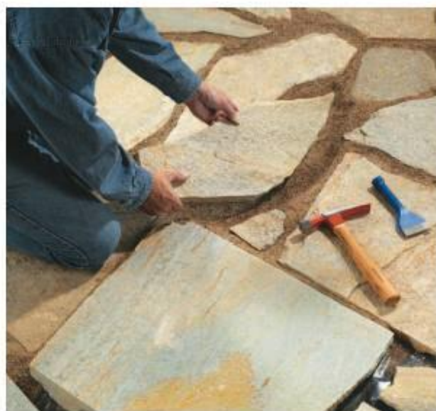
Replace a sandset flagstone by lifting out the damaged stone, leveling and tamping the sand bed, and setting in a new stone and repacking the sand joints. Trim and dress the new stone as needed.
