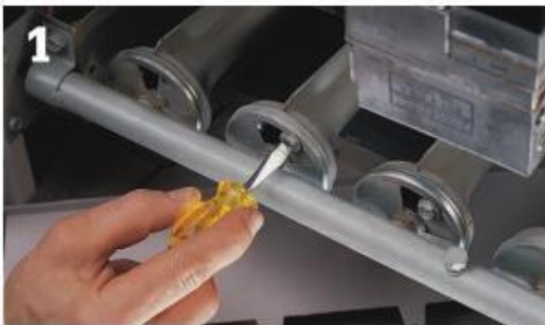
1 Remove the screws holding the burners to their brackets or to a slide-out pan.
