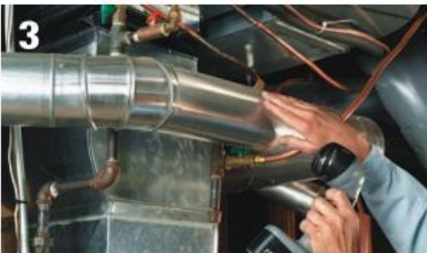
Inspect the areas around vent pipes for signs of corrosion. Corroded pipes will need to be replaced.
