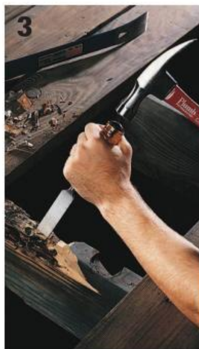
3 Use a hammer and chisel to remove any rotted portions of joist.
