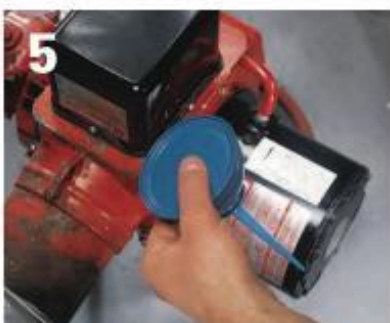
5 Add lubricating oil to the ports or cups. The motor housing may indicate what kind of oil to use.
