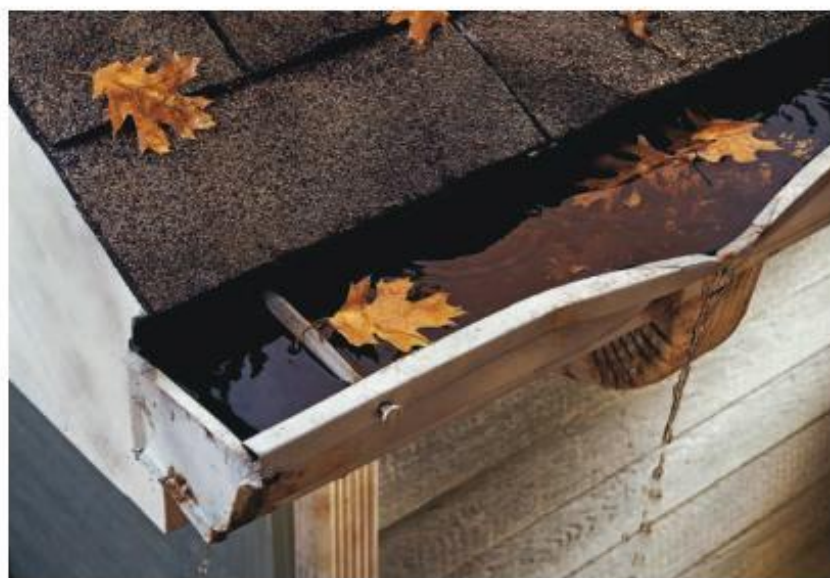
Keep gutters and downspouts clean so rain falling on the roof is directed well away from the foundation. Nearly all wet basement problems are caused by water collecting near the foundation, a situation that can frequently be traced to clogged and overflowing gutters and downspouts.
