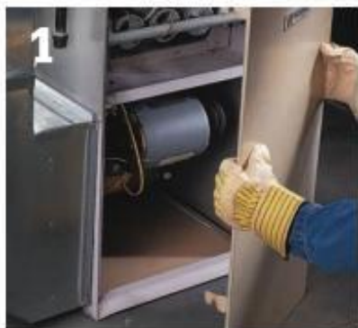
Remove the access panel to the blower housing and inspect the motor.
