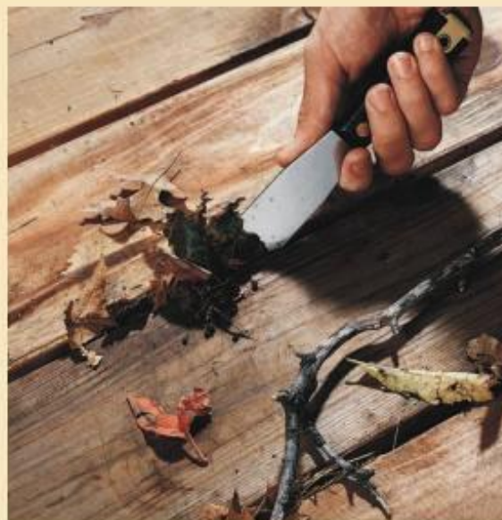
Clean debris from cracks between decking boards with a putty knife. Debris traps moisture, and can cause wood to rot.
