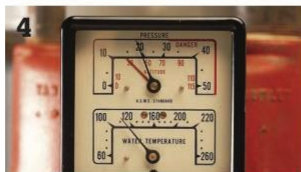
4 The boiler should reach a pressure of 20 psi before you turn the power back on.
