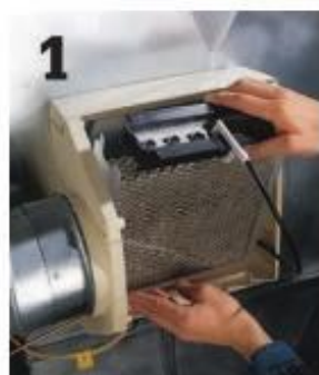
1 Remove the distribution tray from the humidifier.
