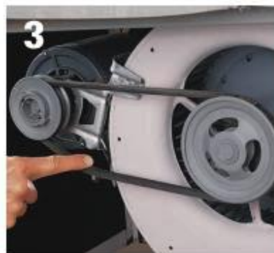
Check the tension by pushing down on the middle of the belt.
