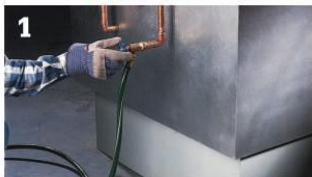
1 Use a garden hose to drain water from the boiler. Keep the drain end of the hose lower than the drain cock on the boiler.
