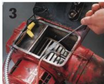
3 The blades on most blower fans are thin and hard to reach, so use a long brush carefully: a bent fan blade makes much more noise than a dirty one.
