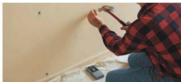
Locate framing members using a stud finder or by knocking on the wall and feeling for solid points. Verify the findings by driving finish nails through the wall surface. After finding the center of one stud, measure over 16" to locate neighboring studs.
