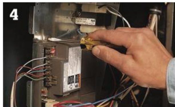
4 Unscrew the control center's mounting screws and install the replacement unit.
