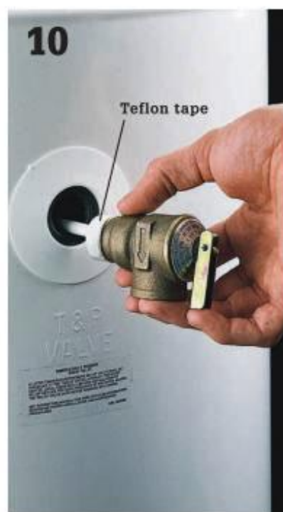
Wrap threads of new pressure-relief valve with Teflon tape, and screw valve into tank opening with a pipe wrench.
