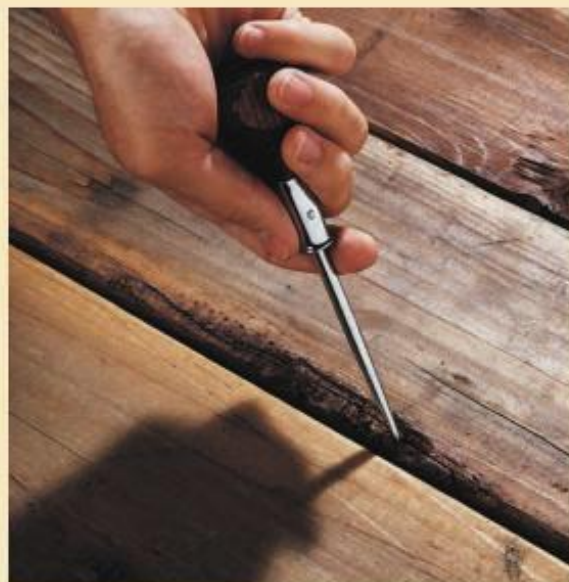
Use an awl or screwdriver to check deck for soft, rotted wood. Replace or reinforce damaged wood.
