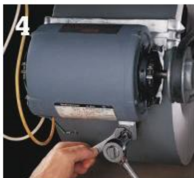
Loosen the pulley tension adjustment nut slightly to tighten the belt.
