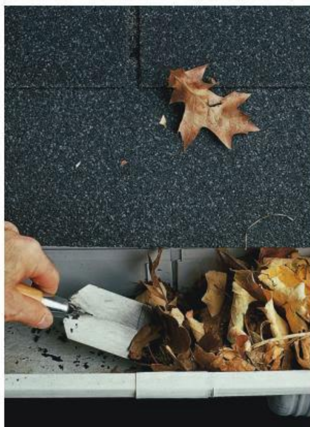
Use a trowel to clean leaves, twigs, and other debris out of the gutters before starting the repairs.
