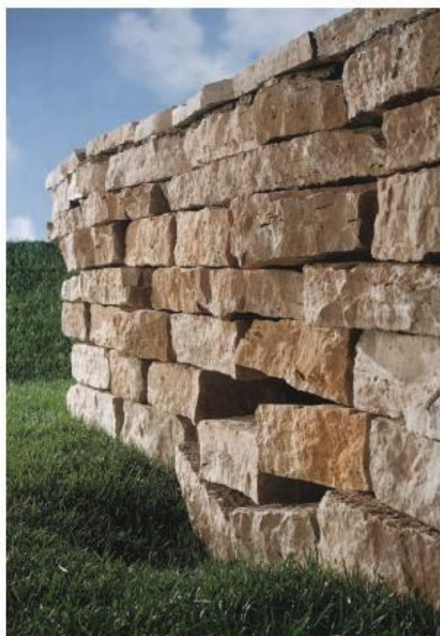
Stones in a wall can become dislodged due to soil settling, erosion, or seasonal freeze-thaw cycles. Make the necessary repairs before the problem migrates to other areas.
