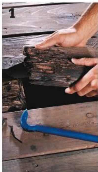
1 Remove nails or screws from the damaged decking board, using a cat's paw or screwgun. Remove the damaged board.
