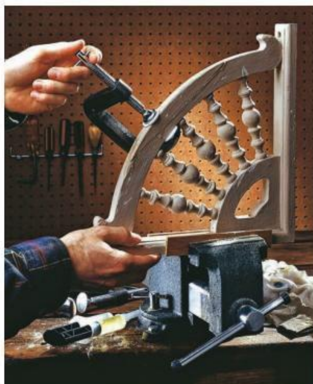
Repair delicate or ornamental trim molding in your workshop, whenever possible. You'll get better results than if you try repairing it while it's still attached.
