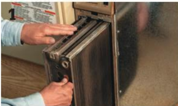
Clean electronic filters every month , then reinsert them in your furnace.
