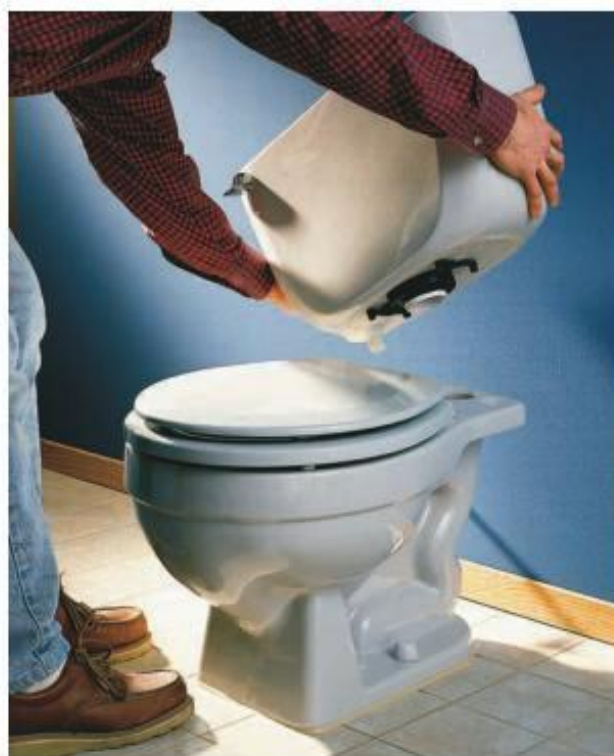
Install a toilet by anchoring the bowl to the floor first, then mounting the tank onto the bowl. China fixtures crack easily, so use care when handling them.
