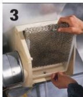
3 Remove the evaporator pad from the frame.
