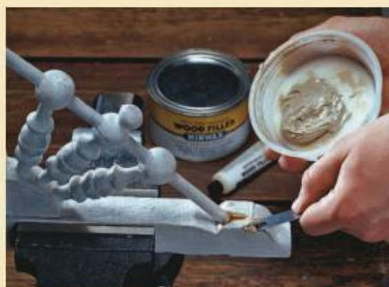
Repair decorative trim molding with epoxy glue or wood filler. For major repairs, make your own replacement parts, or take the trim to a custom millwork shop.
