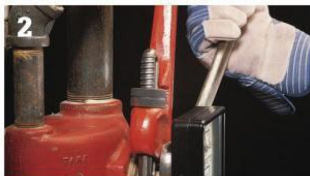
2 If the valve or gauge on top of the boiler is attached to a separate fitting, hold the fitting still with one wrench while removing the valve or gauge with another.
