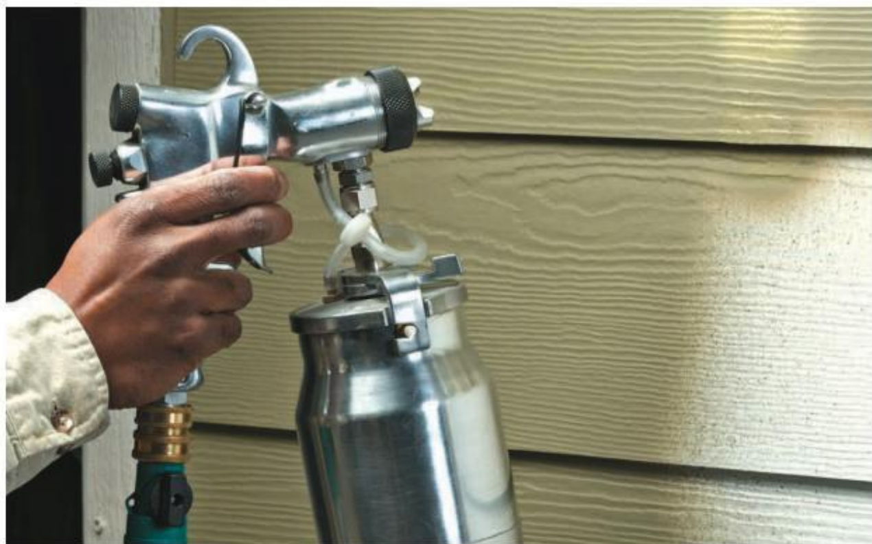
Paint sprayers allow you to cover large areas of siding and trim in a short amount of time. They also make it easier to paint areas that are hard to reach with a brush or roller.
