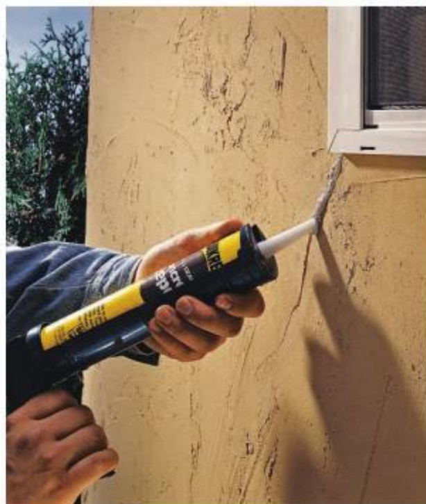
Fill thin cracks in stucco walls with masonry caulk.
