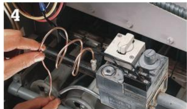
4 Remove the thermocouple from the control housing and install a new one.
