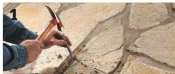
Chisel out the mortar around the damaged stone, being careful not to strike surrounding stones.
