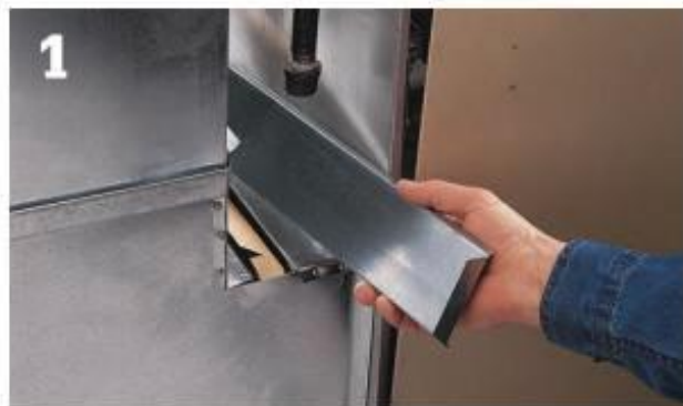
Many filters are located between the return air duct and the blower, and rest in a slot or bracket.
