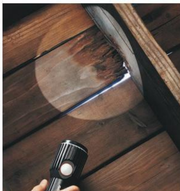
Inspect hidden areas regularly for signs of rotted or damaged wood. Apply a fresh coat of finish yearly.
