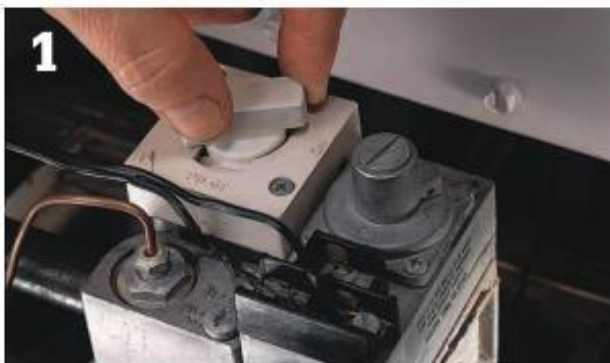
1 Turn off the main gas supply and the pilot gas supply (if your furnace has a separate one).
