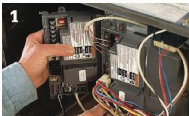
1 Remove the control center wires one at a time and switch them over to the new control center.
