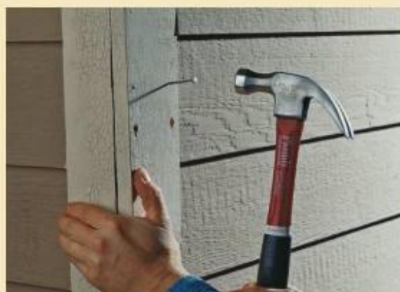
Reattach loose trim with new ring-shank siding nails driven near old nail locations. Fill old nail holes with paintable caulk, and touch up caulk and new nail heads with paint to match the surrounding surface.
