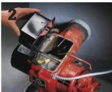
2 If the transformer attaches to the blower housing with a hinge, simply swing it out of the way. If it comes loose, be careful not to strain the wire connections.
