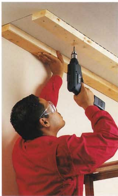
A. Position each plate, check to make sure they are level, and attach them to the ceiling with 3" screws driven into the joists or blocking.
