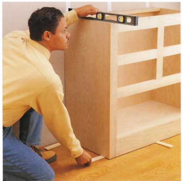
C. Check the cabinet for level, shimming under it if necessary. When the cabinet is in position, toenail the side panels at the shim locations.
