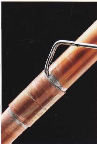
E. Push \frac{1}{2} " to \frac{3}{4} " of solder into each joint, allowing capillary action to draw the liquefied solder into the joint.
