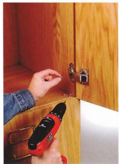
F. Hang the cabinet door with concealed hinges. Adjust the door to sit precisely on the cabinet frame.
