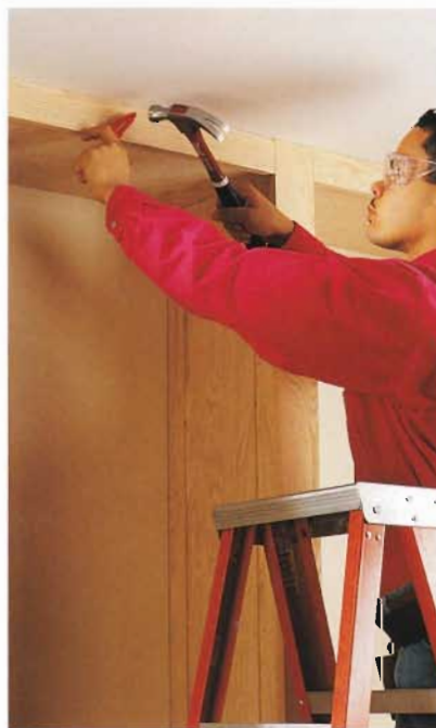
E. Measure and cut the 1 × 3 top rails to fit between the stiles. Then drill pilot holes and attach the rails to the top plate and top panels.
