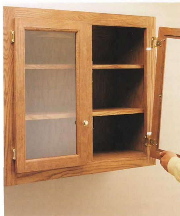
I. Install overlay doors and door hardware after the finish for the cabinet and doors is dry.
