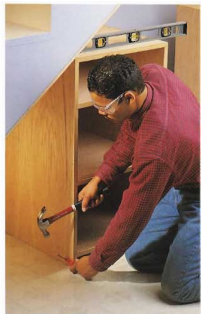
F. Check to ensure the cabinet is level. Attach it to the floor with 2" finish nails.
