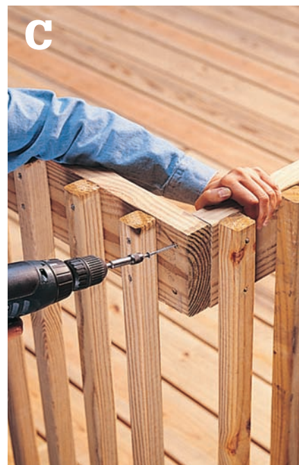
Level the 2 × 6 railing behind the 2 × 2s, then attach it by driving screws through the pilot holes.
