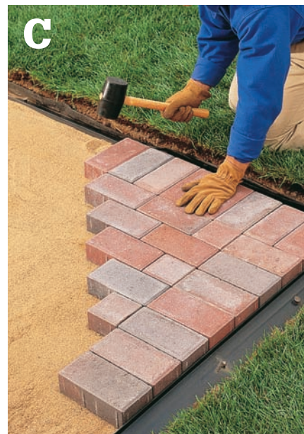
Lay border pavers in 2 ft. sections, then fill in with field pavers.
