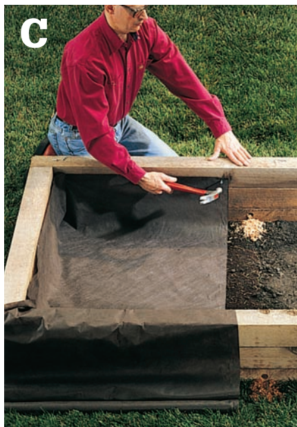
Place the third layer of landscape timbers over the second, staggering the joints. Secure the timbers in place with nails. Drill \frac{1}{2} " drainage holes through the bottom row of the timbers. Line the bed with landscape fabric.
