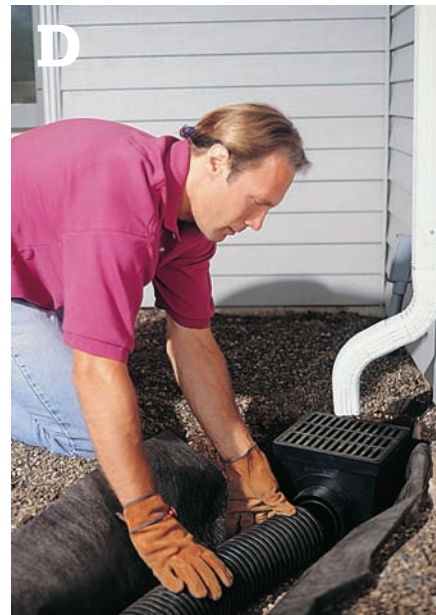
D Attach a catch basin to the drain tile opening, and position the basin to collect the excess water in the problem area.
