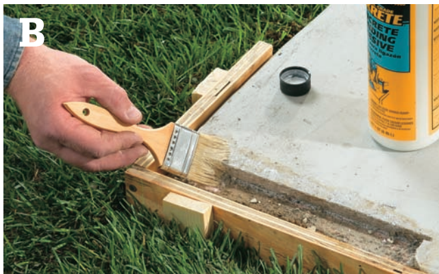
B Set the form flush with the slab surface, then apply bonding agent and patching cement.
