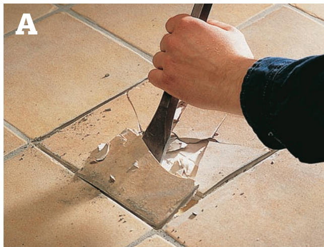
Cut out the grout , then break up and remove the damaged tile in pieces.
