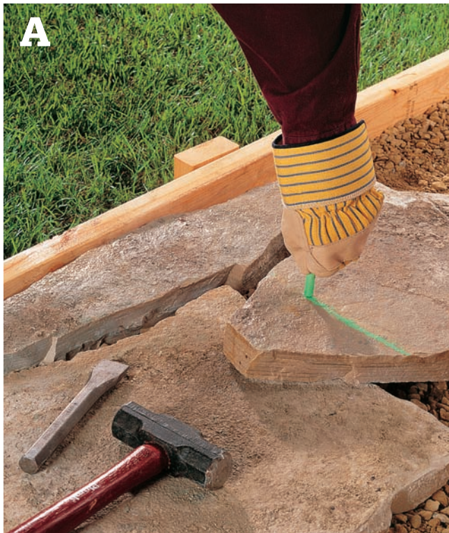
Mark a cutting line on both sides of the stone, using a crayon or chalk.
