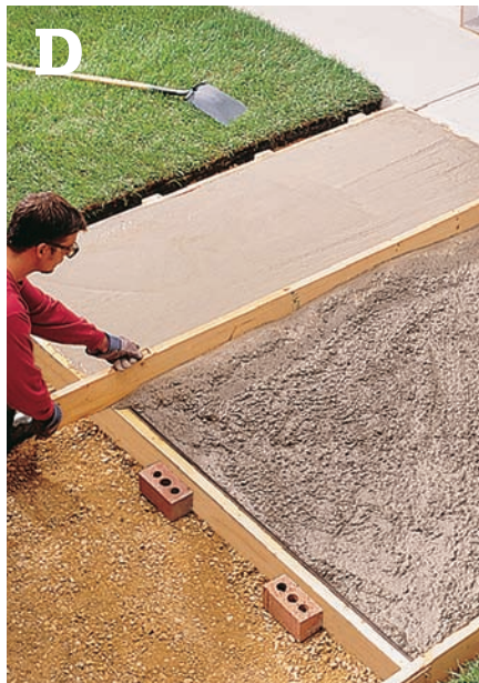
D Screed the concrete smooth, riding the screed board along the tops of the form sides.
