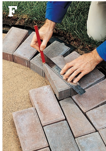
F Pave around curves, setting even gaps; fill in with cut pavers as needed.
