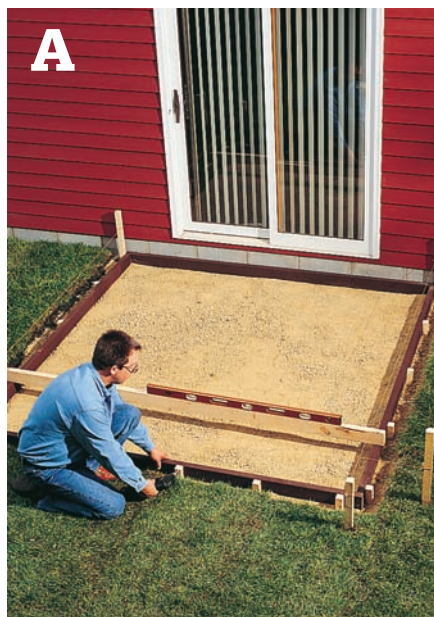
Stake the form at 2-ft. intervals, checking the form for level and slope.
