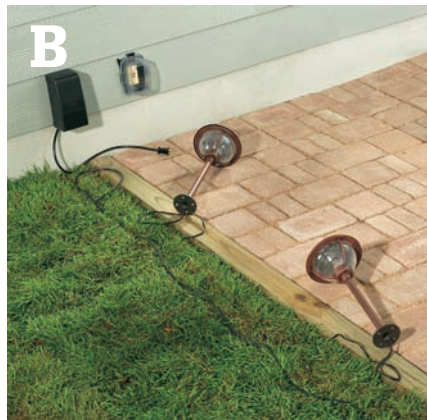
Position the cable and fixtures according to your plan, and make any necessary adjustments.
