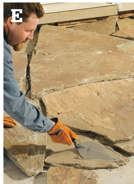
Add mortar and stones to complete the surface, checking for level as you go.
