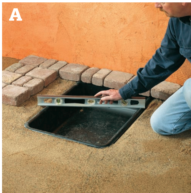
Set the reservoir basin in the hole and check for level.
