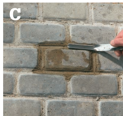
Mortar the new paver in place, then tool and smooth the mortar for a seamless repair.
