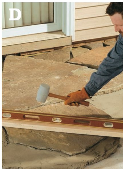
Bed the first stone into the mortar, then check it for level.
