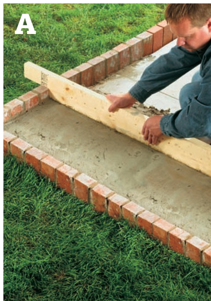
Screed the mortar bed to a consistent thickness, using a 2 × 4 screed board set on the edging. Rake the surface of the mortar with a notched trowel.
