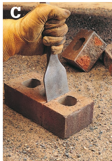
To split a brick , align a mason's chisel on a scored line. Tap the chisel with a hammer until the brick splits.
