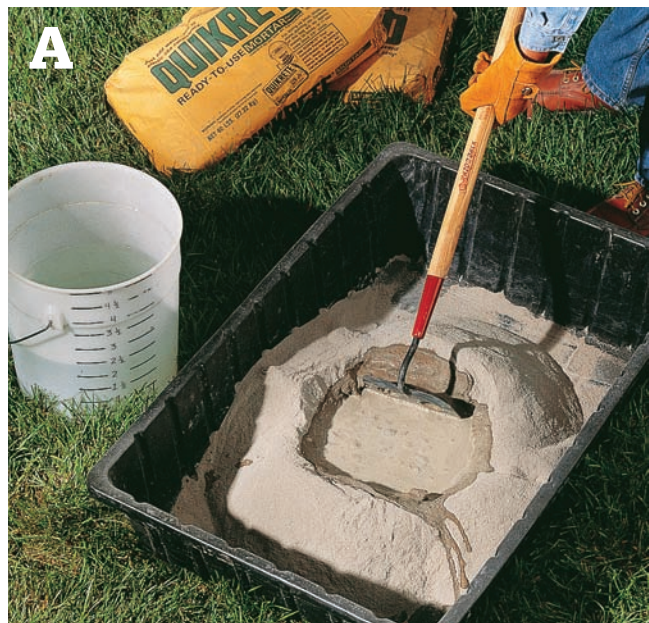
Mix the mortar with some of the water, then add more water as needed.
