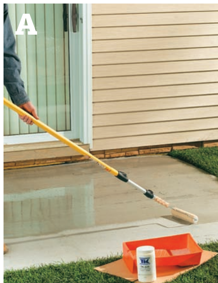
Thoroughly clean the concrete slab, then apply a concrete bonding agent.
