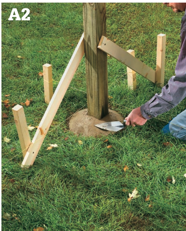
Ground Installation: Anchor the posts in concrete, overfilling the footings to create a rounded top.
