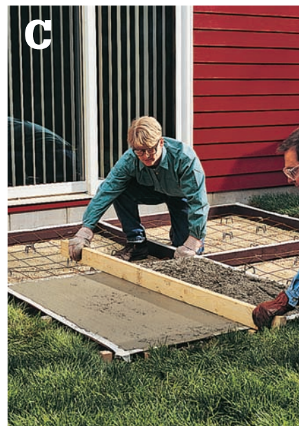
Place concrete into the first quadrant , then screed it level with the top of the form.
