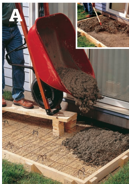
Pour concrete in evenly spaced loads (called a “pod”), starting at the end farthest from the concrete source. Use a masonry hoe to distribute concrete evenly (inset).
