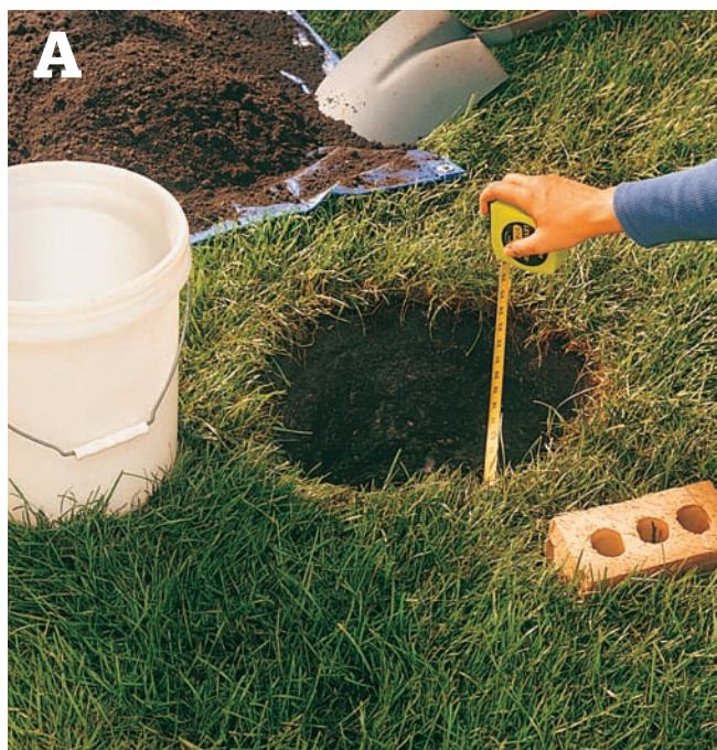
Dig a hole approximately as deep as the combined height of the basin and the paving stones plus 4".
