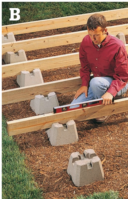
Position the remaining footings and insert the joists. Check to make sure the framework is level, and adjust as needed.
