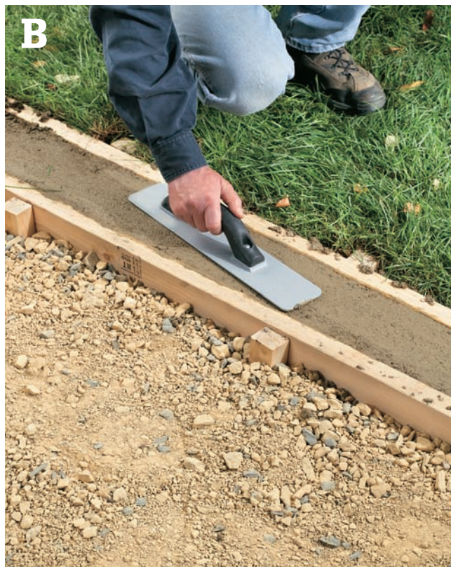
Float the top of the curb with a concrete float, and finish the surface as desired.
