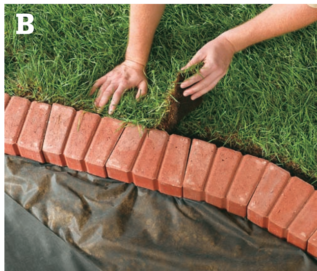
Lay sod or backfill behind edging to hide it from view.
