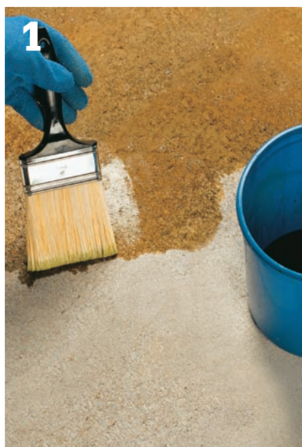
Use a paintbrush to apply stain , using long, even strokes. Minimize brush strokes.
