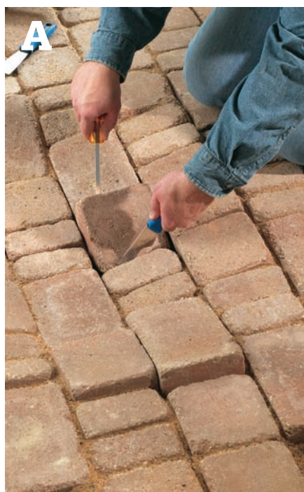
Pry up the first paver , being careful not to damage the surrounding units.
