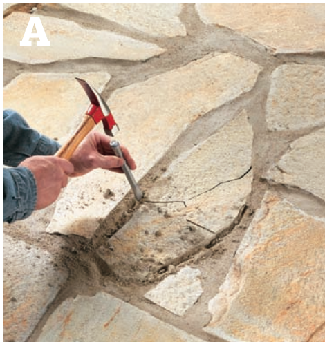
Chisel out the mortar around the damaged stone, being careful not to strike surrounding stones.
