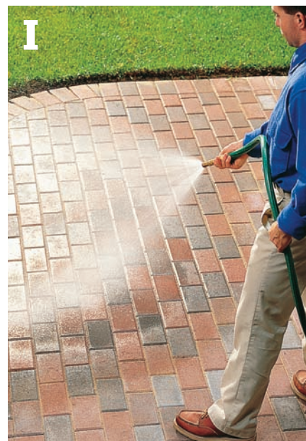
Soak the patio , then let it dry to complete each round of packing the joints.
