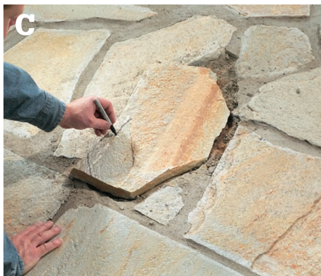
Mark the replacement stone so it will fit into the cavity with the proper spacing for mortar joints.
