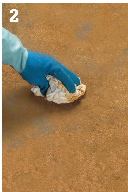
Once stain has absorbed , remove residual stain with rags.
