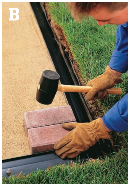
Place the first two border pavers , setting them in the sand with a rubber mallet.
