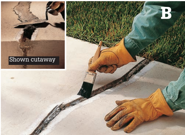
Brush inside the crack and along the surface edges with latex bonding agent.
