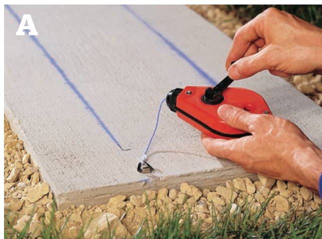
Lay out the first course of block, cutting blocks as necessary. Mark the ends and corners, then remove the blocks and snap reference lines.
