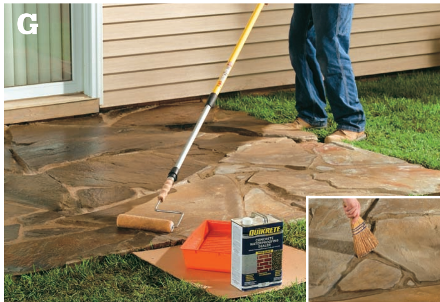
Smooth the mortar joints flush with the stone surfaces (inset), and then let the mortar cure completely. After a week, seal the stone, if desired.
