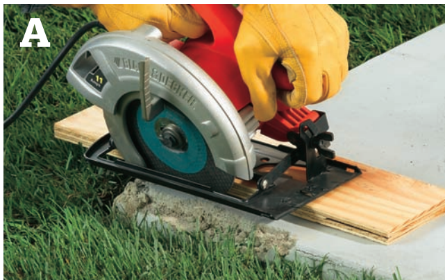
A Cut into the slab at a 15° angle to create a clean keyed edge for the patching material.
