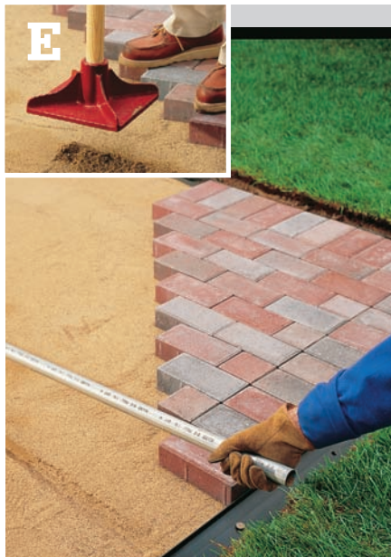
E Remove screed pipes as you near them, replacing sand and retamping the surface.
