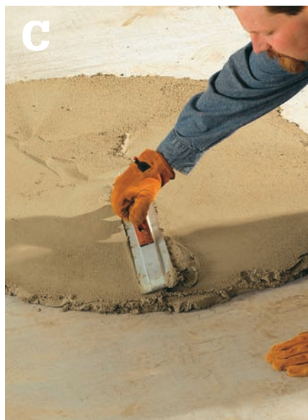
Move some of the stones aside , then apply mortar for setting the first few stones.
