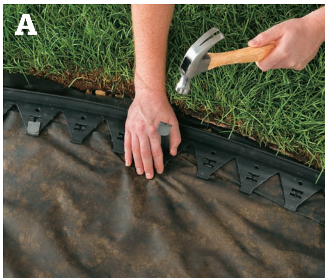
Secure the edging with spikes driven through the nailing tabs.
