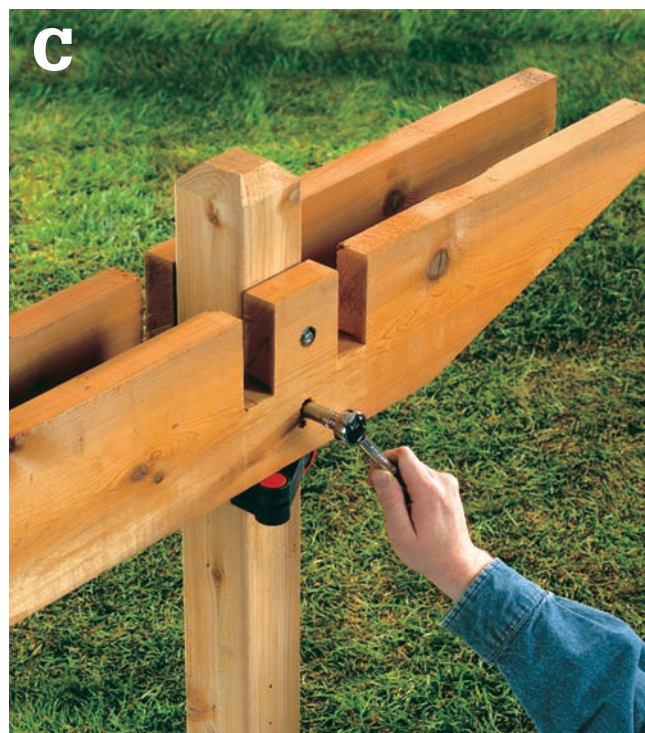
Countersinks help hide the bolt hardware. Locate them in the least conspicuous areas.
