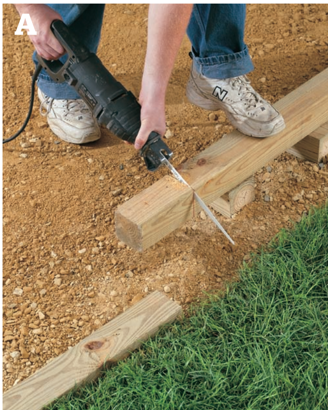
A Cut timbers to length with a reciprocating saw and long blade (or other saw).
