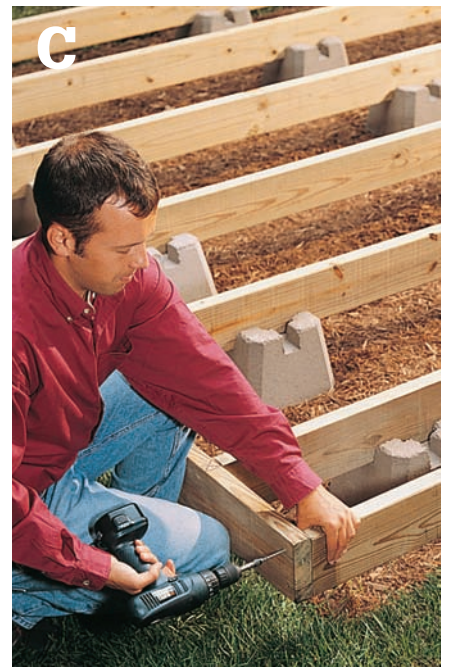
Install the front and back rim joists between the ends of the side joists, securing them with pairs of deck screws.
