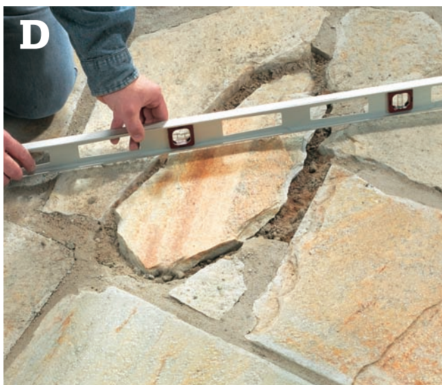
Set a straightedge across the top of the new stone to make sure it is even with the neighboring stones.
