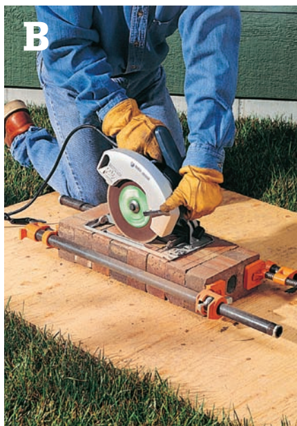
Use a circular saw with a masonry-cutting blade to score a group of bricks. Clamp the bricks, making sure the ends are aligned.
