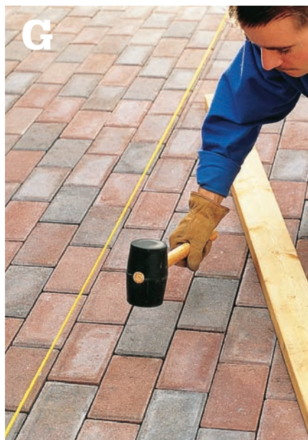
Inspect the entire installation for uneven or misaligned pavers. Using a rubber mallet, tap pavers to set them at the appropriate height.
