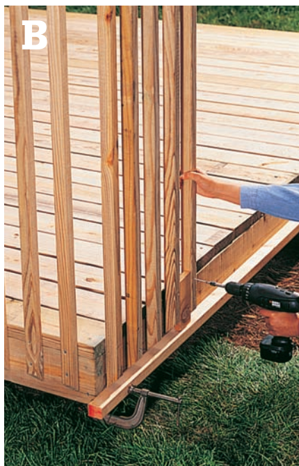
Attach the 2 × 2s to the side joists, leaving a 4" gap between them.
