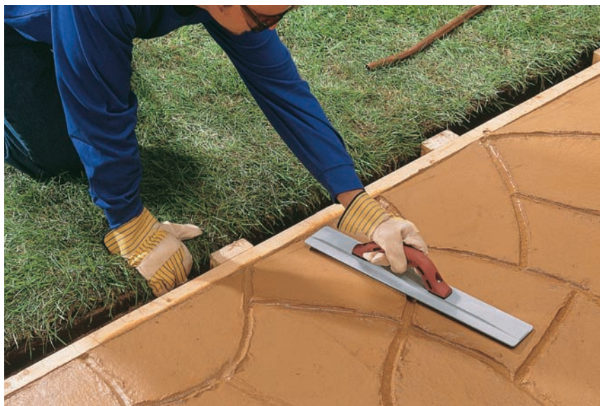
Refloat the surface for a smooth, mortared flagstone appearance.
