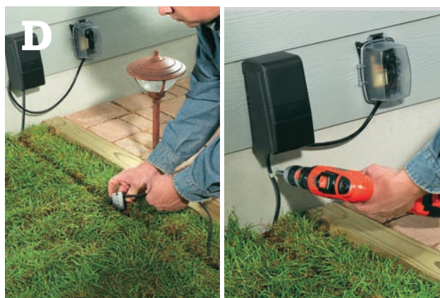
(Below) Test the system , then bury the main cable in the ground or attach it to permanent structures, as needed.
