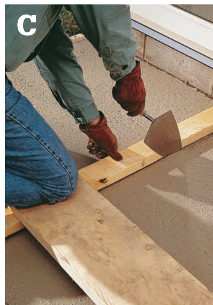
Cut control joints at marked locations with a mason's trowel, using a straight 2 × 4 as a guide.
