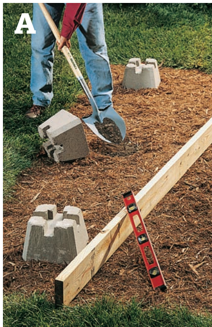
Position the corner footings and the center footing for the back joist. Remove or add soil beneath the footings to level them.
