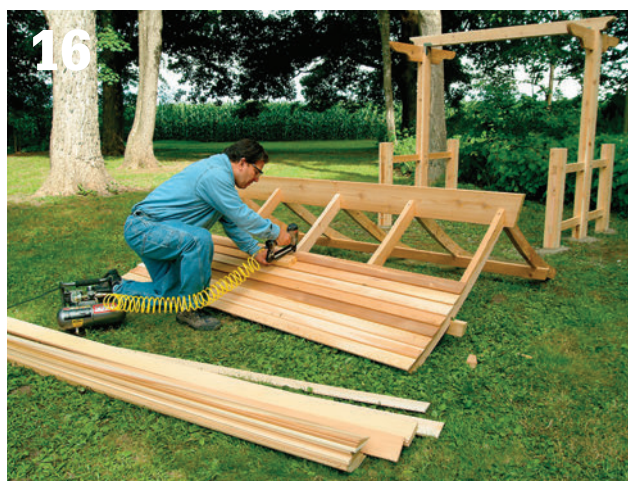
Attach the shingles (in this case, narrow cedar lap siding strips) to the rafters with 1\frac{3}{8} " narrow-crown staples. Start at the bottom and overlap to conceal the staples.
