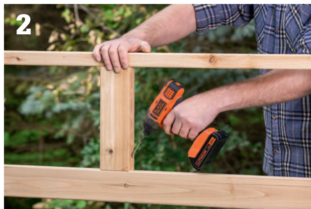
Drive deck screws toenail-style through the braces and into the seat supports
