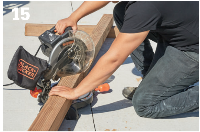
Remove the corbel stock and make the angled cuts with a power miter saw.
