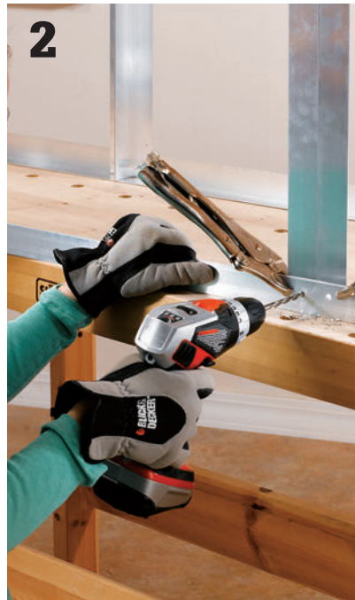
2 Drill guide holes for bolts. Clamp the part for each joint together with locking pliers and then drill for one \frac{1}{4} " bolt per joint.
