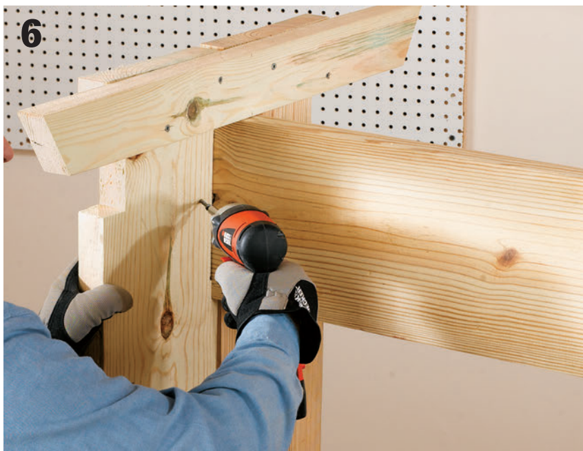
Secure the middle stretcher to the leg assemblies. Attach the second inner leg to the cross support and toe-screw this leg into the middle stretcher.
