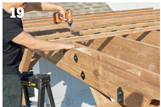
Attach the purlins to the rafter tops with exterior screws driven from above.
