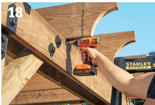
Install the remaining rafters , using L-brackets to reinforce the joints.
