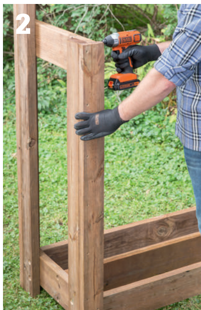
Attach the end rails between the front and rear corner posts.
