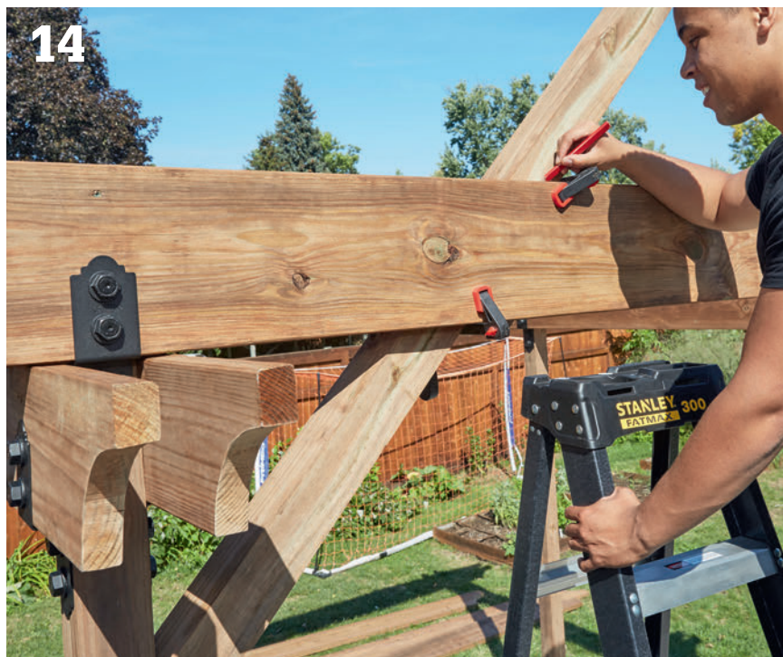
Clamp 4 x 4 stock across the corbel locations at each corner and transfer cutting lines where they cross the rafter tops.
