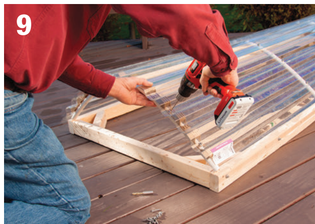
Cut closure strips to fit at each end and then drive the screws to secure the ends of the panels. Screws should be driven only at troughs in the corrugated panels and should go through panel, closure strip, and rib wall at once.
