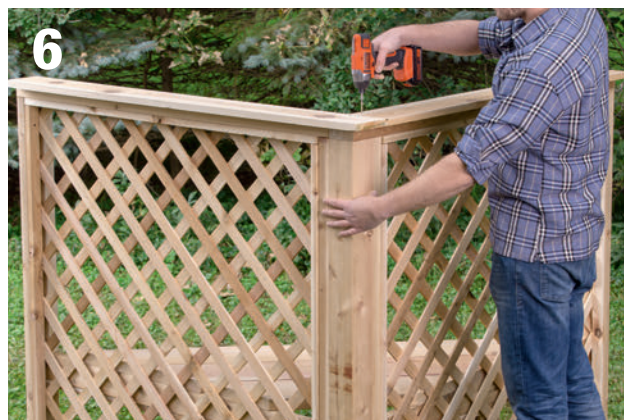
Attach the long and short caps to the tops of the trellis frames. The long cap overlaps the long rail and the post.
