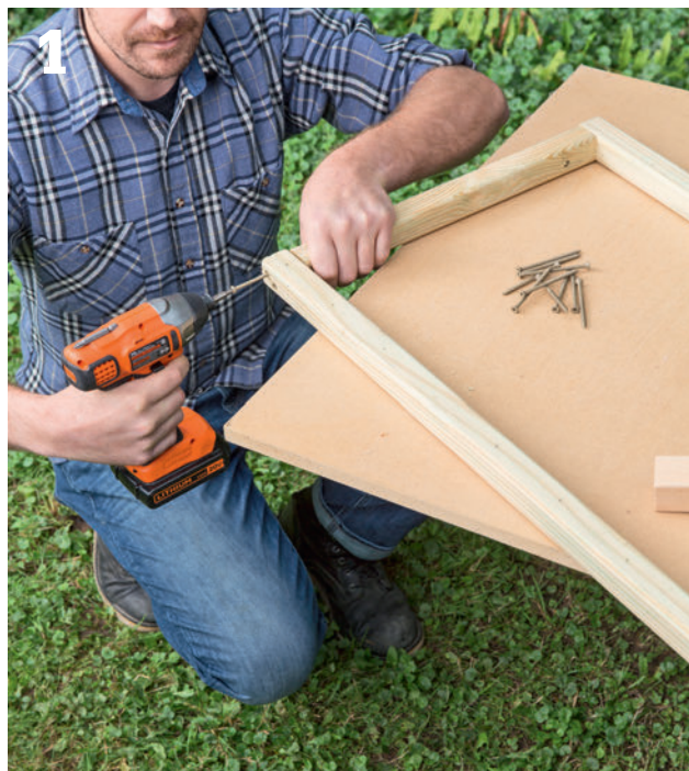
Fasten the cleats between the rails to construct the panel frames.
