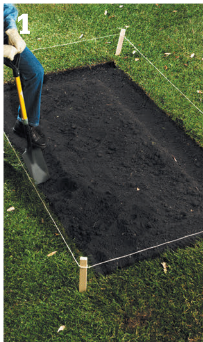
Remove the grass in the sandbox location with a flat-end spade, and then dig a trench for the first row of timbers.
