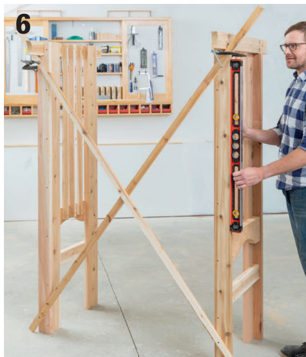
Brace the side frames in an upright, level position with long pieces of 1 × 4 while you attach the top beams.
