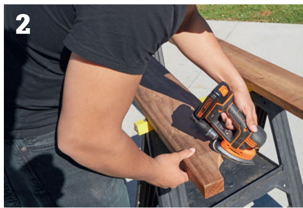
Smooth the cut end profile with a sander and break the edges of the cuts into a slight bevel to help prevent splintering.
