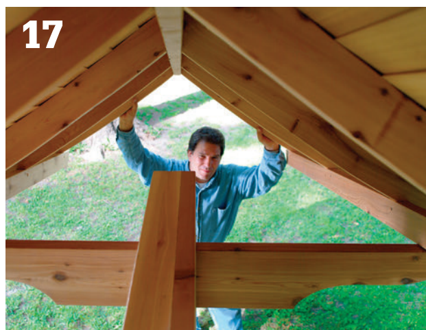
With a helper , raise the roof structure onto the post-and-beam structure, position it, and then secure it with deck screws. Reinforce the connection with rafter ties at the rafter/ridgeboard joints.
