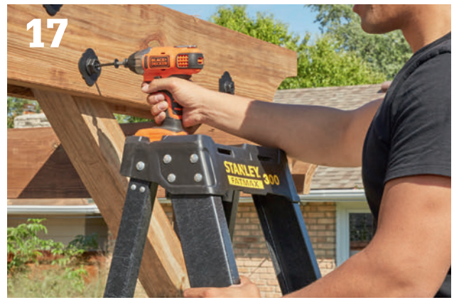
When all the corbels are cut, aligned and tacked into place, attach the final hardware.
