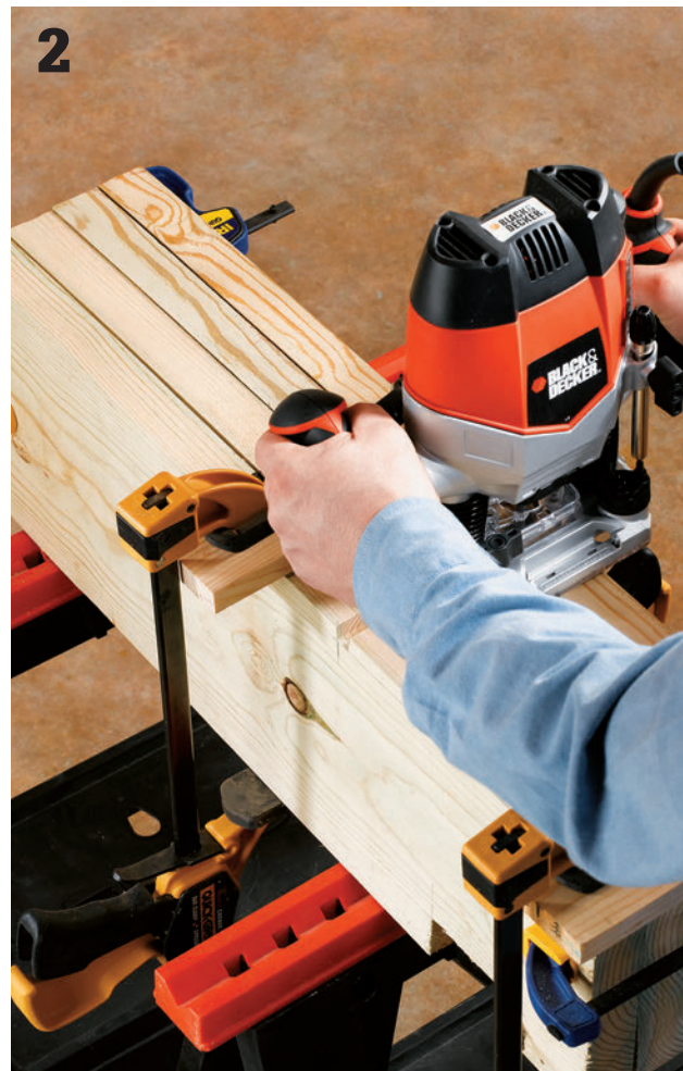
Gang-cut the stretcher notches into the legs. Clamp a straightedge guide on each side of the notch layout lines so the distance from the blocks to the notch layout line equals the router bit setback distance.
