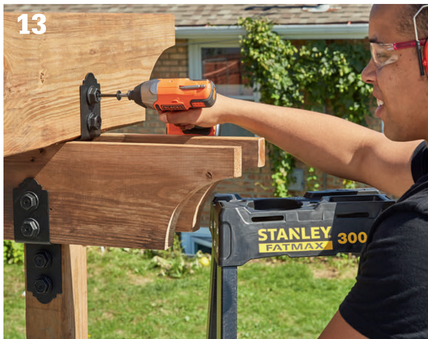
Attach the finished rafter hardware to the outer rafter at each corner.
