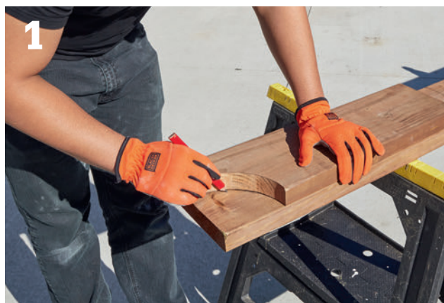
Use a cutoff piece of the correct width board for each part (the rafters are wider than the joists) and plot the end profile according to the diagram on page 180. Cut the profiles on the cutoff pieces with a jig saw to make templates.
