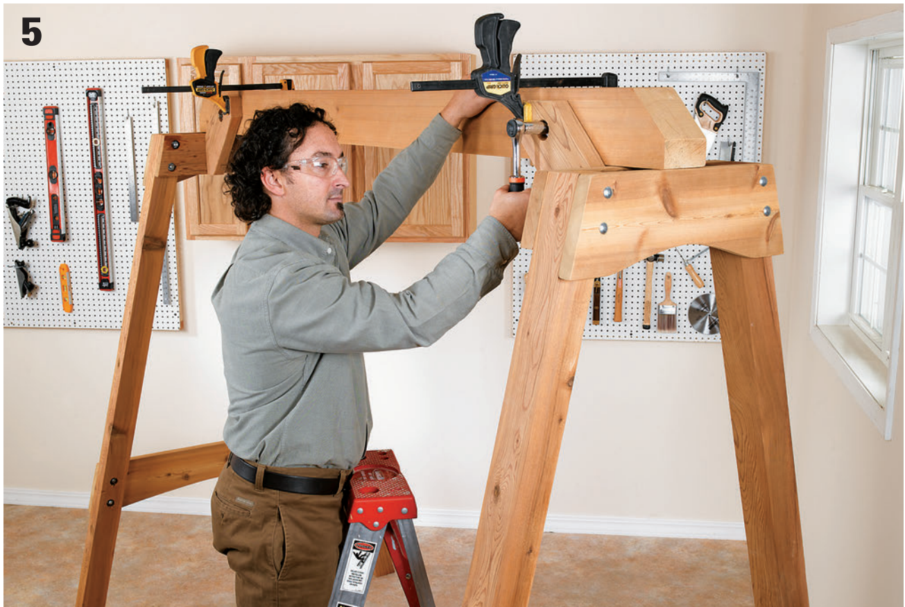
Attach the beam. Drill counterbores for washers on both gussets and drill guide holes for \frac{3}{8} "-dia. \times 6\frac{1}{2} "-long lag bolts. Insert the bolts and secure with lock washers and nuts.
