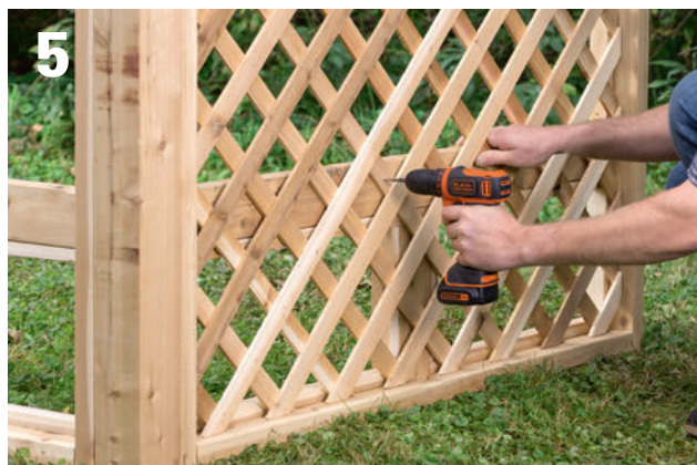
Fasten the lattice panels to the seat supports with 1¼" deck screws, then attach outer retaining strips.
