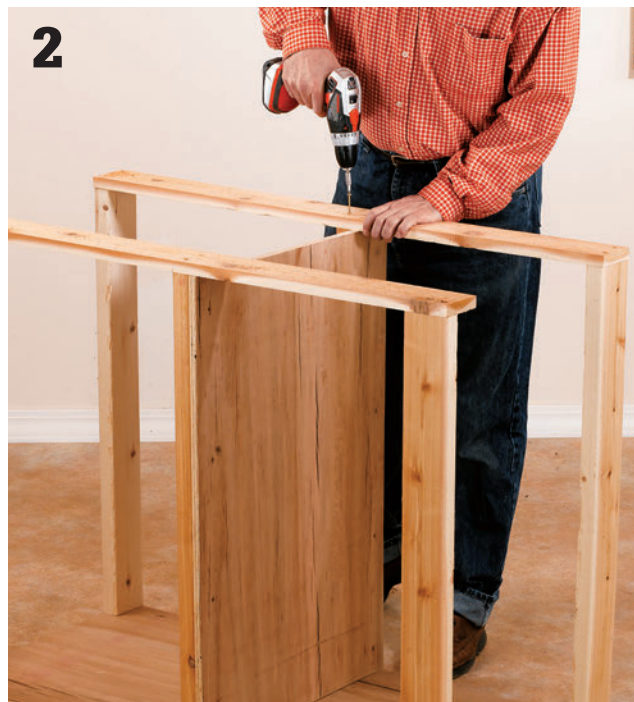
Install corner posts and top rails. Each top rail should be attached to a corner post and a center panel post with 2\frac{1}{2} " screws. Drive one screw into each post.
