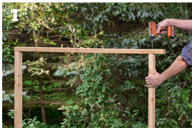
Attach the long rail at the top of one trellis frame with a 3\frac{1}{2} " overhang at one end to cover the post
