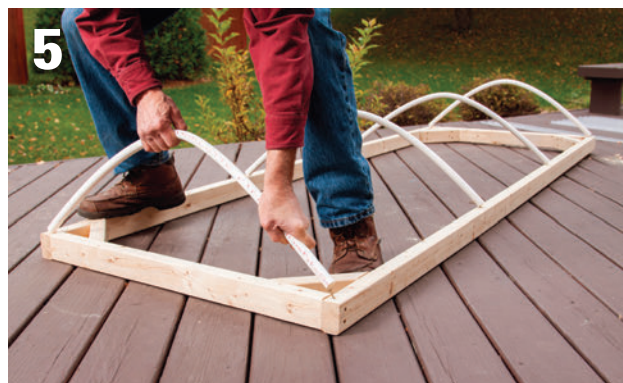
Flex the PVC tubing to both ends fit over opposite screws. The tubing should snap back to create tension that holds it in place.
