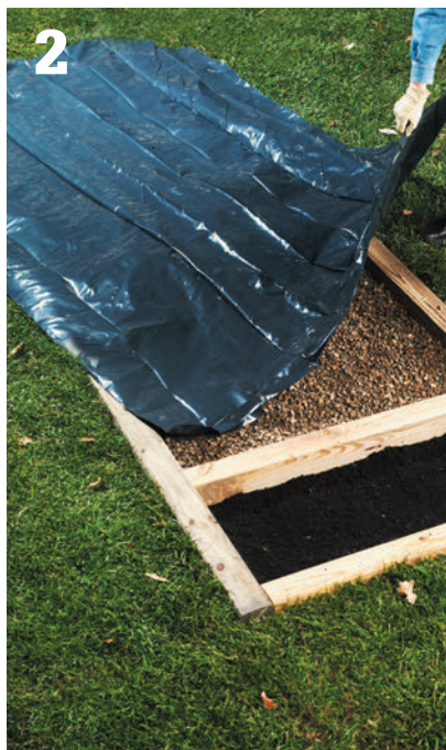
Prepare the base. Lay the first row of timbers, including the wall for the storage box. Fill the sandbox area with a 2" layer of gravel, and cover with plastic sheet or weed blocker.
