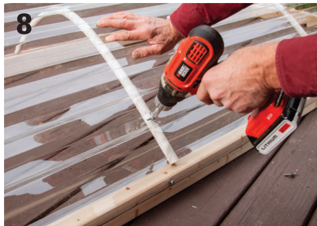
Drive the next course of screws through guide holes in the panel and into pilot holes in the PVC ribs.
