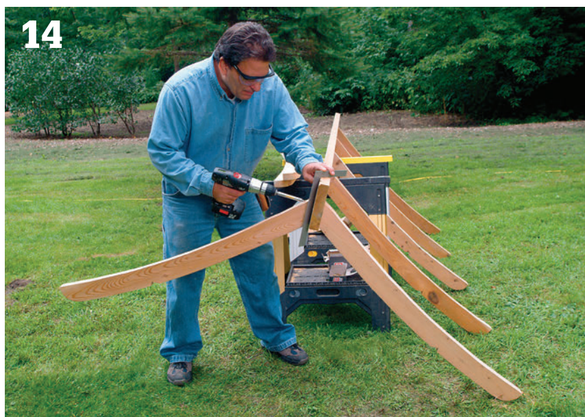
Attach the rafters to the ridgeboard with deck screws driven into pilot holes. The bottoms of the rafters should be flush with the bottom of the ridgeboard.
