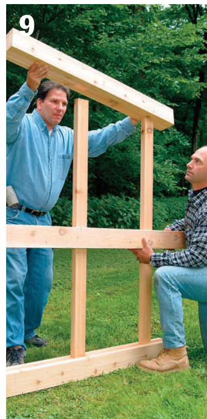
Join the main posts to pairs of outrigger posts by inserting the rails through the mortises. Center the main post on the rails. Pin joints temporarily with deck screws. (Do not glue them.)
