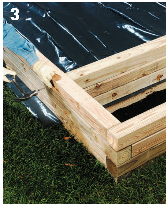
Build the rest of the sandbox frame, staggering the corner joints. Drill holes and drive barn nails through the holes.
