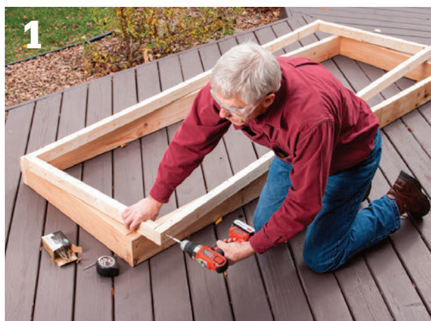
Assemble the box frames with simple butt joints. The base frame and the canopy frame are rectangles of the same dimensions.
