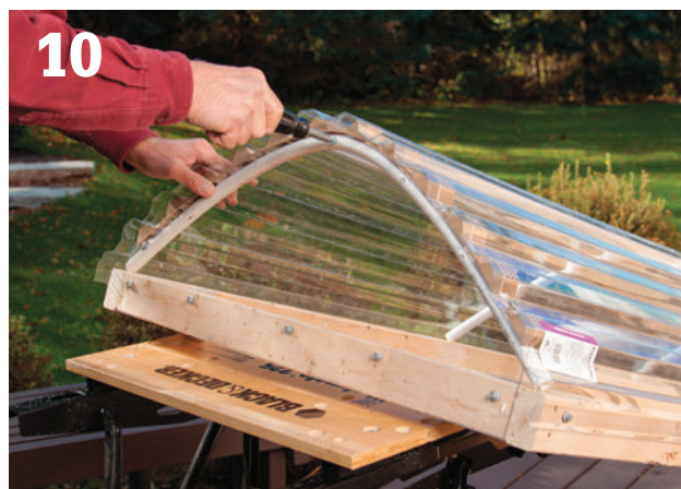
Attach the acrylic end panels to the canopy frame. Carefully drill guide holes in the acrylic sheeting before driving screws. Use a hand screwdriver to ensure that you do not overdrive the screws and crack the acrylic.
