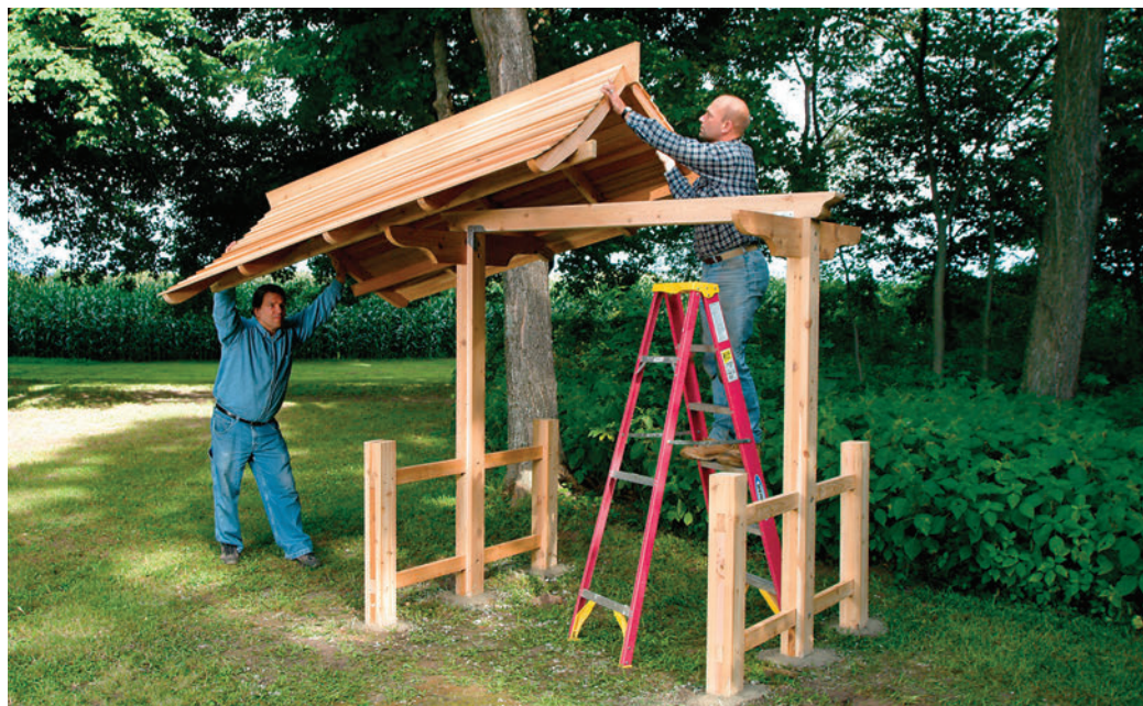
With a helper , raise the roof structure onto the post-and-beam structure, position it, and then secure it with deck screws. Reinforce the connection with rafter ties at the rafter/ridgeboard joints.
