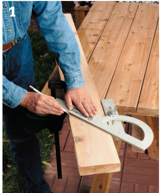
Use a saw protractor to mark a 50° angle on the end of the table leg, and then cut the angle using a circular saw.
