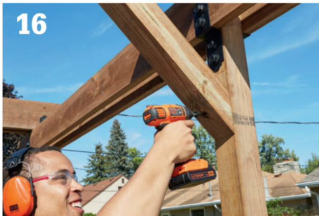
Make the angled cuts where the corbels meet the posts and then tack into position with deck screws.
