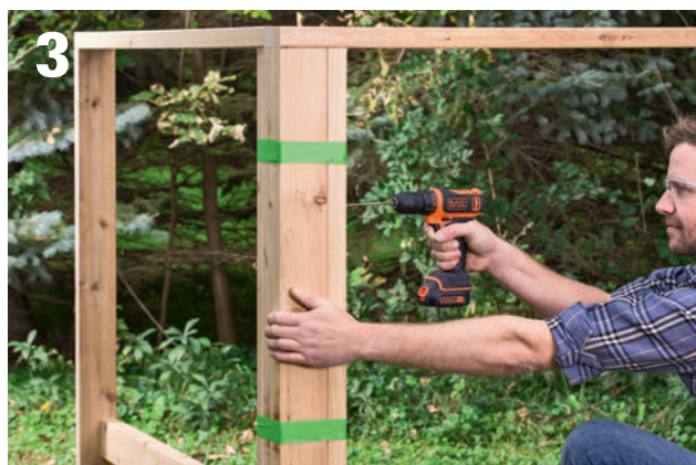
Fasten the trellis frames to the post at right angles
