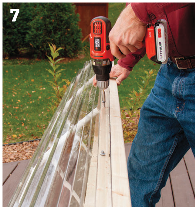
Secure the lower edge of one of the corrugated roofing panels to the base frame. Use self-sealing roofing screws (they have an EPDM rubber gasket).
