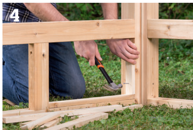
Nail 1 × 2 retaining strips for the lattice panels to the inside faces of the trellis frames.
