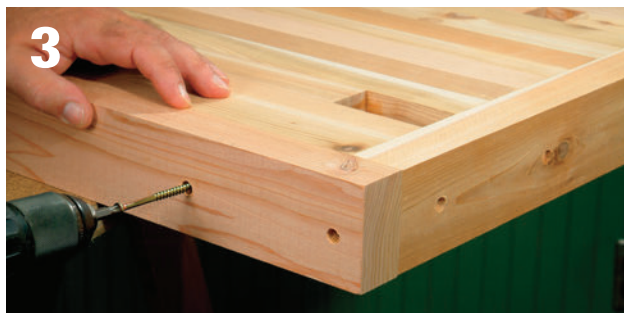
Attach the front and side seat frames with glue and counterbored deck screws. Cut plugs to fit the counterbores when the swing is completed.
