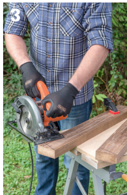
Miter-cut the middle supports and roof supports with a circular saw or with a power miter saw.
