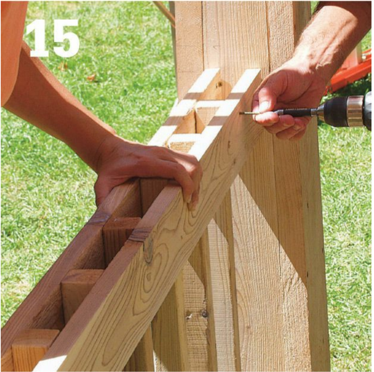
Attach the spindles to the inside of the first side rail. Attach the second side rail when the railing is in place.
