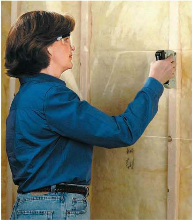
A water barrier of 4-mil plastic sheeting can be stapled to studs before installing cementboard or fiber-cement board.
