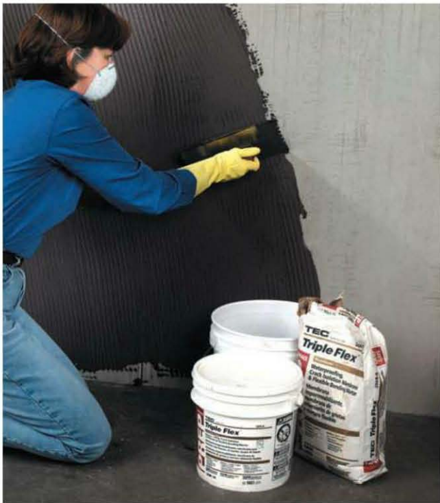
Waterproofing/isolation membranes are an easy way to add waterproofing and crack protection to existing walls. This application is especially suited to smooth, solid concrete surfaces. The tile adhesive is applied directly to the membrane after it dries.
