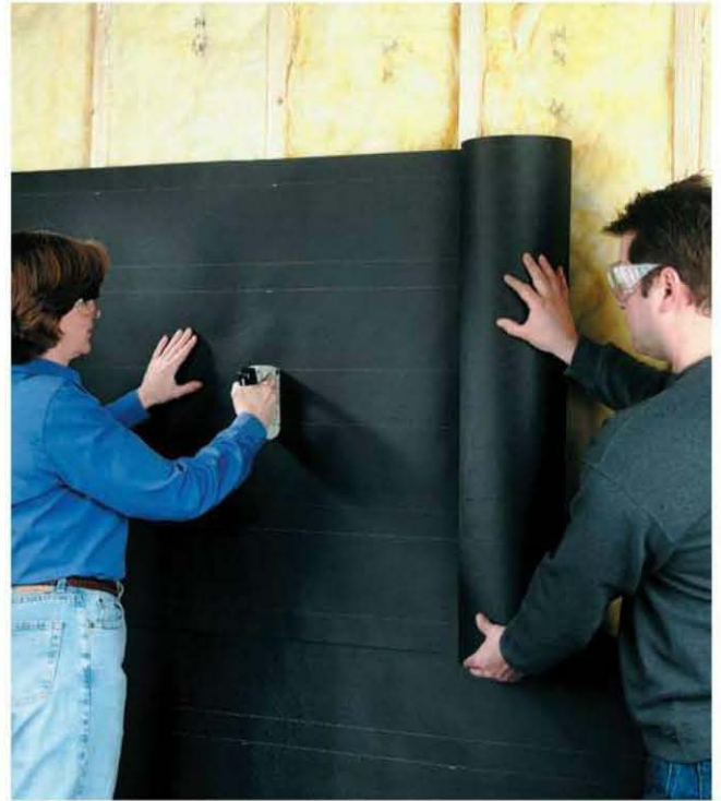
Building paper (15#) can also be used as a water barrier behind cementboard and fiber-cement board. Start from the bottom and install horizontally so each layer overlaps the previous one by two inches.
