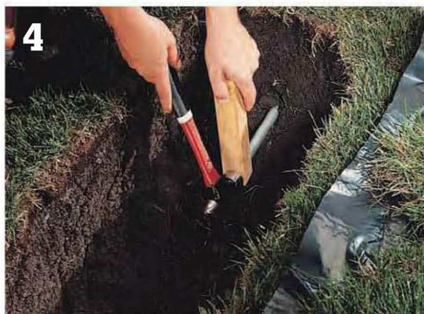
Drive conduit beneath sidewalks and other obstacles , using a block of wood and a hammer.
