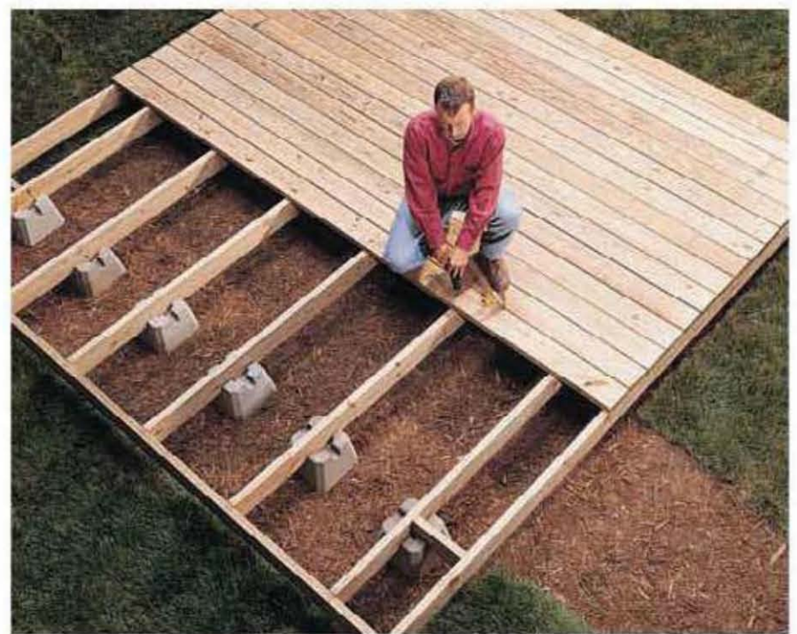
Install the decking by driving a pair of screws into each joist. Use a framing square to leave a 1/8" space between boards.
