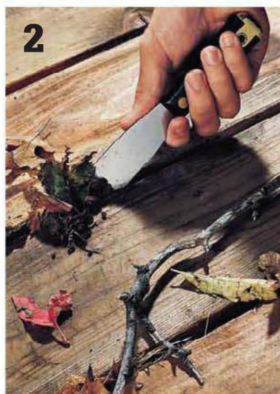
Clean debris from cracks between decking boards with a putty knife. Debris traps moisture and can cause wood to rot.
