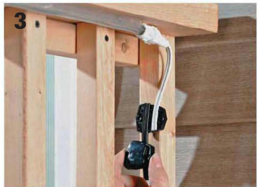
Connect the rope wires to the branch cable with a cable connector designed for outdoor cable.
