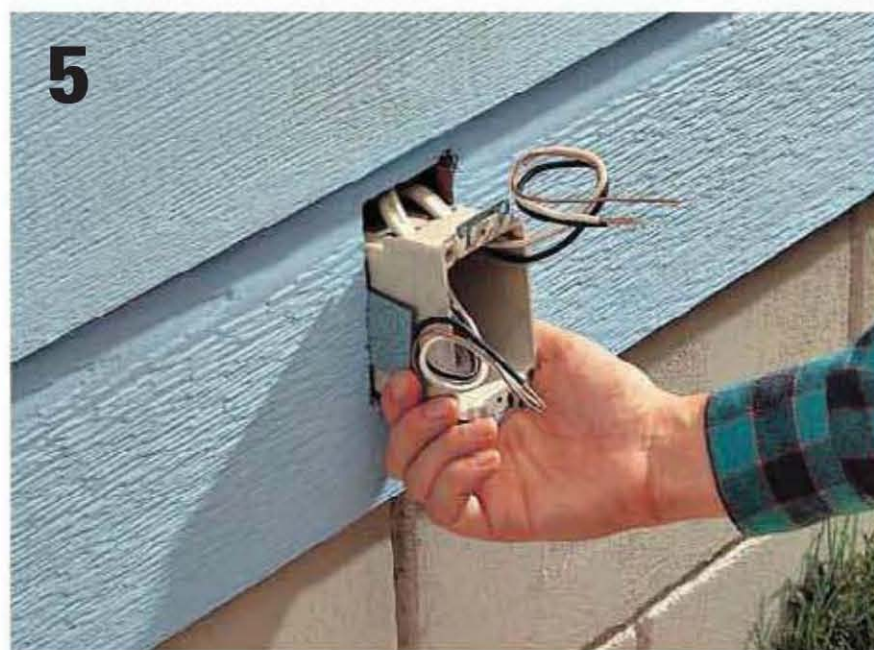
Route cables into the GFCI box , push the box into the cutout, then tighten the mounting screws until the box is secure.
