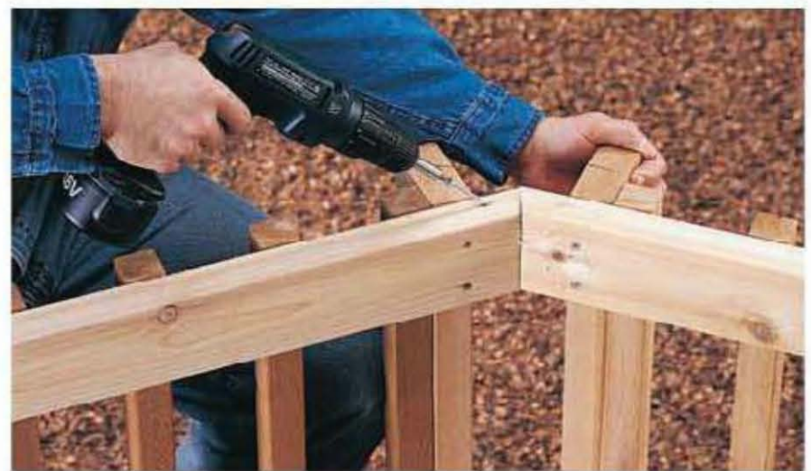
Drill \frac{1}{8} " pilot holes , then screw the top rail sections together where they meet at the corners.
