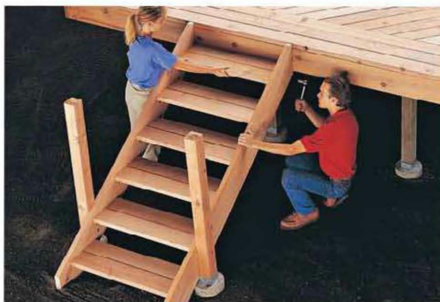
Fasten the stair to the deck with a ratchet wrench, using 4" lag screws.
