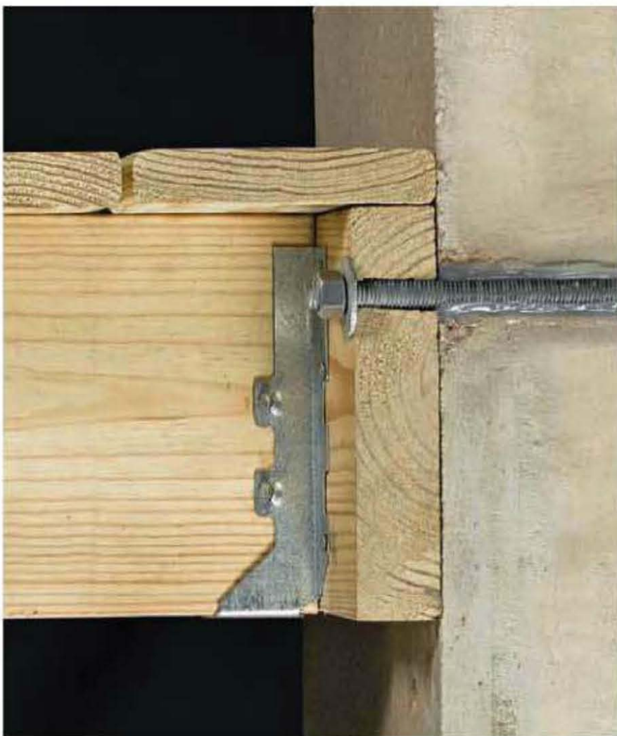
A bolt driven through the foundation from the inside can be fitted with a washer and bolt to secure the ledger.
