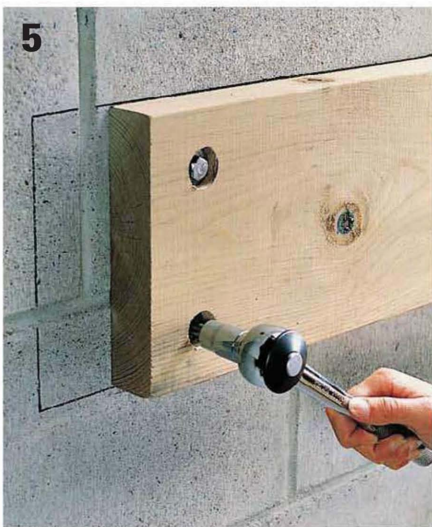
Attach ledger to wall with \frac{3}{8} \times 4 " lag screws and washers, using a ratchet wrench or impact driver. Tighten screws firmly, but do not overtighten.
