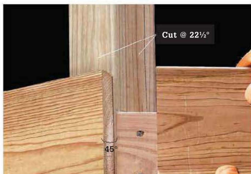
Cut 45°-miters at the ends of rim joists that meet posts at a 45° corner. Cut 22½°-miters at the ends of face boards that meet at a 45° corner.
