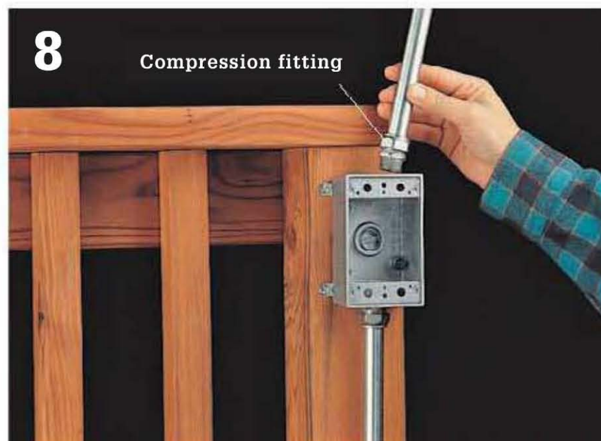
Attach conduit to the switch box so it extends from the box to the deck light location, using a compression fitting.
