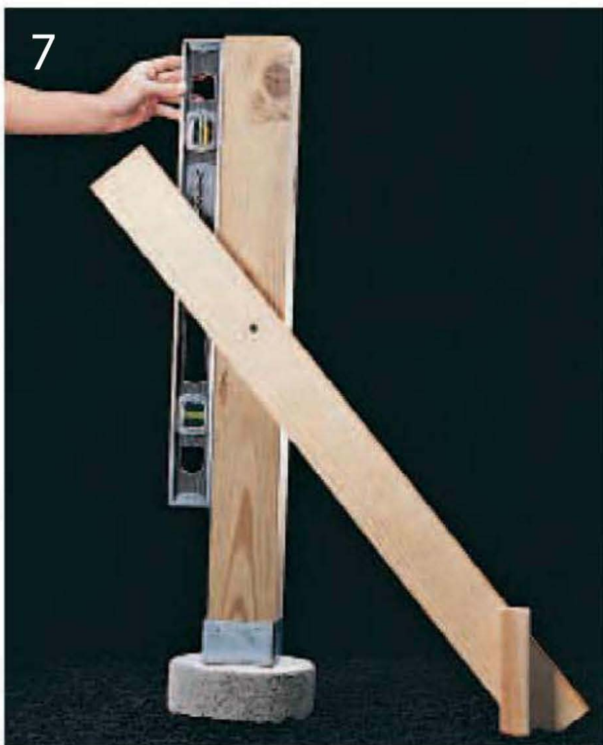
7 Use a level to make sure the post is plumb. Adjust the post, if necessary.
