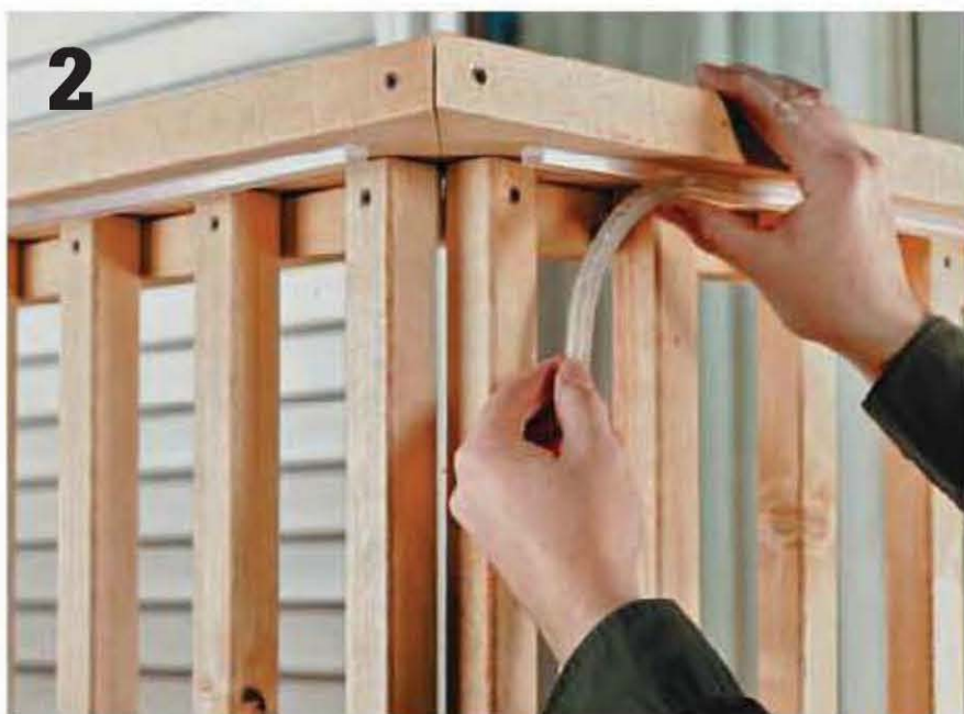
Fasten U channel to the bottom of the railing, then press the rope light in the channel securely.
