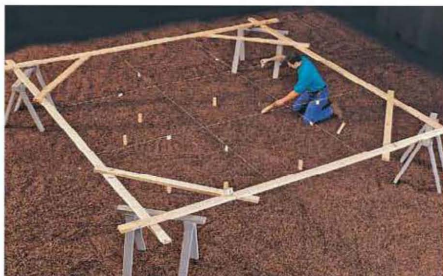
Locate the deck footings by stretching mason's strings across the site chooser, marking footing locations with tape, and dropping a plumb bob from each mark.
