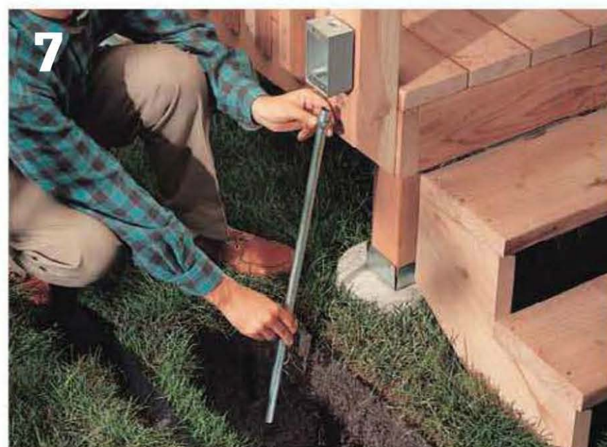
At the deck, attach conduit to the receptacle box so it extends from the bottom of the box to 4" from the bottom of the trench.
