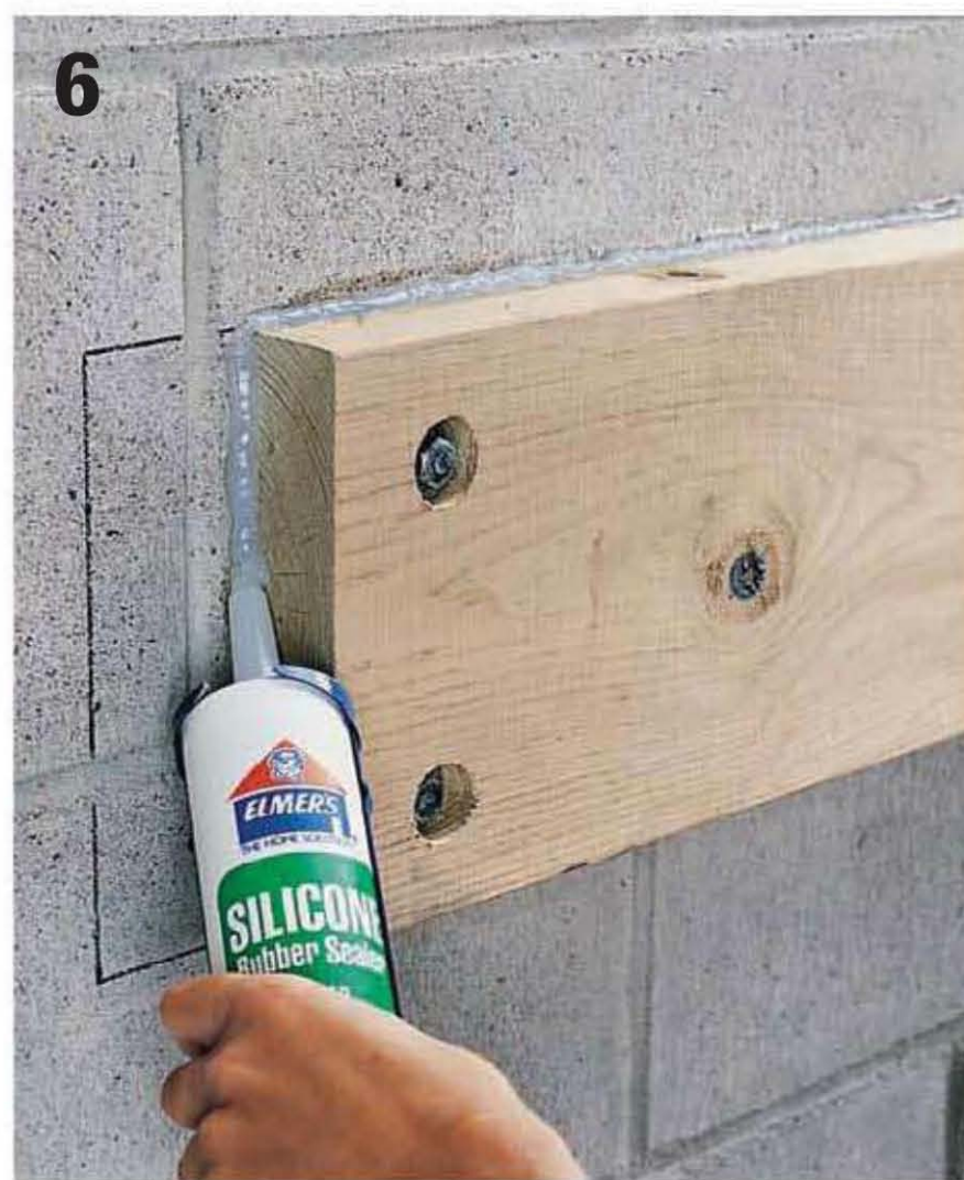
Seal the cracks between the wall and ledger with silicone caulk. Also seal the lag screw heads.
