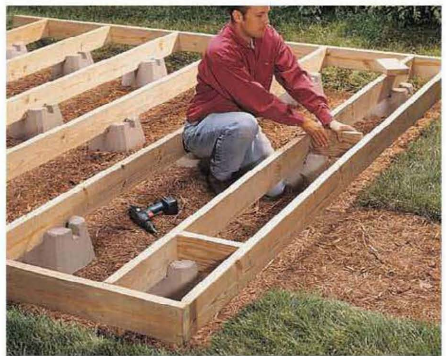
Position the sleepers in the slots of the footings , then attach them to both joists with pairs of deck screws.
