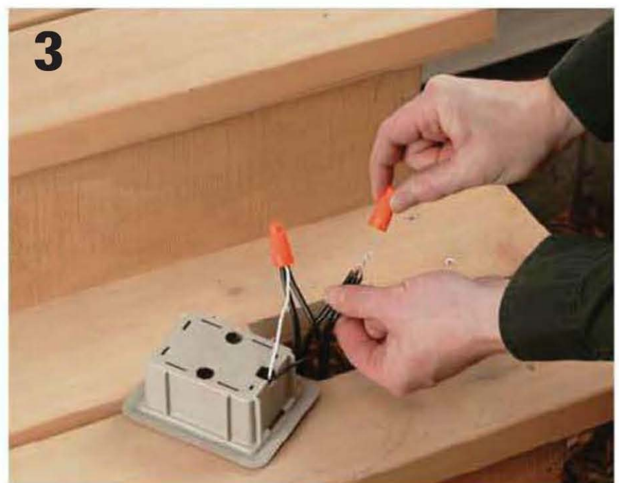
Join the lead wires of the fixture with the wires of the low-voltage cable using outdoor wire connectors.
