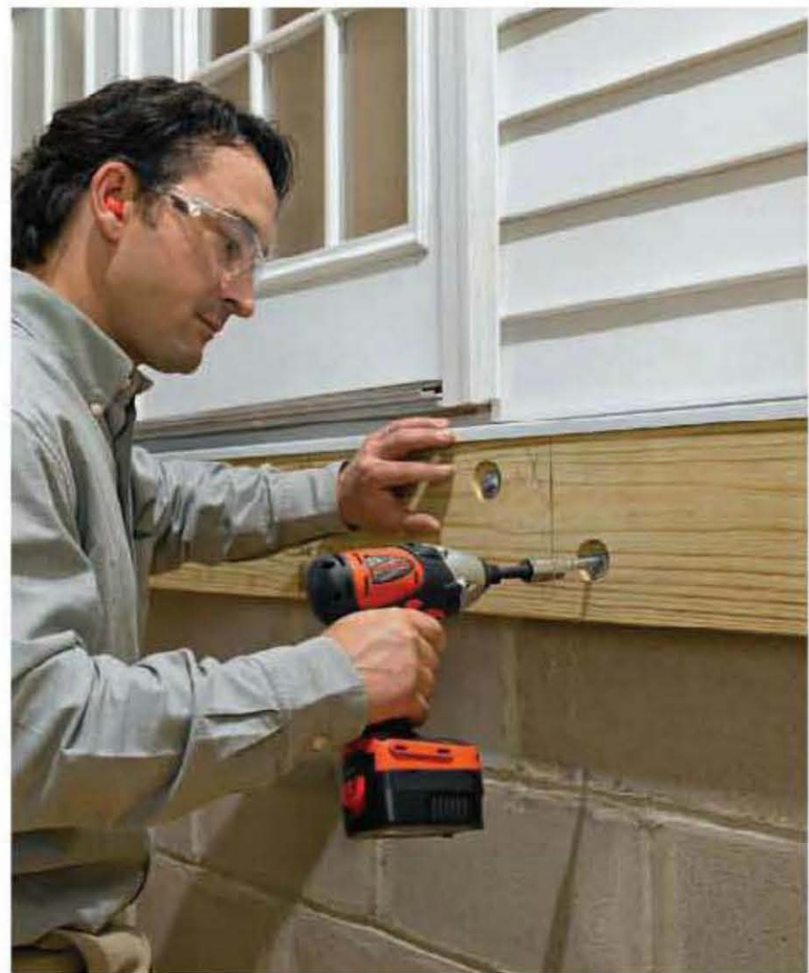
Galvanized or stainless steel lag bolts and washers are the correct fasteners for installing ledgers to the band joist of a house. You can also use them for making other wood-to-wood connections.
