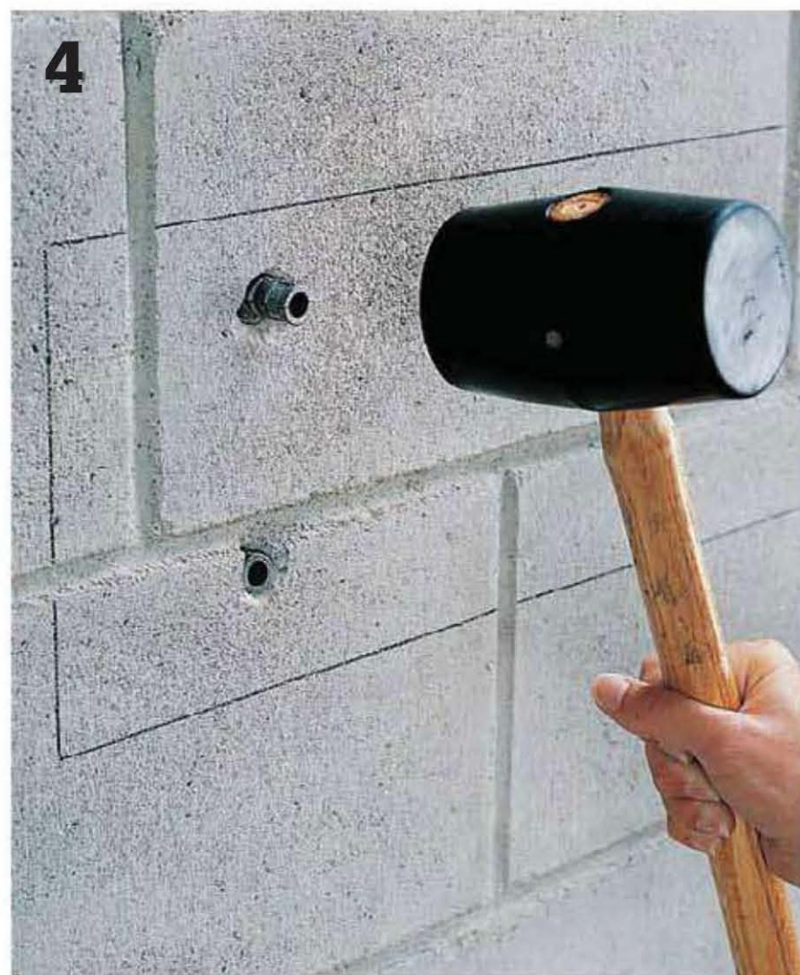
Drive lead masonry anchors for \frac{3}{8} " lag screws into drilled holes, using a rubber mallet.
