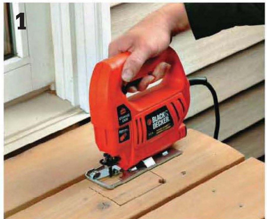
Mark the fixture location , then cut the holes using a jigsaw.
