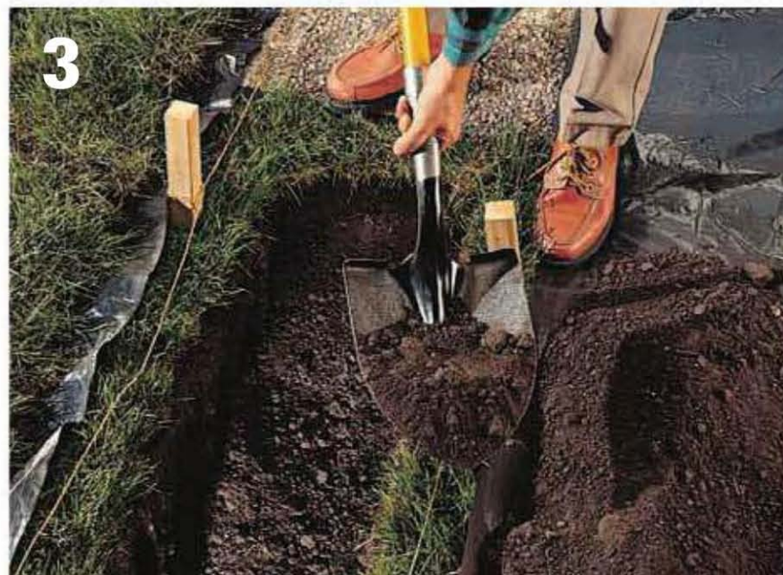
Outline trench locations with stakes and string, then dig the trenches to the depths required by your local code.
