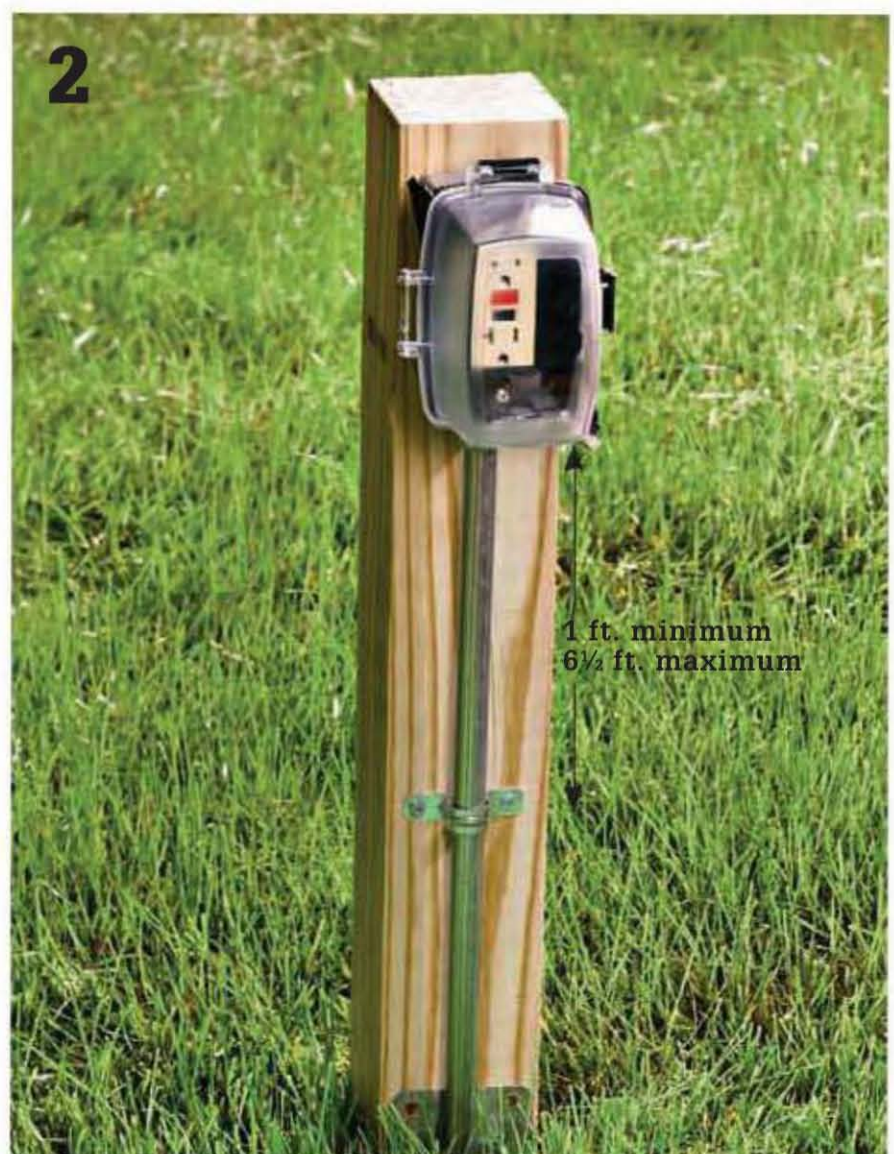
Install GFCI receptacles in weatherproof electrical boxes at least 1 ft.—and no more than 6½ ft.—above ground level.
