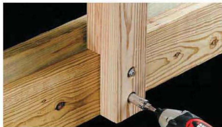
Attach the railing posts to the upper deck rim joists with carriage bolts, washers, and nuts.
