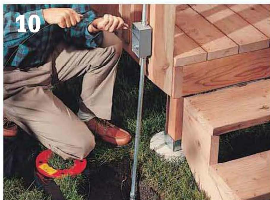
At the deck, use the fish tape to pull cable through the conduit and into the receptacle box and switch box.
