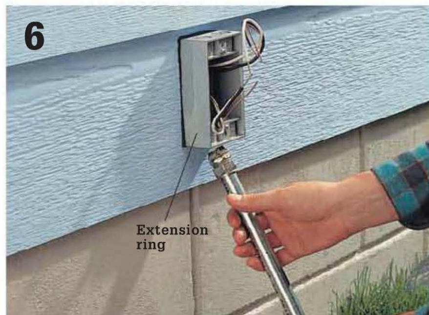
At the house, install conduit so it extends from the bottom of the extension ring to 4" from the bottom of the trench.
