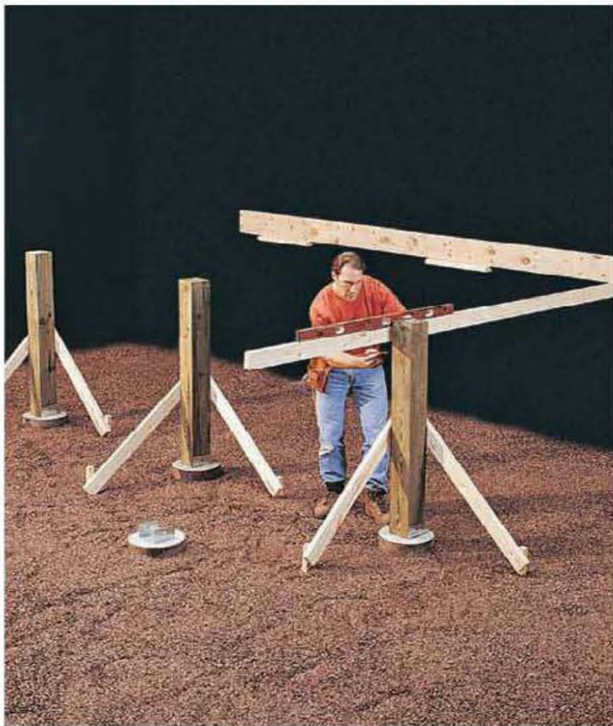
Determine the finished post height by leveling a straight 2 x 4 from the bottom edge of the ledger.
