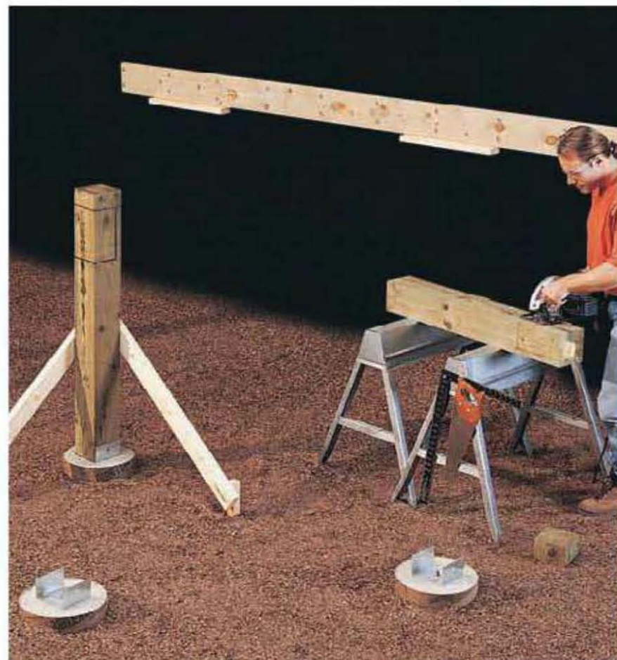
After marking the notches for the primary beam, cut out the tops of the posts with a circular saw and a handsaw.
