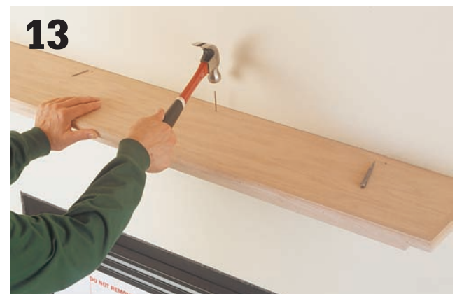
Fit the mantle over the cleat , and secure it with finish nails driven through pilot holes.
