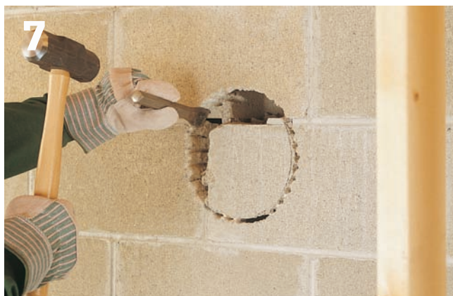
Break out the vent hole with a masonry chisel and hand maul, then carefully smooth the rough edges.
