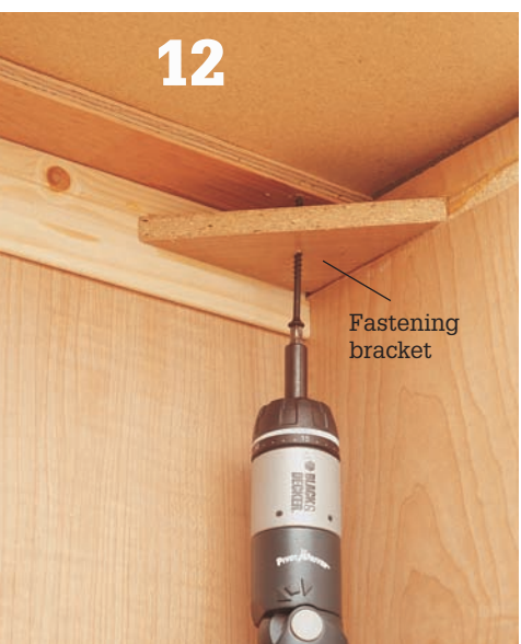
12 Secure the countertop through the cabinet brackets.
