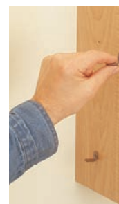
Drill holes to accept the posts of the shelf brackets, then push the brackets into place.
