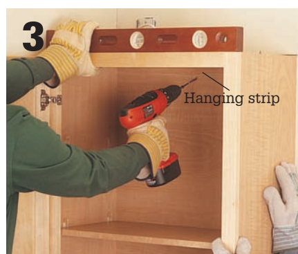
Set each wall cabinet against the back and side walls, and attach it with screws.
