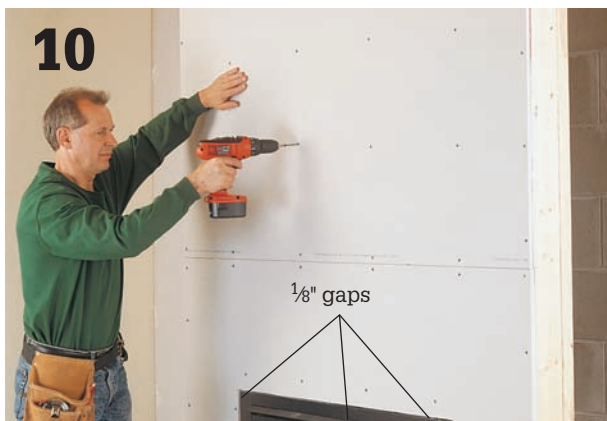
Cover the frame with wallboard , leaving a gap around the black front face of the unit.
