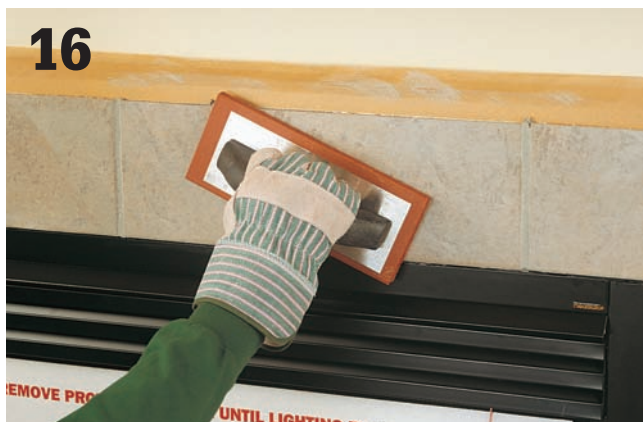
16 Force grout into the joints with a grout float, then make two passes to remove excess.
