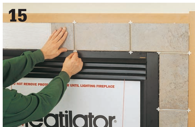
15 Apply adhesive inside the layout lines, then press the tile firmly into the adhesive.
