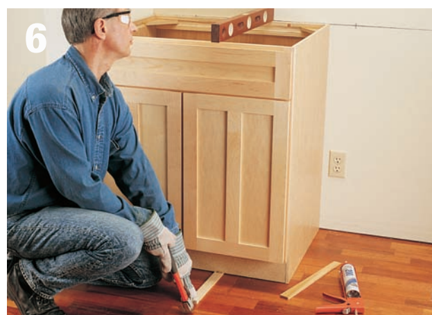
Shim under the sink base cabinet so that it is perfectly plumb and is aligned with the layout line.
