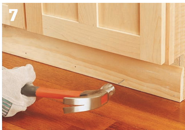
Trim the shims , and install the toe-kick molding with finish nails driven through pilot holes.
