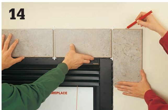
14 Dry-fit the tile around the fireplace front, and mark the wall to indicate tile positions.
