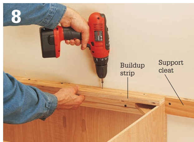
Install a plywood support cleat and buildup strips to provide support for the countertop.
