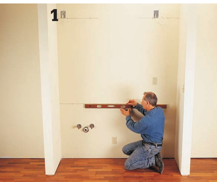
Measure up from the floor's high point , and draw level lines for the tops of both sets of cabinets.
