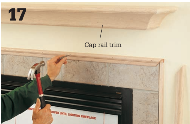
17 Attach the trim pieces around the tile with finish nails, and set the nails with a nail set.
