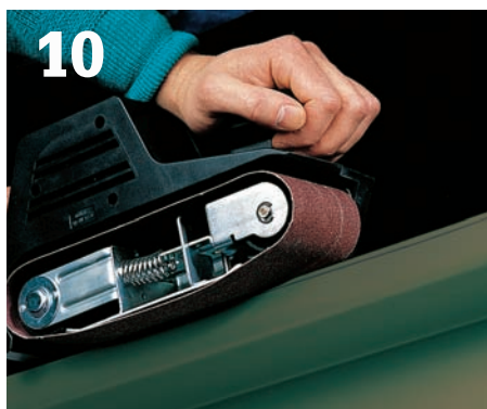
10 Sand the backsplash so it fits tight to the back wall.
