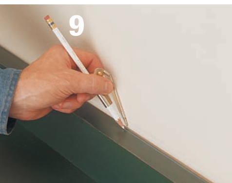
9 Set the countertop. If necessary, scribe the backsplash with a compass.
