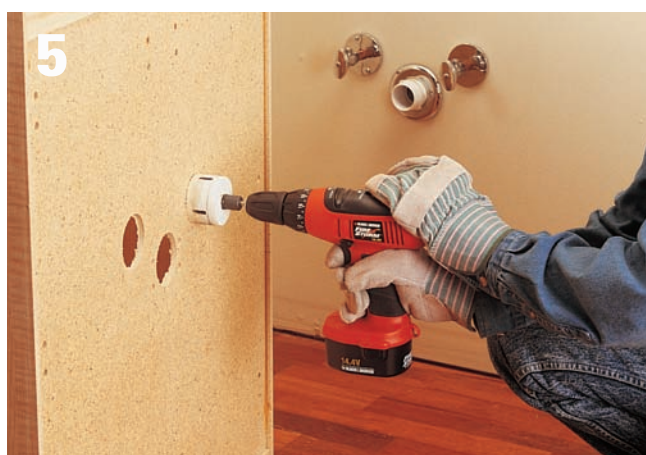
Cut holes through the back panel of the sink base cabinet for plumbing lines, using a hole saw.
