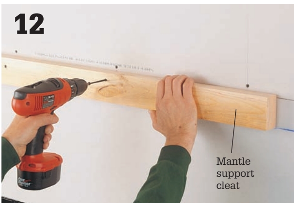
Draw a level line for the mantle support cleat, then attach the cleat to the studs with screws.
