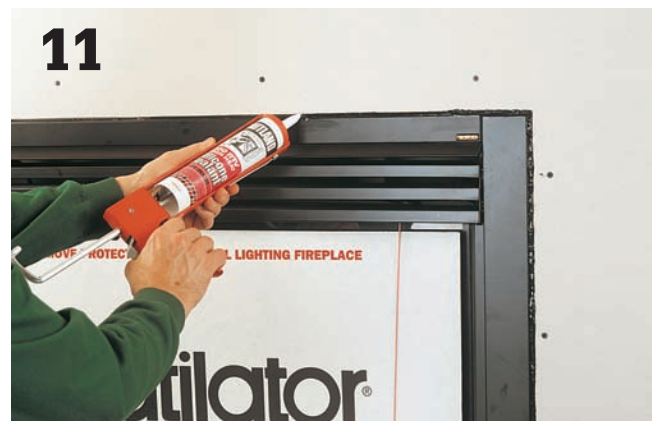
Seal around the unit's front face with high-temperature sealant.
