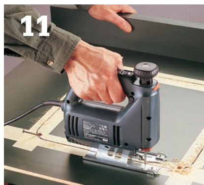
11 Draw the sink cutout onto the countertop, then make the cut with a jigsaw.
