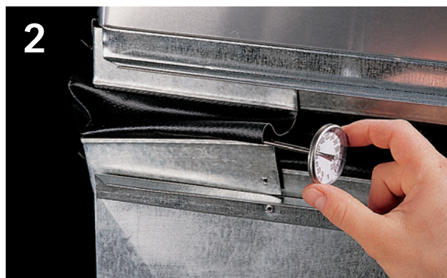
Check the temperature inside the supply duct and compare it with the temperature in the return duct.
