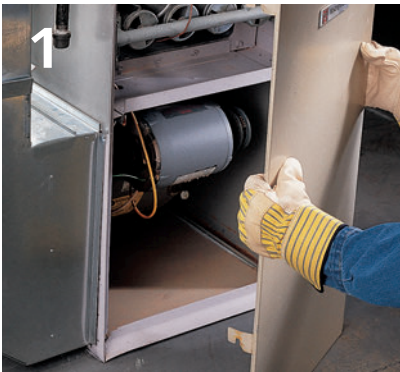
Remove the access panel to the blower housing and inspect the motor.
