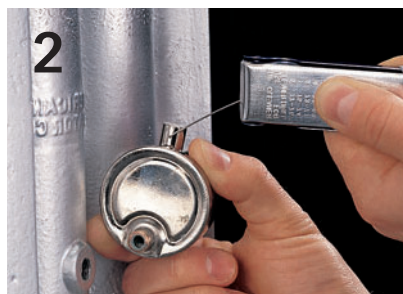
2 If the radiator isn't heating, clear the orifice with a fine wire or needle.
