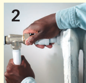
2 Fasten the valve to the supply tube, then secure the connecting nut on the tailpiece to the valve.
