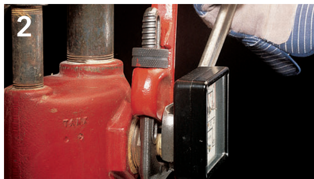
If the valve or gauge on top of the boiler is attached to a separate fitting, hold the fitting still with one wrench while removing the valve or gauge with another.
