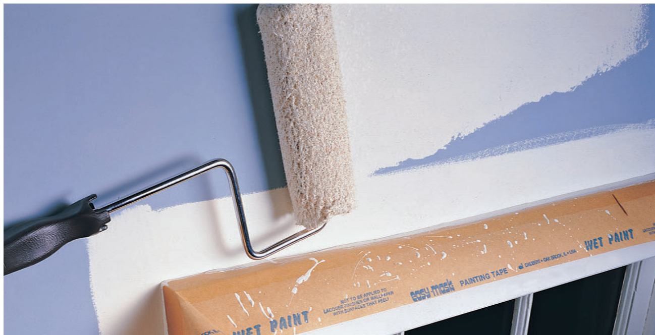
Cut in around doors and window casing with a paintbrush and then finish painting the wall with a roller.
