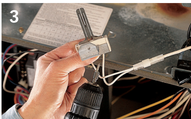
Disconnect the faulty hot-surface igniter from the mounting bracket.
