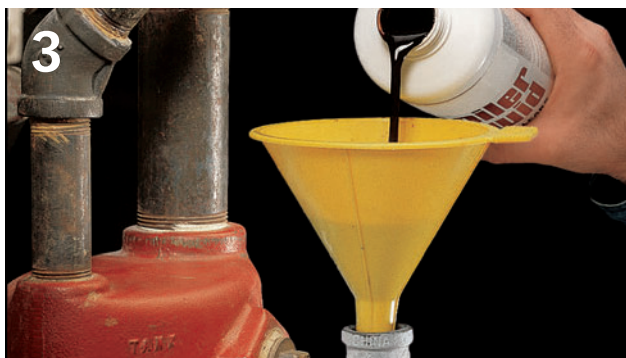
Using a funnel , add a recommended rust inhibitor to the boiler through the valve or gauge fitting.
