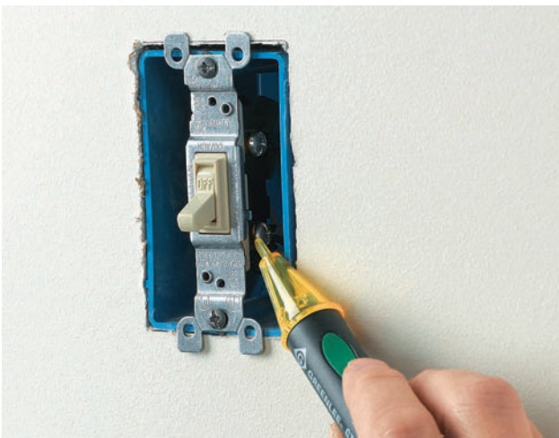
Confirm power is OFF by testing at the outlet, switch, or fixture with a voltage tester.
