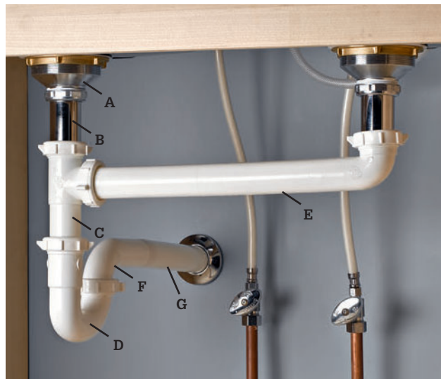
Kitchen sink drains include a strainer body (A), tailpiece (B), waste T (C), P-trap (D), outlet drain line (E), trap arm (F), and wall stubout with coupling (G).
