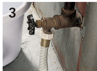
3 A convector-based heating system is usually bled at the boiler by holding a hose underwater and flushing the system until there are no more air bubbles coming from the hose.
