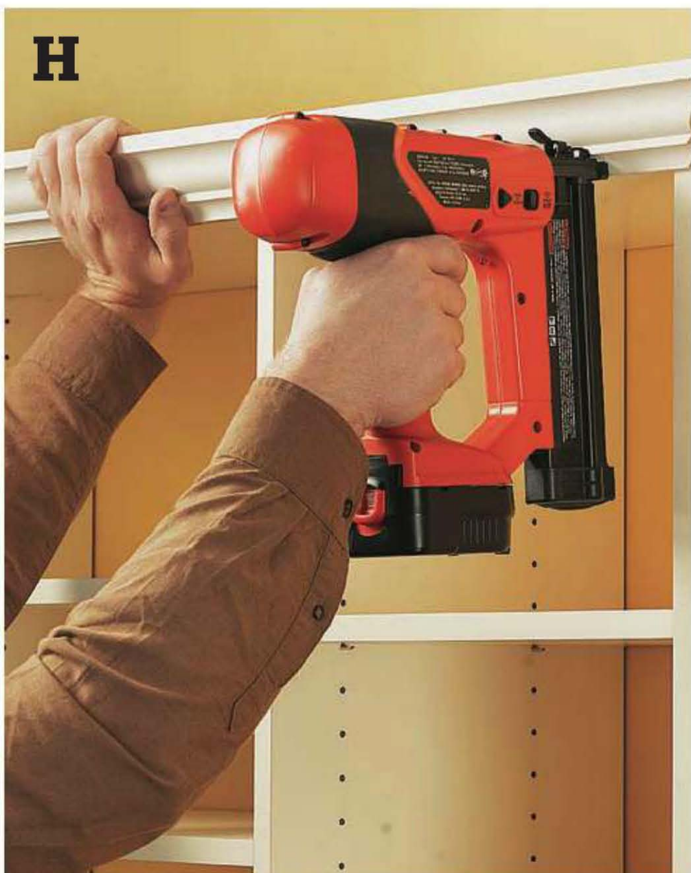
Using a pneumatic nailer , fasten crown molding in place along top front edges of closet unit.
