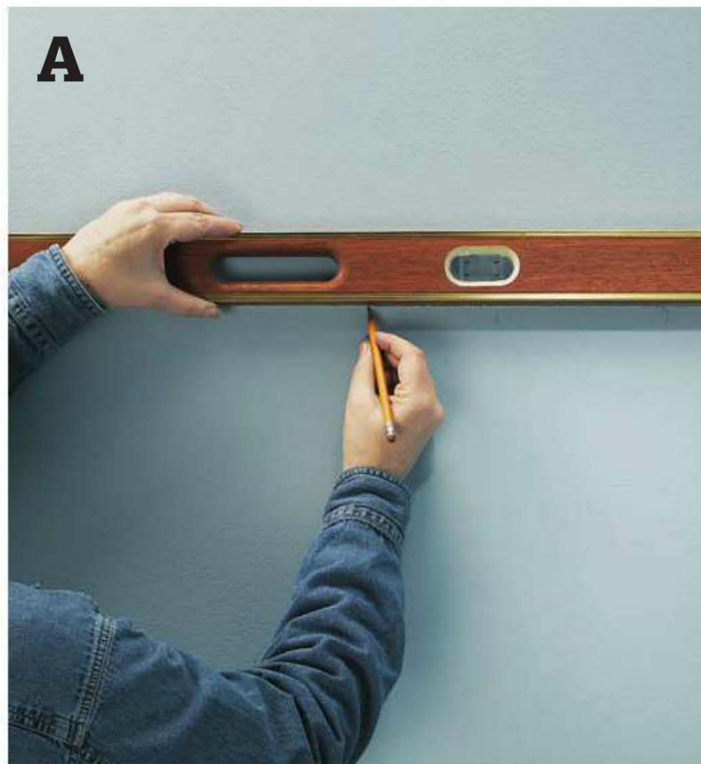
Measure your closet, and draw a level line 48" up from ground.
