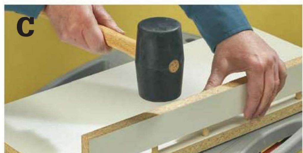
Tap the cleat and shelf together with a rubber mallet, and allow to dry.
