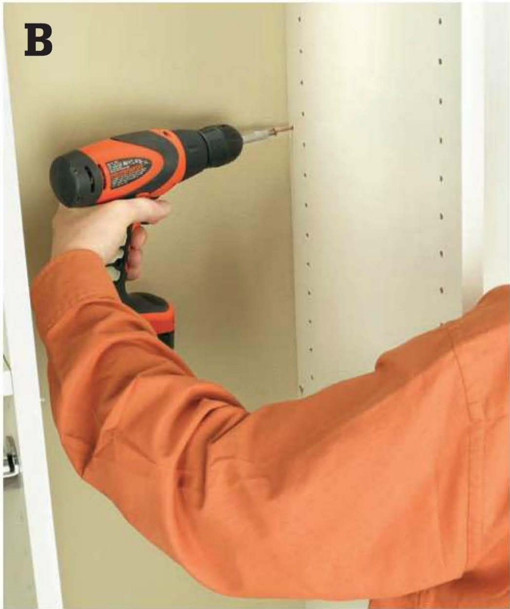
Fasten the two verticals together with 1½" screws. Work from the interior of the existing unit and drill the screw into the end of the wall vertical.
