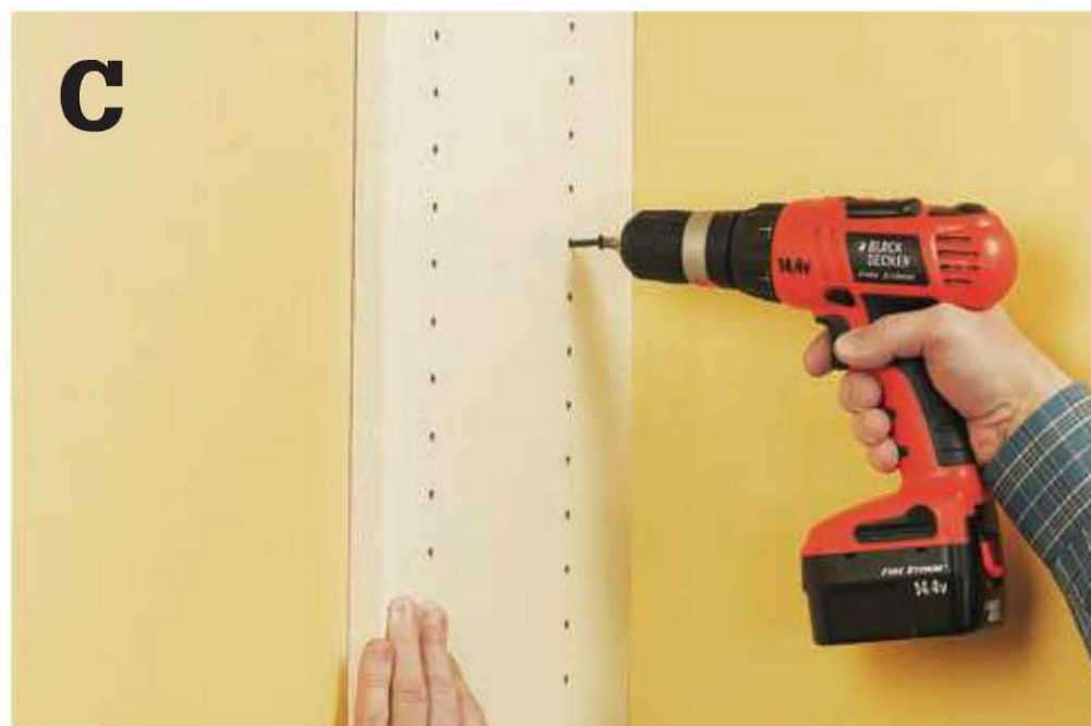
Align the first vertical against the wall and temporarily screw it to the wall.
