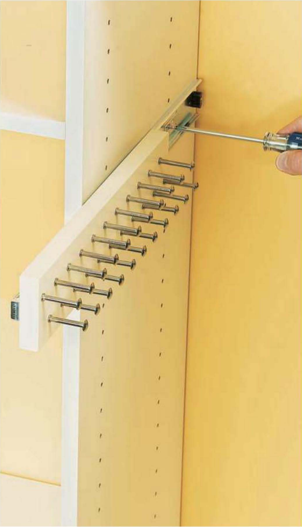
This manufacturer tie rack fastens directly into predrilled shelf-pin holes. Such versions are widely available and easy to install.
