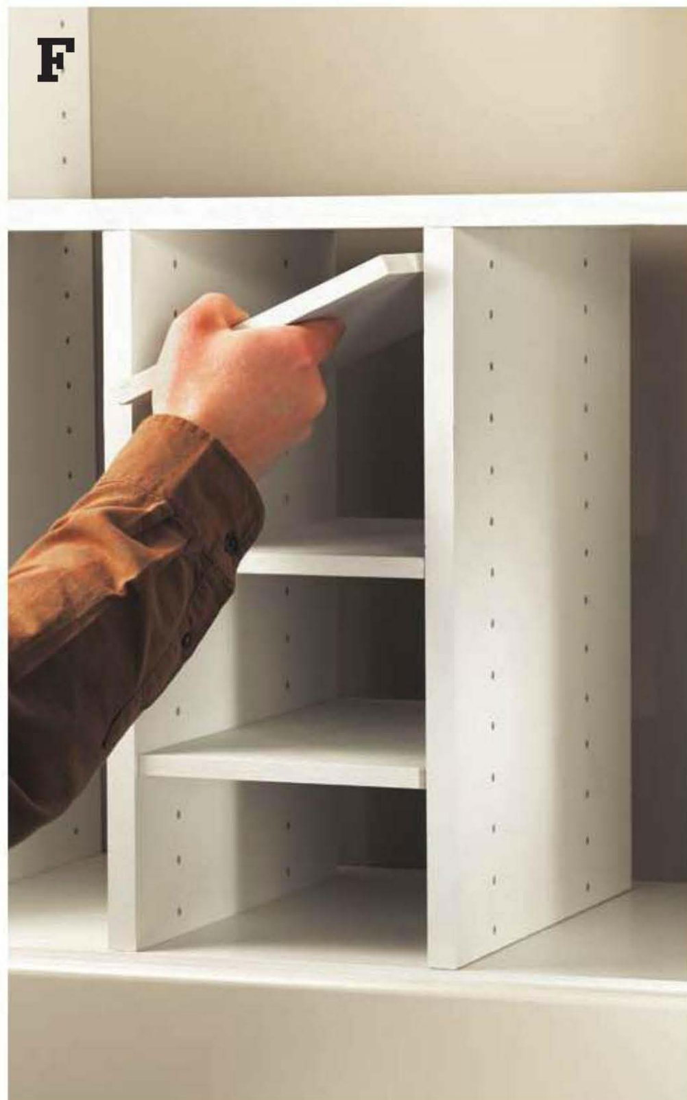
It is easiest to install adjustable shelving by first tilting it at a 45^\circ angle, sliding it into place, and then lowering it down level onto the shelf pegs. Tap into place, if necessary.
