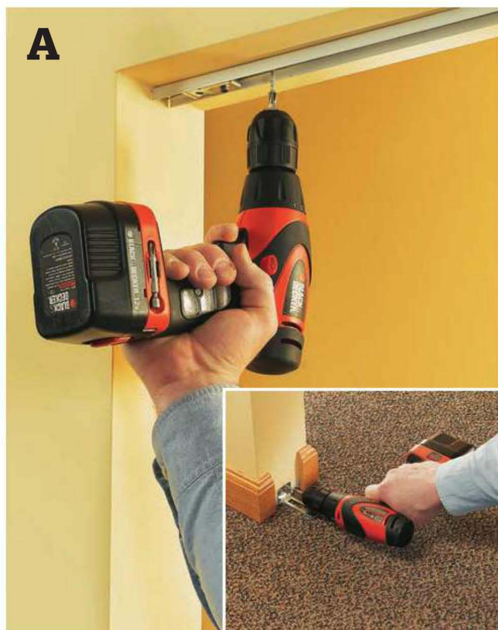
Fasten the track to the header with panhead screws. Fasten brackets to the side jambs with flathead screws.
