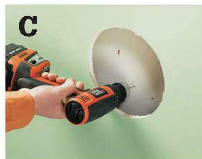
Drill placement holes using a \frac{1}{32} " drill bit.
