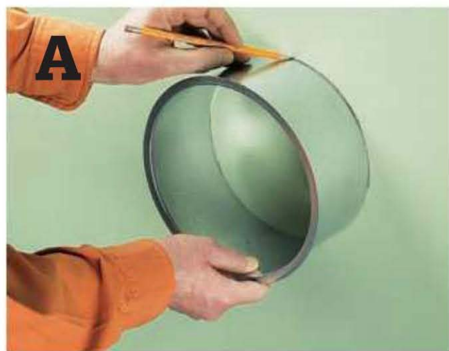
Mark the wall where there are no studs, and then hold the vent up to the wall and trace around it for a cut line.
