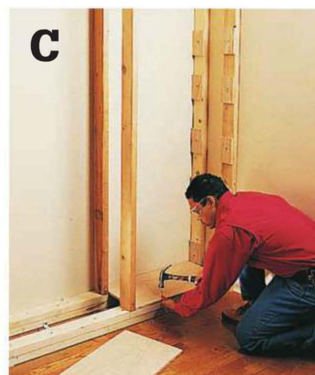
Attach the plywood top and bottom panels to the top and sole plates using 1½" finish nails.
