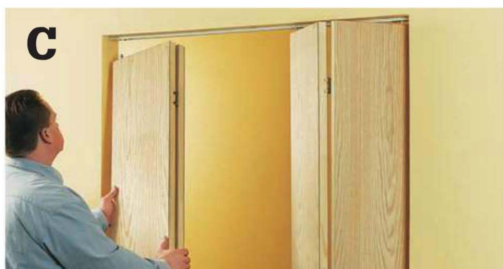
Lift doors into position , inserting the pivot and guide posts into the head track.
