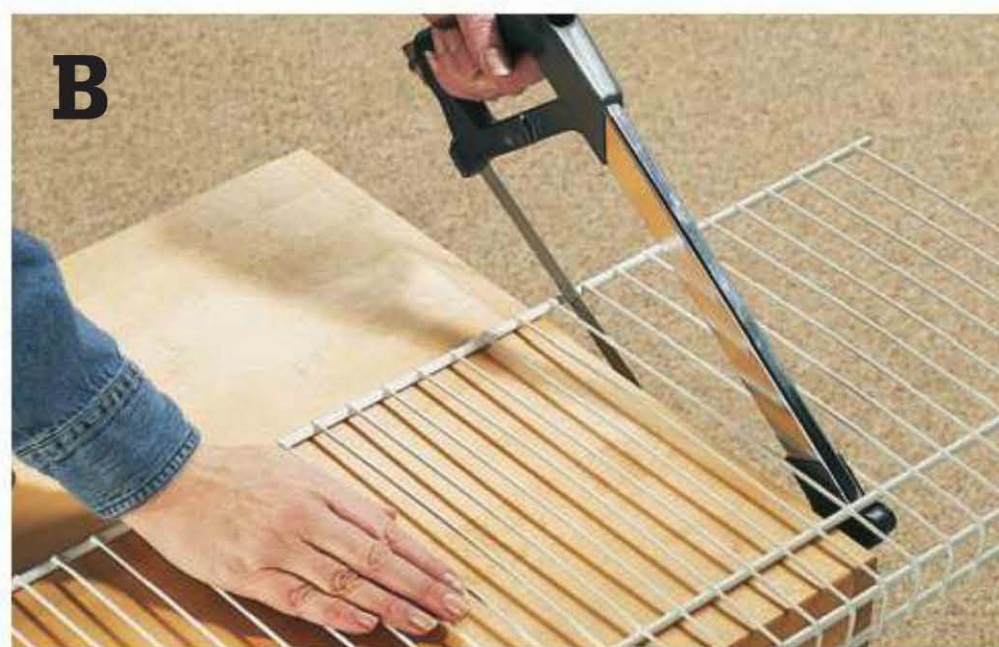
Measure and mark cut length of shelving onto the wire. Cut wire shelving to length, using a hacksaw.
