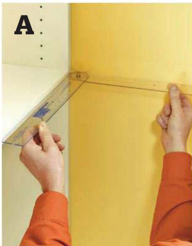
Measure the space in between the back and side units, using an angle finder for wall sides that are not square.
