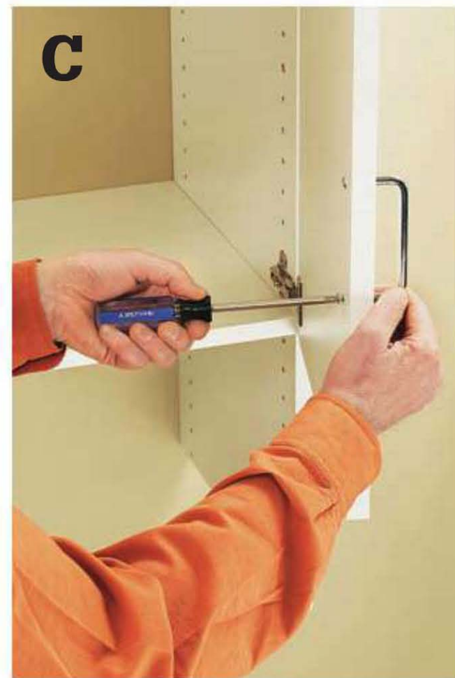
Attach door handles or knobs, and any door catch hardware.
