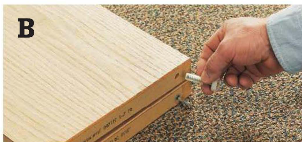
Insert pivot posts into predrilled holes at the bottoms and tops of doors. Insert guide posts at the tops of the leading doors.
