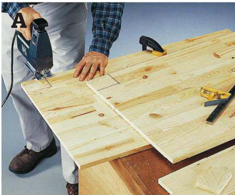
Cut the toe-kick notches into the ends and divider using a jigsaw.
