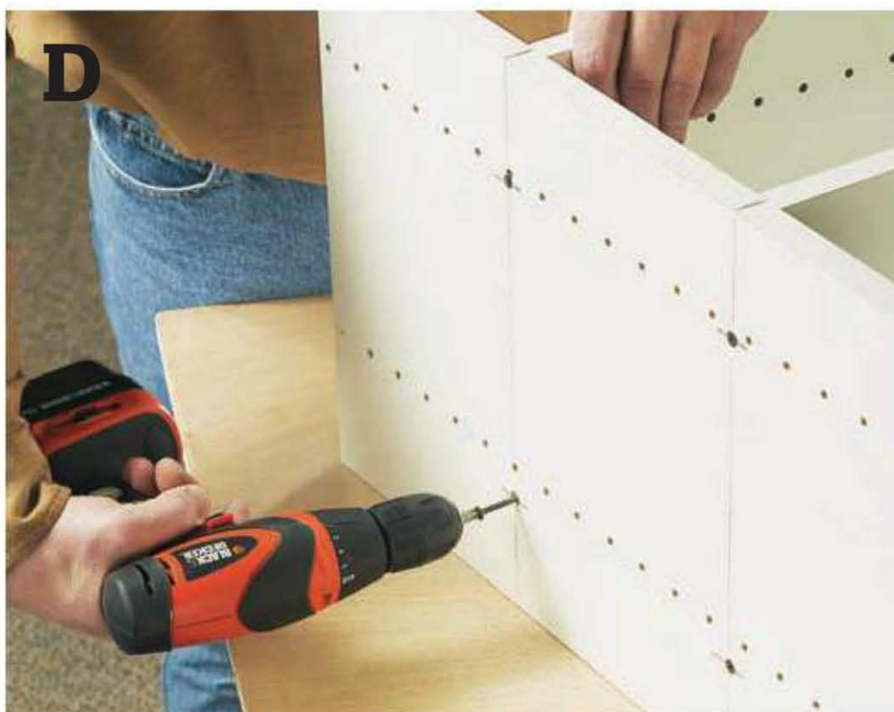
Countersink screws through the fixed shelf into pars.
