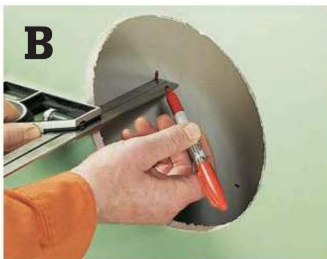
Trace the cut line to the interior of the other side of the wall.
