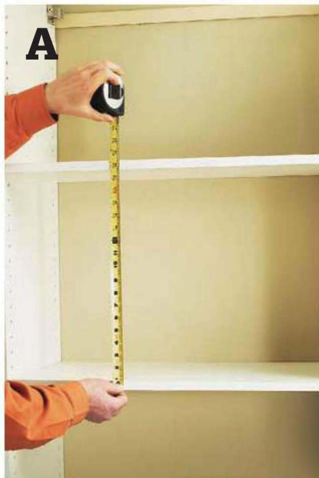
Measure the width and height of the door opening from the outer edge of verticals and fixed shelves.
