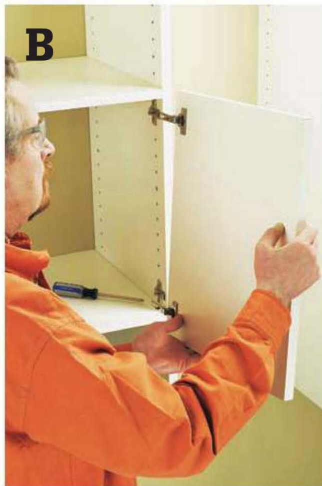
Attach hinges to the verticals and door. Then attach door according to manufacturer instructions.
