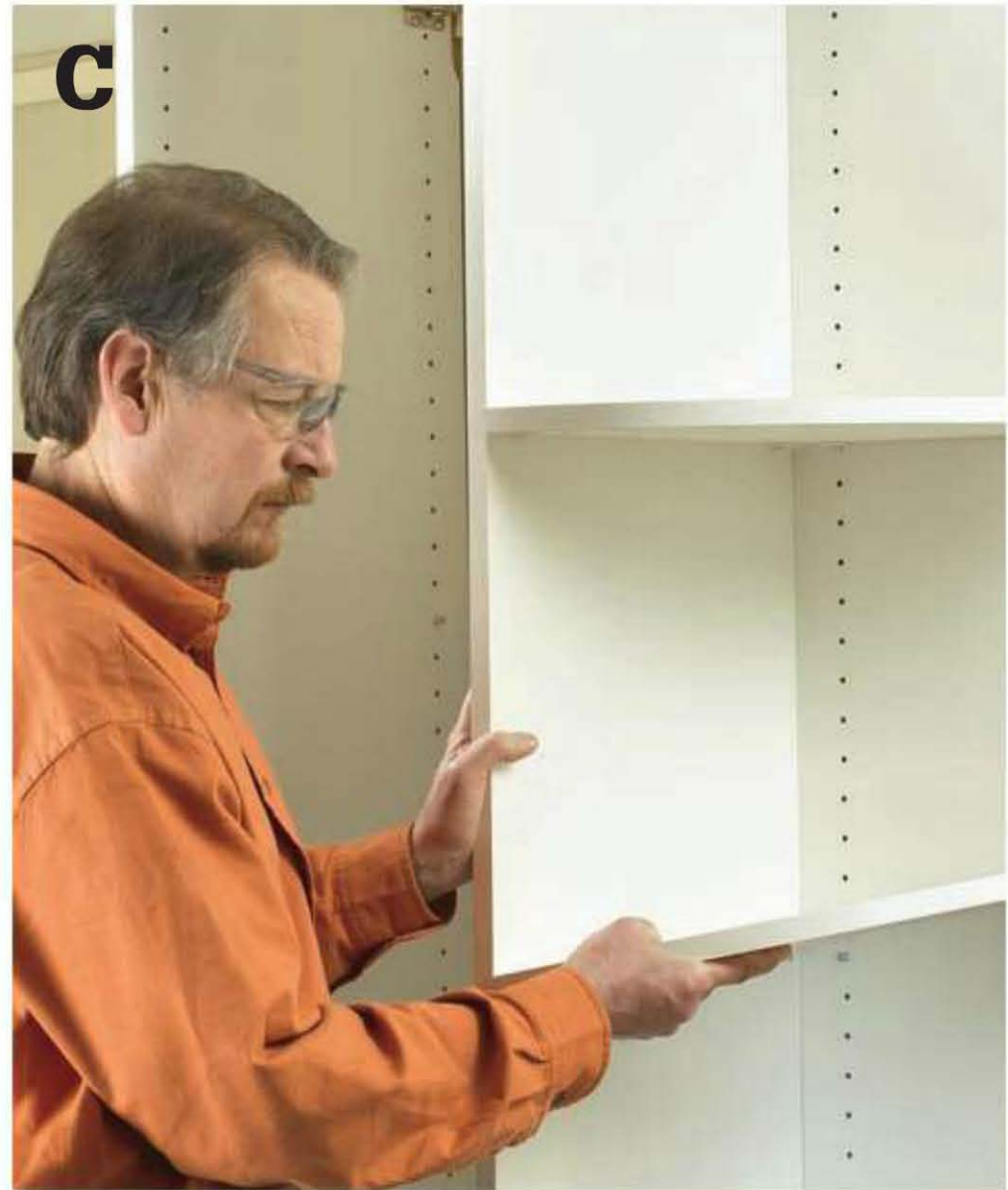
Install adjustable shelves on shelf pins. Fixed shelves (at top, middle, and bottom) are fastened to the existing unit with KD screw/dowels (KD screws on the new corner vertical).
