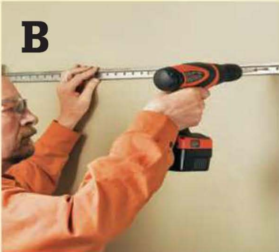
Align the bottom of the wall rail with the level line on wall, and fasten to wall with a few screws.
