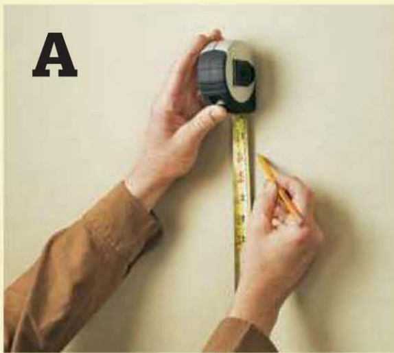
Measure up to 81" and mark a level line on the wall.
