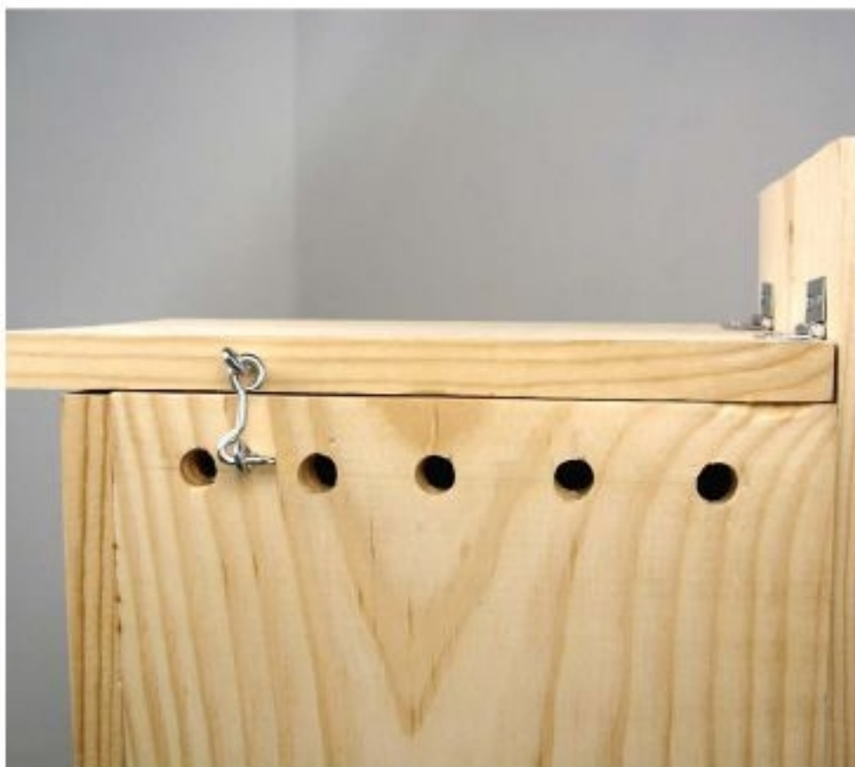
Install the screen-door hook. Place a screen-door hook on one or both sides to hold the top securely closed. Adjust the hook so it is tight enough that predators such as raccoons can't open it and eat the eggs or the nestlings.
