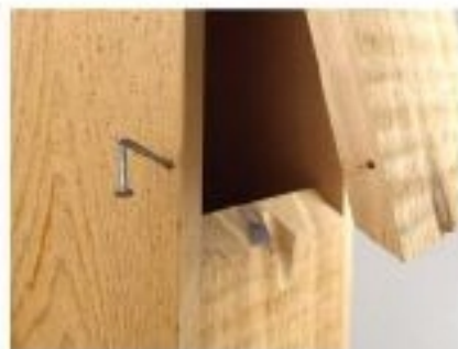
Keep your ducks safe by using a bent nail to keep the side door closed.
