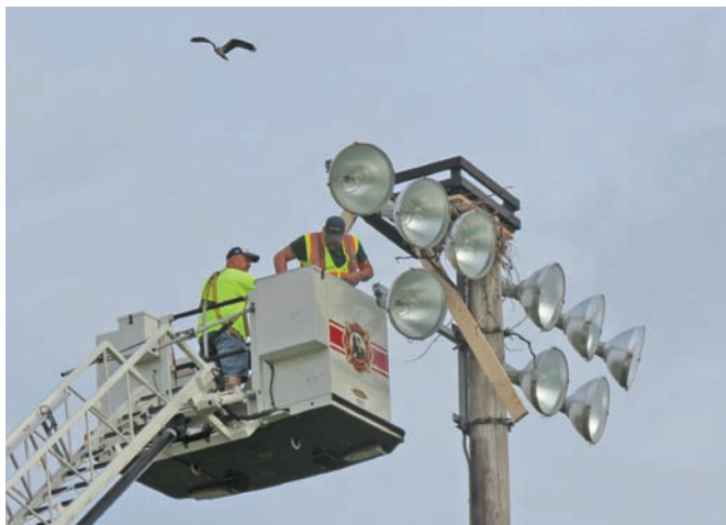
To help out the Ospreys and prevent a potential fire, the Stoughton, Wisconsin, fire department installed a new nesting platform for the Ospreys, a safe distance away from the hot lights. Patrick Ready
