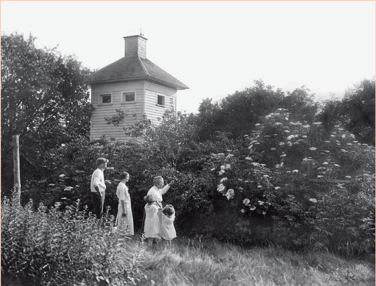
Althea Sherman (third from left) teaches neighbors about Chimney Swifts. Her Chimney Swift tower, pictured in the background, was made from pine, white oak, and native cottonwood. This twenty-eight-foot-tall, nine-foot-square wooden tower enclosed a two-foot-square artificial chimney, which protruded through the roof. © Althea R. Sherman Collection, the Althea R. Sherman Project
