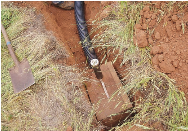
This artificial burrow, installed by birder and photographer Steve Simmons, uses a strong plywood box with a handled lid for easy access. It is placed two feet underground and attached to an eight-foot-long corrugated plastic pipe, which is connected to a smaller box at the entry. Backhoes are first used to dig out the soil. Steve Simmons
