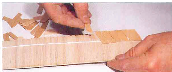
Fig. 5.11-8: Placing the first row of shingles on a bead of glue with their bottom edges extending slightly over the lower edge of the plywood base.
