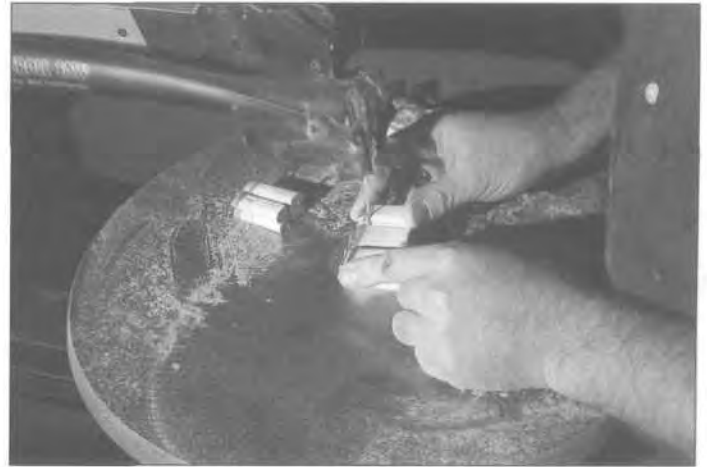
Cutting the windows in the second terrace. In an attempt to make the cut as inconspicuous as possible, the saw is introduced in the crevice between the towers.
