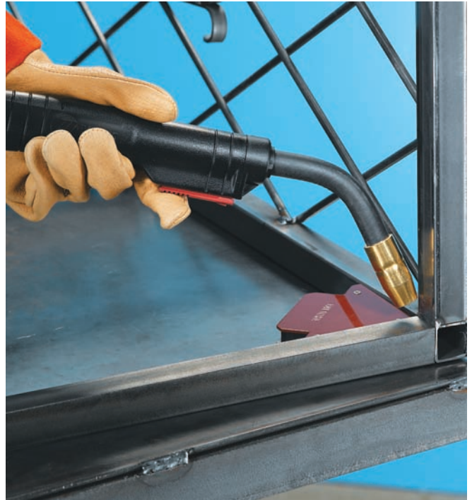
Tack-weld the front supports in place and check for square.
