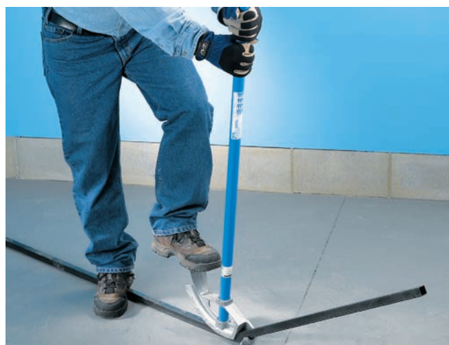
Create the window and door arches by bending the tubing with a large conduit bender.
