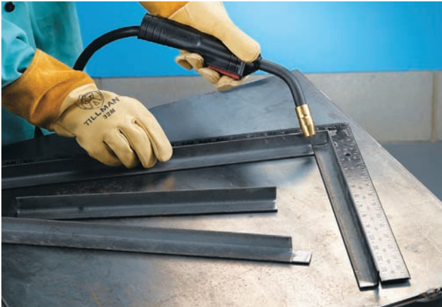
Using a carpenter's square, lay out the table sides. Tack-weld together and check for square before final welding.
