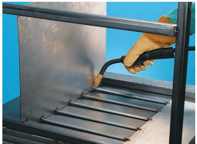
Weld the decorative bars to the table sides and shelf every 3". Weld from the inside.
