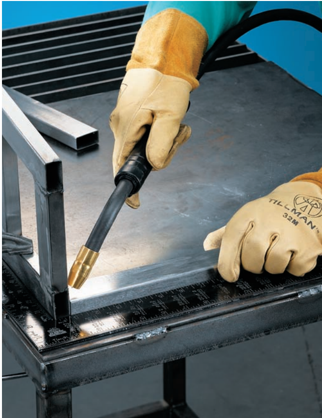
After assembling the sides, weld the backs in place. Check for square both vertically and horizontally.
