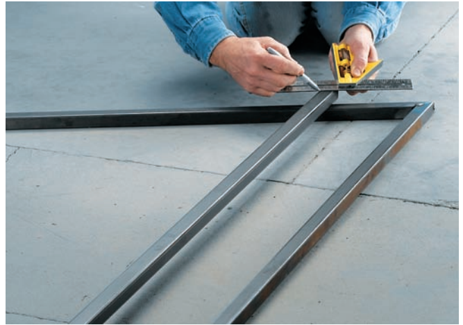
Mark the roof crossbar for cutting.
