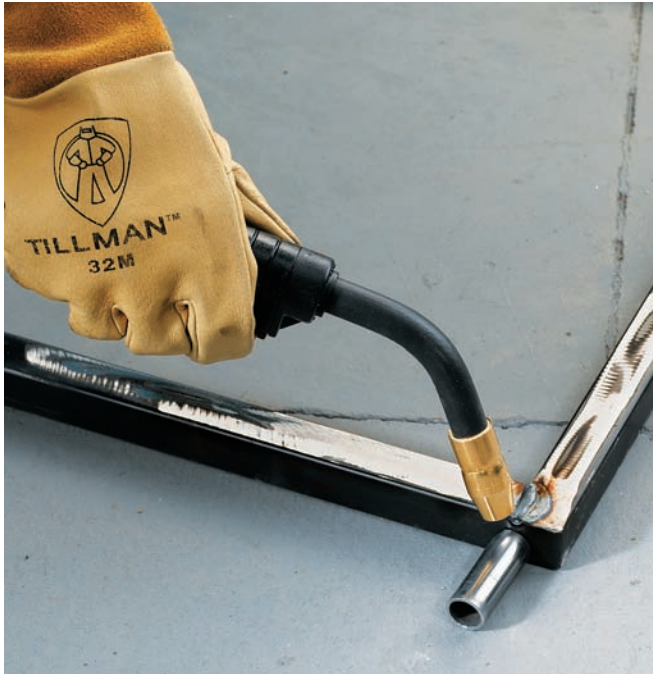
Weld the roof sleeves to the tops of the side panels.
