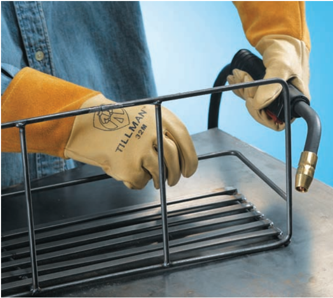
Weld the top shelf frame to the frame 2" above the shelf.
