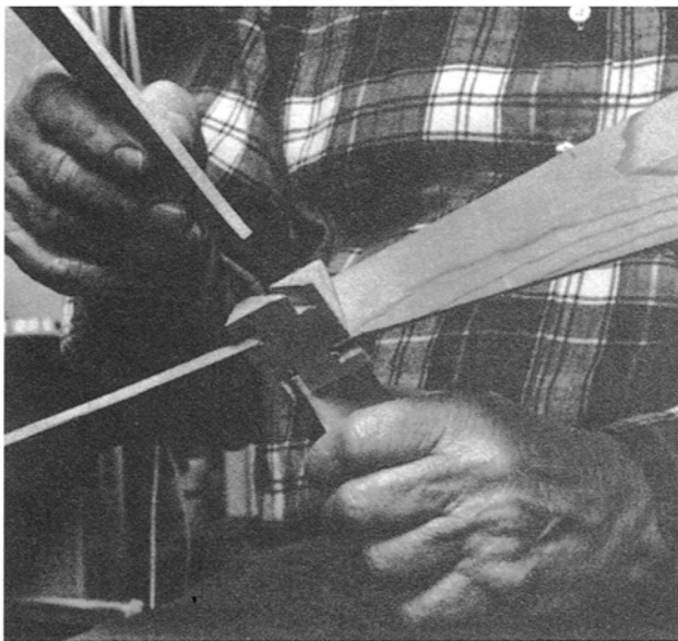
Figure 2-12. Fit the blades snugly into the slots.
